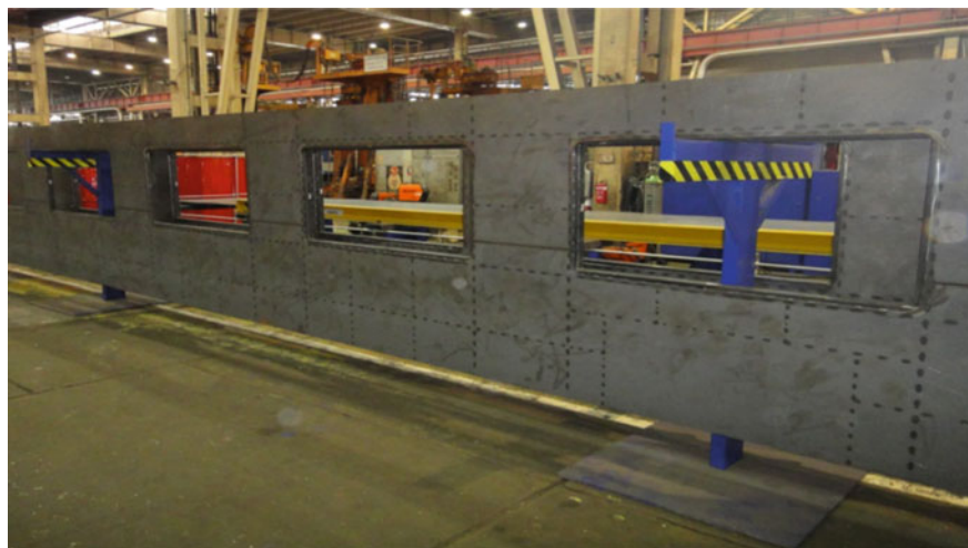
Fig. 4 Welded side wall elements (Photo: István Borhy)
