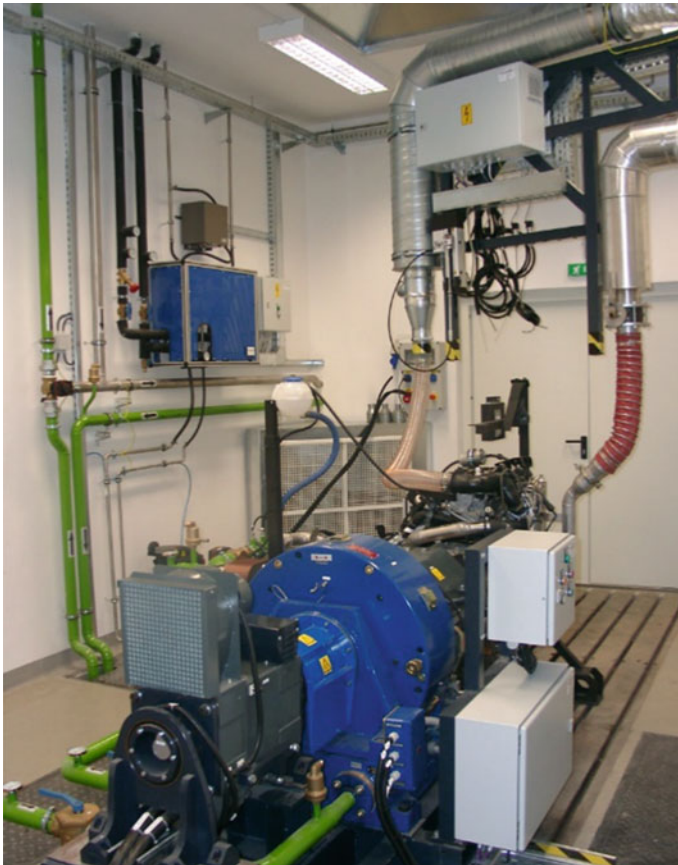
Fig. 9 Interior of the engine test laboratory
