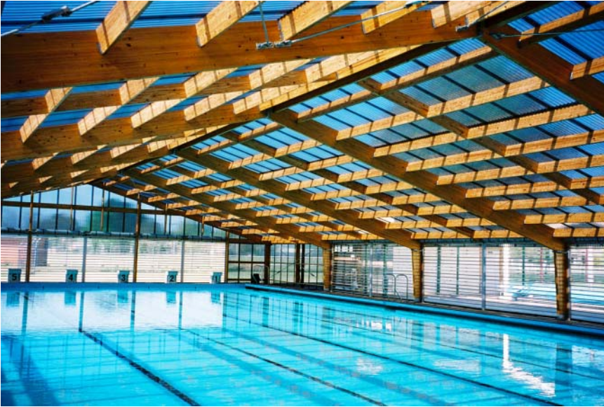
8.2 Swimming pool enclosure, Guyra, Australia. Courtesy of Hyne, Australia.
