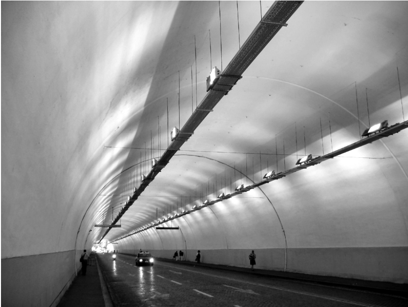
11.4 Tunnel: photocatalytic coating and dedicated UV lighting system (Rome, Italy). Courtesy of G. L. Guerrini, CTG Italcementi Group.
