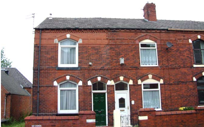
4.9 Example of replacement brickwork.
