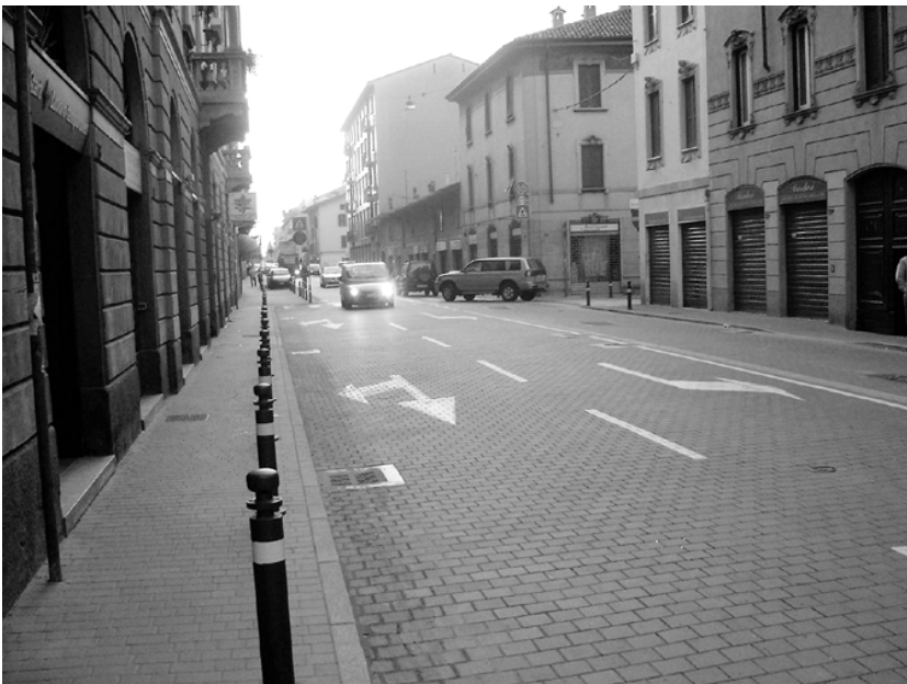
11.5 Photocatalytic road made from paving blocks (Italy). Courtesy of G. L. Guerrini, CTG Italcementi Group.
