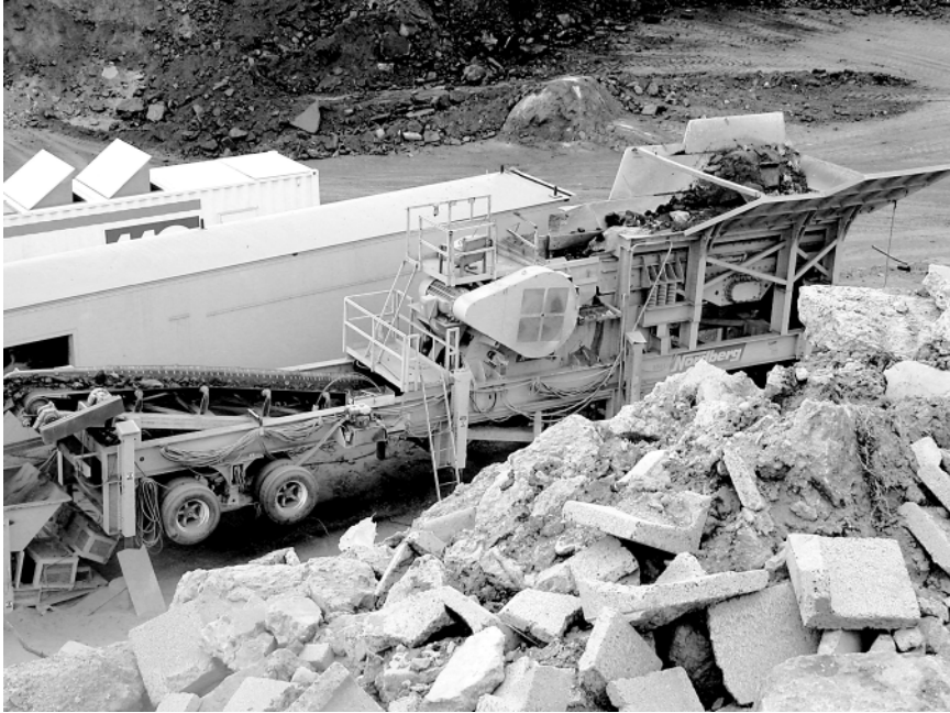
1.6 Recycling concrete using a portable crusher. Photo courtesy of Metso Materials, Tampere, Finland.
