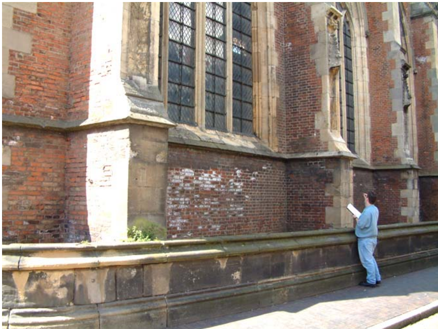
4.4 The north side of the chancel at Holy Trinity Church, Hull, UK.
