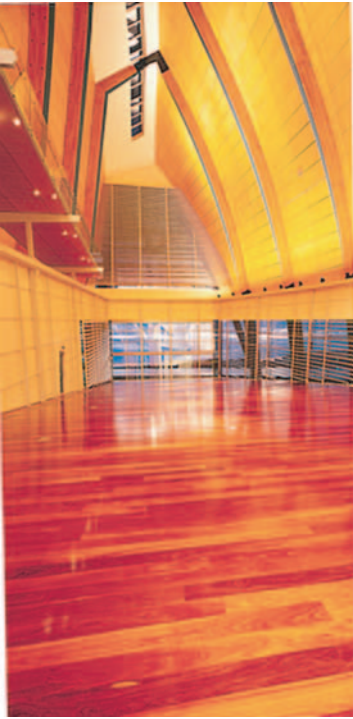
8.10 Western Australian Maritime Museum, Fremantle, Australia, showing the glulam three-pin arch exposed as an architectural feature (a) and during construction (b). Courtesy of the Australian Maritime Museum, Fremantle, Australia.
