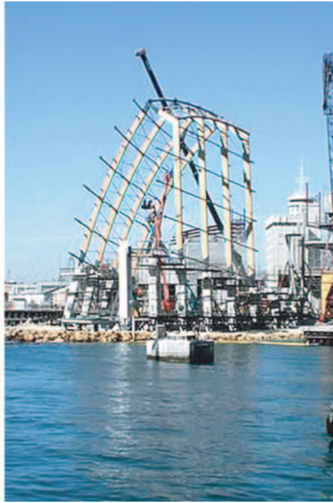
8.10 Western Australian Maritime Museum, Fremantle, Australia, showing the glulam three-pin arch exposed as an architectural feature (a) and during construction (b). Courtesy of the Australian Maritime Museum, Fremantle, Australia.
