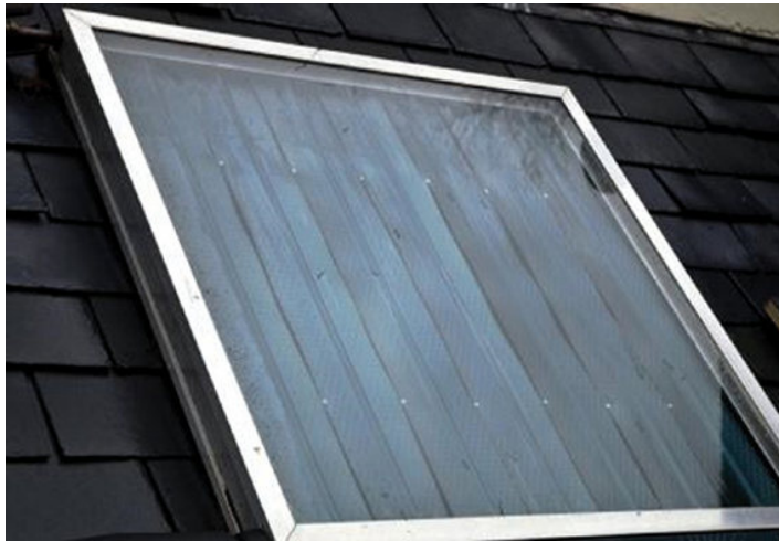
Figure 3.14 Flat plate collectors solar thermal system (Photo by Steve Goodhew).
