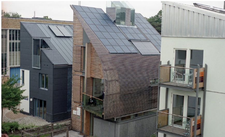
Figure 3.5 Homes at the UK BRE innovation park (Photo by Steve Goodhew).
