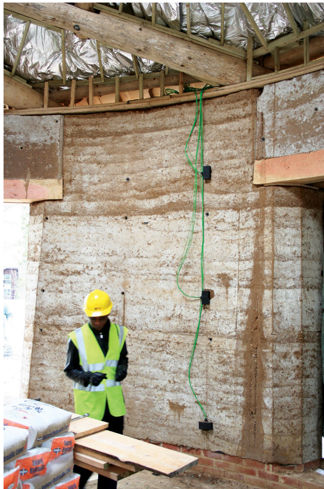
Figure 5.3 Rammed earth wall as part of a complex of buildings in Lincolnshire UK (Photo by Steve Goodhew).
