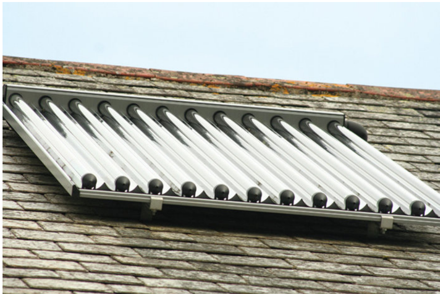
Figure 3.15 Evacuated tube collector solar thermal system (Photo by Steve Goodhew).
