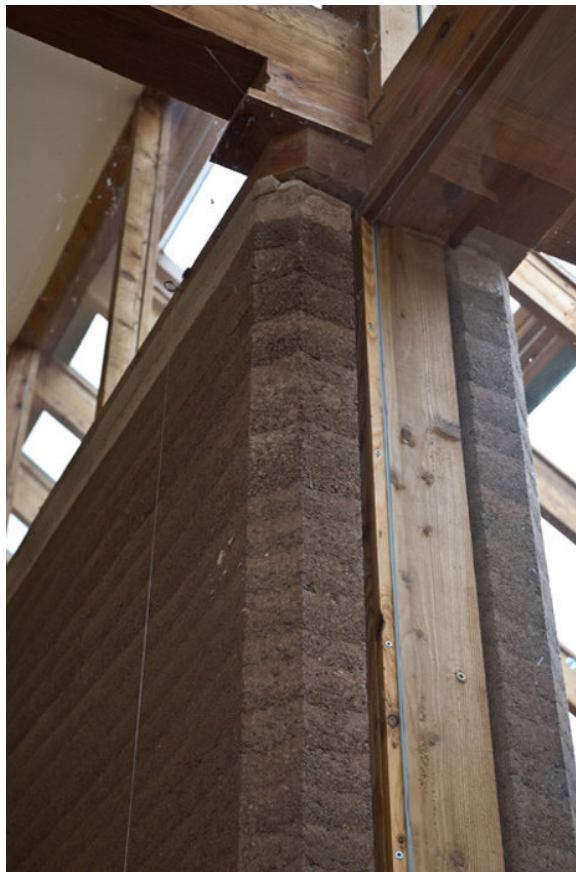
Figure 4.5 Rammed earth walls at the Centre for Alternative Technology, Mid Wales, UK (Photo by Steve Goodhew).
