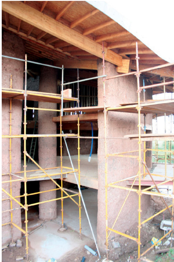
Figure 5.4 Series of cob walls built as part of a 3-storey large cob dwelling in Devon UK (Photo by Steve Goodhew).
