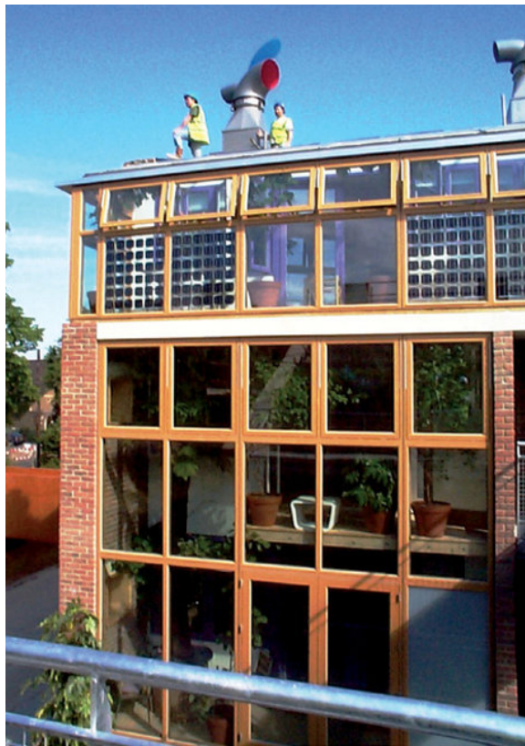
Figure 3.11 Chicken head ventilator at BedZED. Reproduced by permission of Brian Pilkington.
