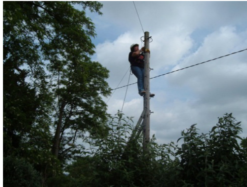
Engineer (OSP) climbing the telephone pole.
