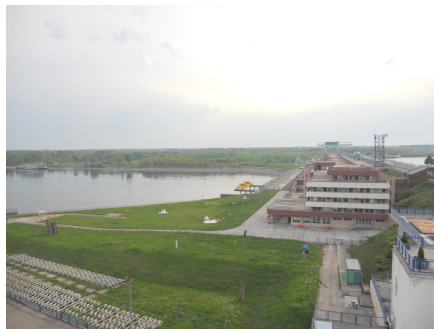
Hydroelectric power station at Gabčíkovo Dam, Slovakia.
