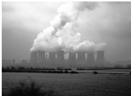
Cooling towers showing evaporating water at Ratcliffe-on-Soar Power Station, United Kingdom.
