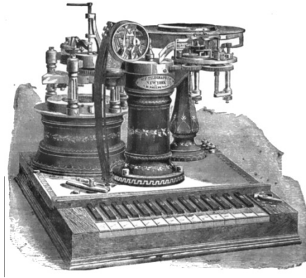
Phelps' Electro-motor Printing Telegraph from circa 1880, the last and most advanced telegraphy mechanism designed by George May Phelps
