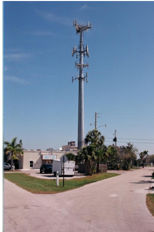
Wireless communication tower, cell site
