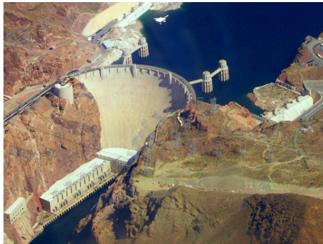
Large dams such as Hoover Dam can provide large amounts of hydroelectric power; it has 2.07 GW capability.
