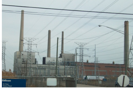
St. Clair Power Plant, a large coal-fired generating station in Michigan, United States.
