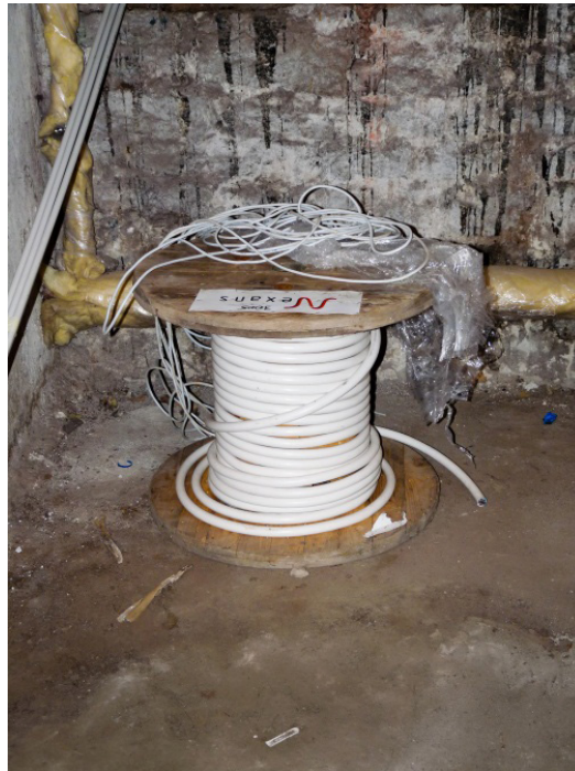
5 core PVC insulated copper cable
