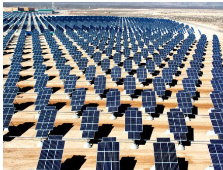
Nellis Solar Power Plant in Nevada, United States.
