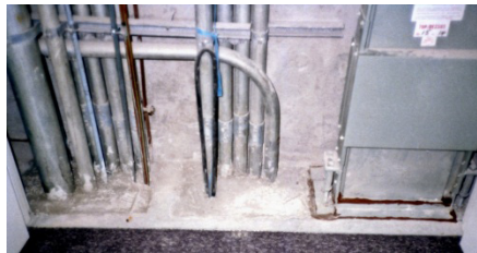
Topside of firestop with penetrants consisting of electrical conduit on the left and a bus duct on the right. The firestop consists of firestop mortar on top and rockwool on the bottom, for a 2-hour fire-resistance rating.
