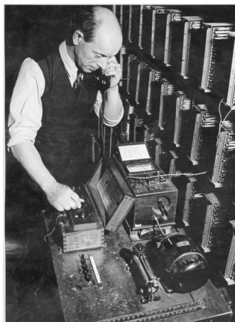
Telecommunications engineer working to maintain London's phone service during World War 2, January 1942 while all the power was off so he needed to find a power supply
