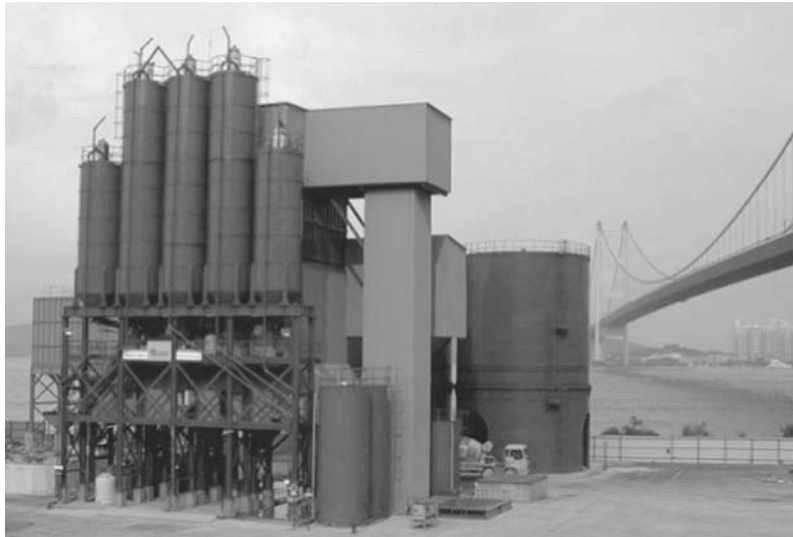
Figure 3-11 Ready-mix concrete plant
