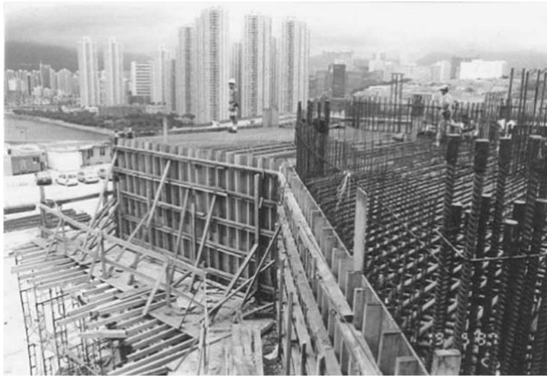
Figure 3-15 Framework for transfer block of a tall building (photo provided by Peter Allen)
