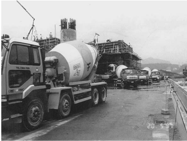
Figure 3-13 Delivery of concrete by truck
