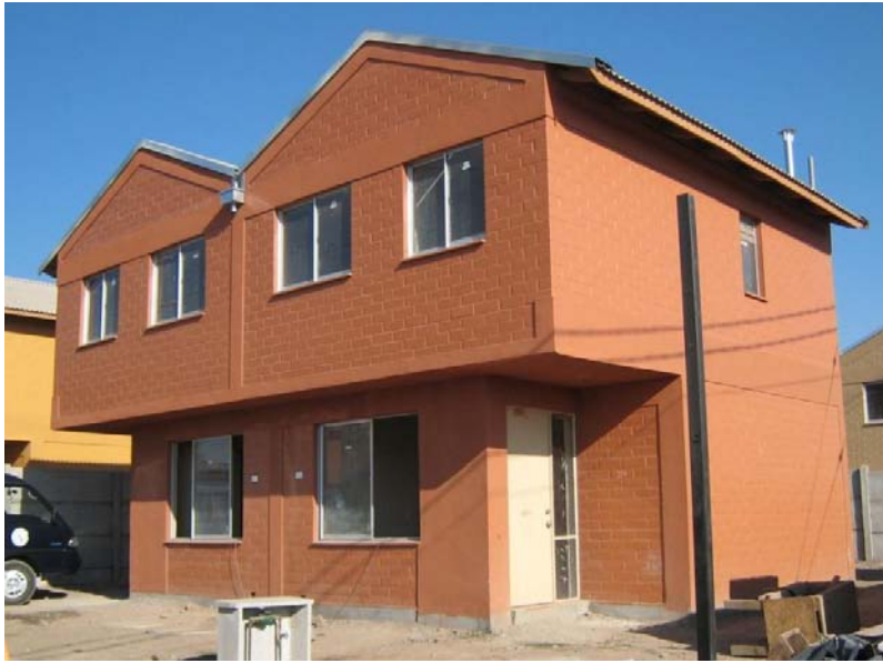
Figure 2. Front view of test structure.
