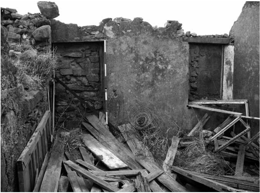
Figure 3.6 The remains of another blackhouse in Ness that has a complex history of adaptation and change
