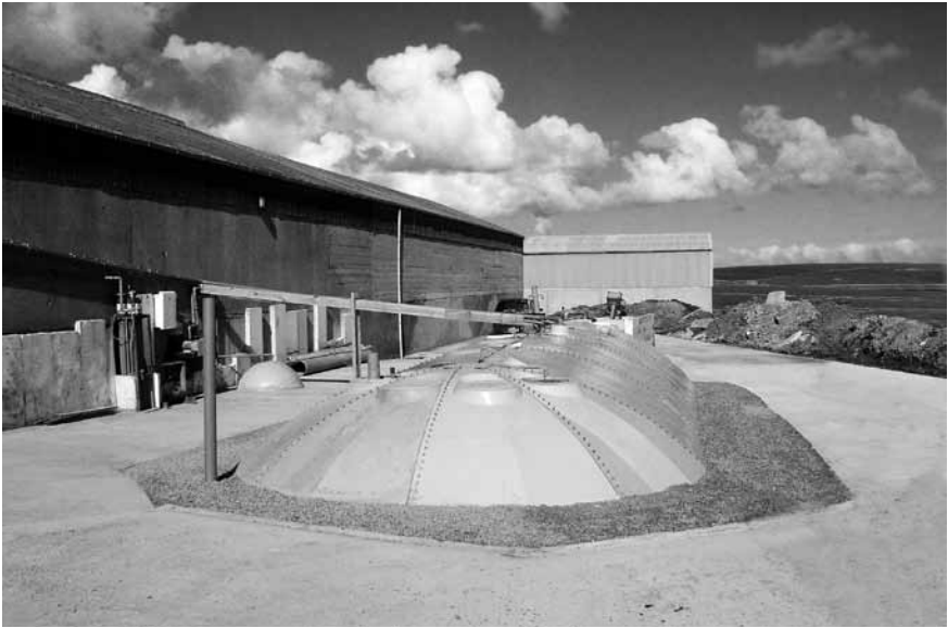
Figure 4.3 Anaerobic digester built by Heat & Power Limited, Westray, Orkney
