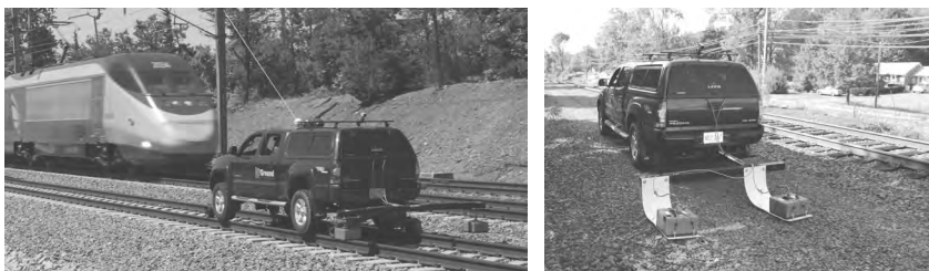
Figure 10.10 400 MHz GPR antenna installed on hi-rail vehicle (left photo), and GPR setup to investigate right-of-way access road for new track (right photo).
