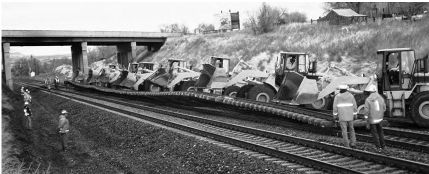
Figure 10.5 Removing track panels with front-end loaders.
