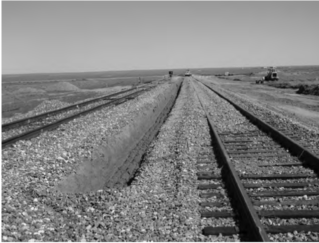
Figure 5.29 Trench prior to being filled with coarse gravel.
