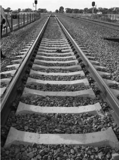
Figure 1.27 Half-frame sleeper track installed at bridge approach.
