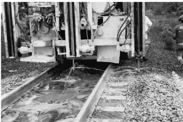
Figure 9.28 Slurry injection nozzle and rod system.
