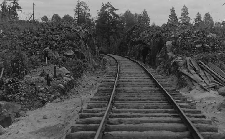
Figure 1.3 Early track structure with hand hewn railroad ties. (Courtesy of Library of Congress.)
