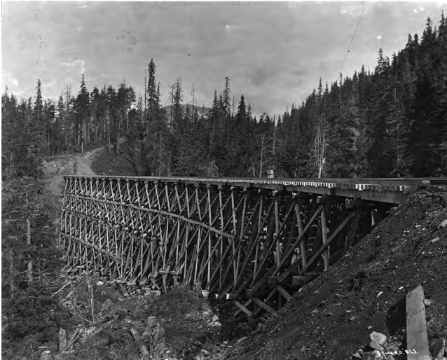
Figure 1.5 Early track construction at a trestle transition. (Courtesy of Library of Congress.)
