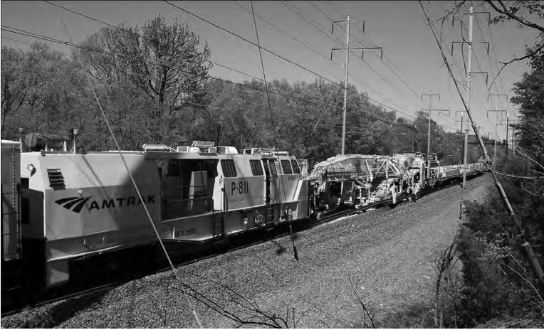
Figure 9.2 Track laying machine in operation. (Courtesy of Amtrak, Philadelphia, Pennsylvania.)
