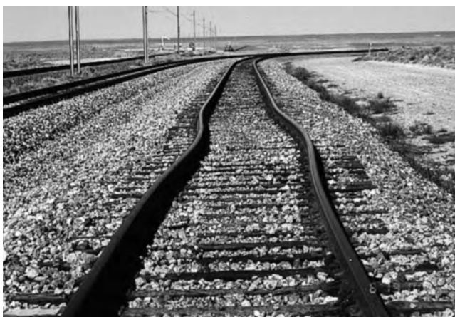
Figure 8.70 Example of track buckle over a short distance.
