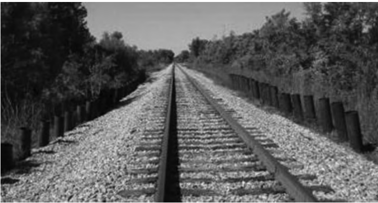
Figure 7.40 Photo of driven pipe piles to improve embankment stability.
