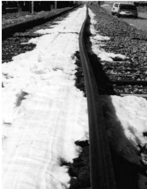
Figure 8.72 Example of track panel shift in cold weather.
