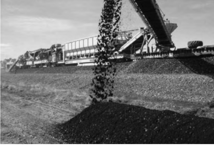
Figure 1.34 Track undercutting operation.
