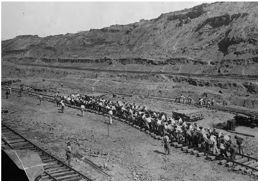
Figure 1.7 Track realignment to facilitate mechanized earthmoving in Culebra Cut of the Panama Canal, January 1912. (Courtesy of Harris and Ewing Collection, Library of Congress.)
