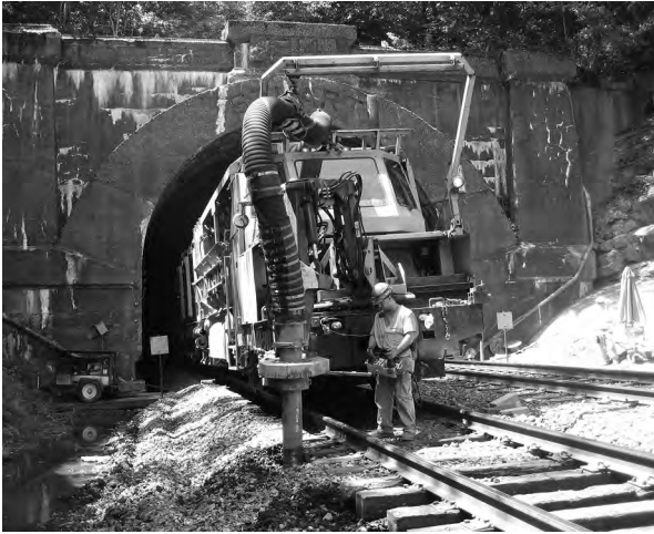
Figure 6.47 Ballast vacuum train. (Courtesy of Loram Maintenance of Way, Hamel, Minnesota.)
