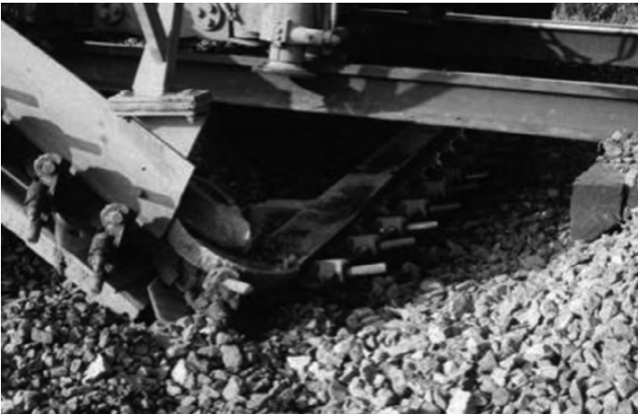
Figure 1.35 Undercutter ballast excavation chain.
