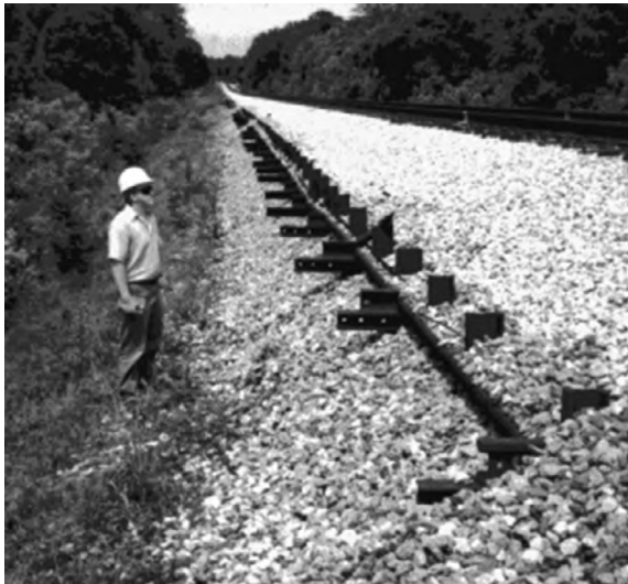
Figure 1.18 Example of rail used for embankment slope reinforcement.
