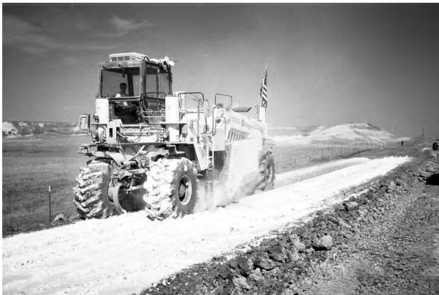
Figure 10.7 Lime admixture stabilization with high-speed mixer/polarizer.
