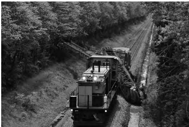
Figure 6.50 On-track “Badger” ditching machine in action. (Courtesy of Loram Maintenance of Way, Hamel, Minnesota.)
