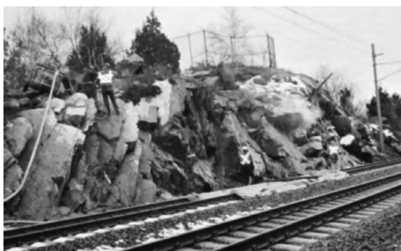
Figure 7.45 Manual rock removal and reinforcement. (Courtesy of R. Kölsch.)
