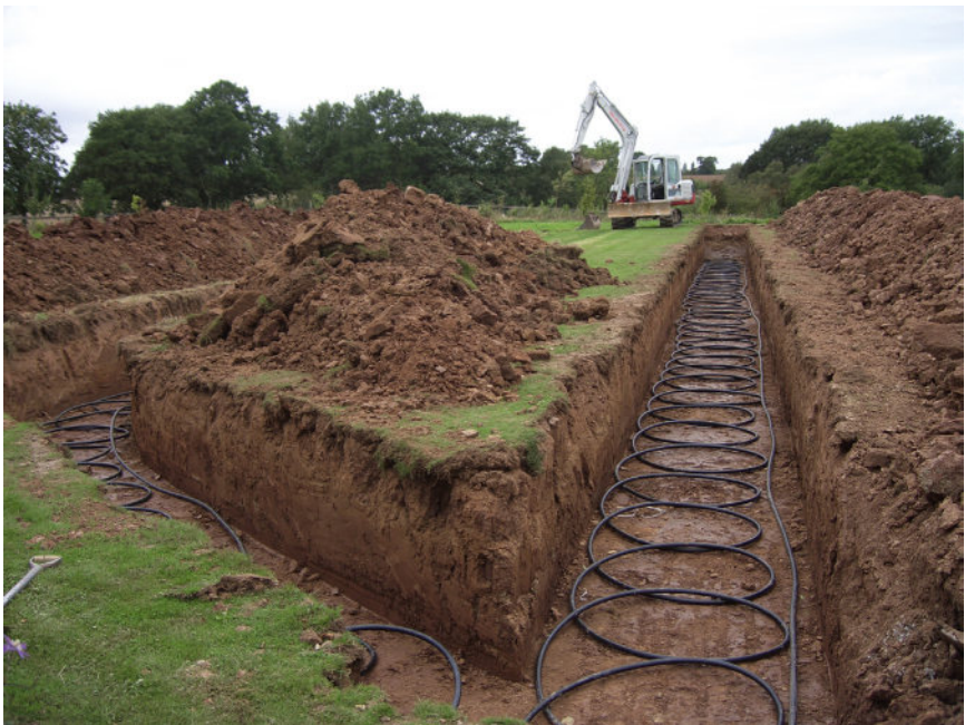
Figure 25.3 Trench for GSHP showing pipe through which glycol solution will be circulated to collect heat (Kensa).
