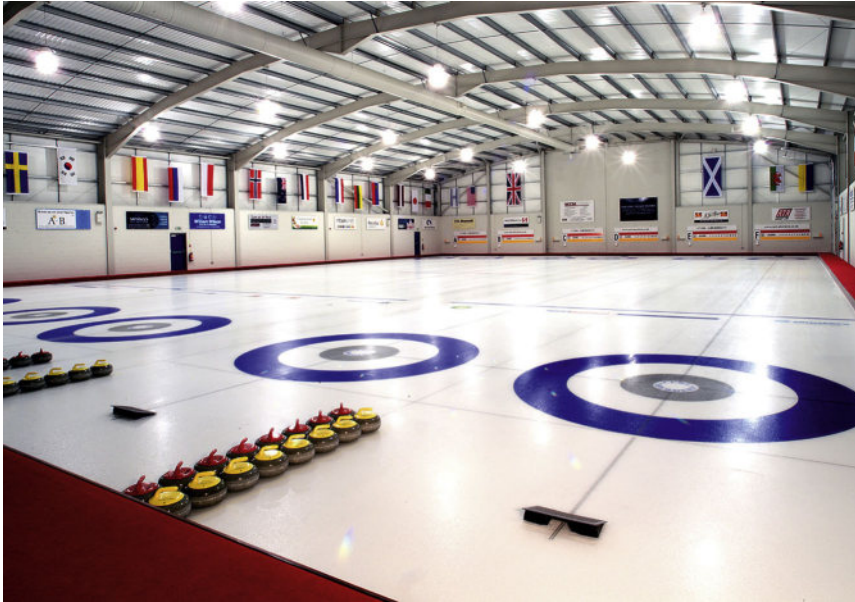
Figure 18.3 Ice rink (Star Refrigeration).
