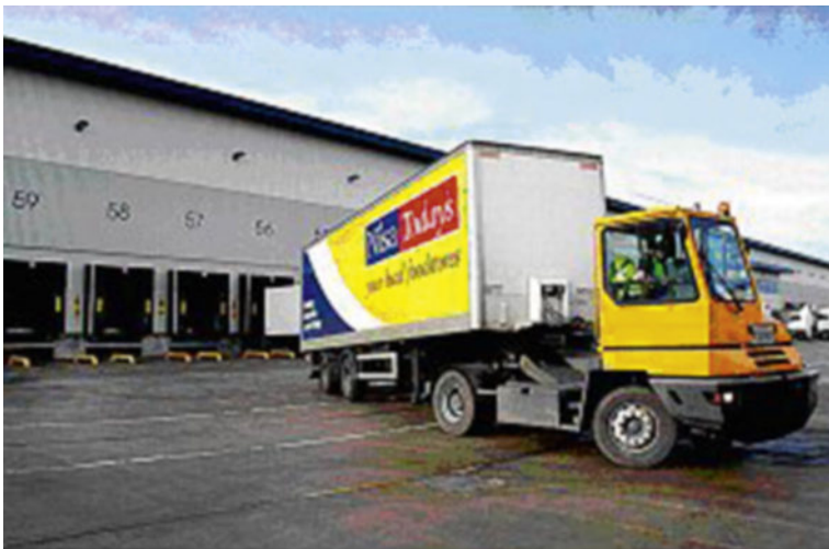
Figure 17.7 Distribution centre (Star Refrigeration).
