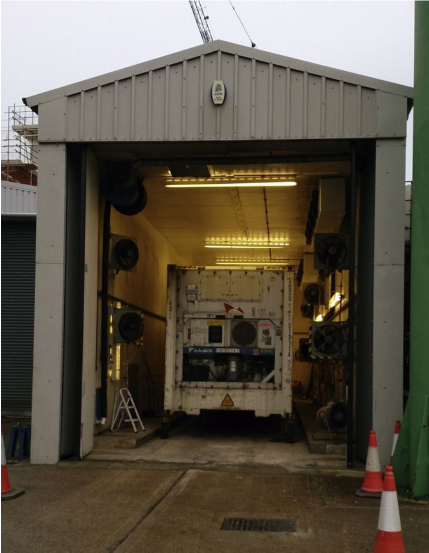
Figure 18.4 Test chamber capable of taking the largest permissible road vehicles (Cambridge Refrigeration Technology).
