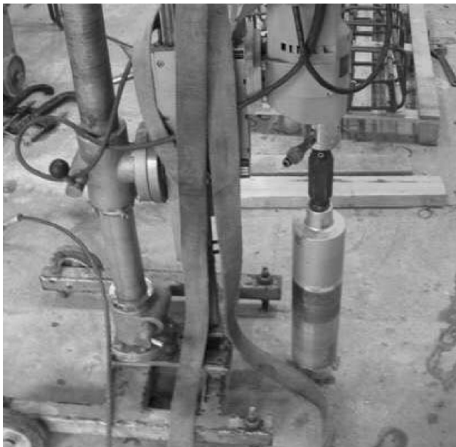
Figure 3.15 A core-cutting drill.
