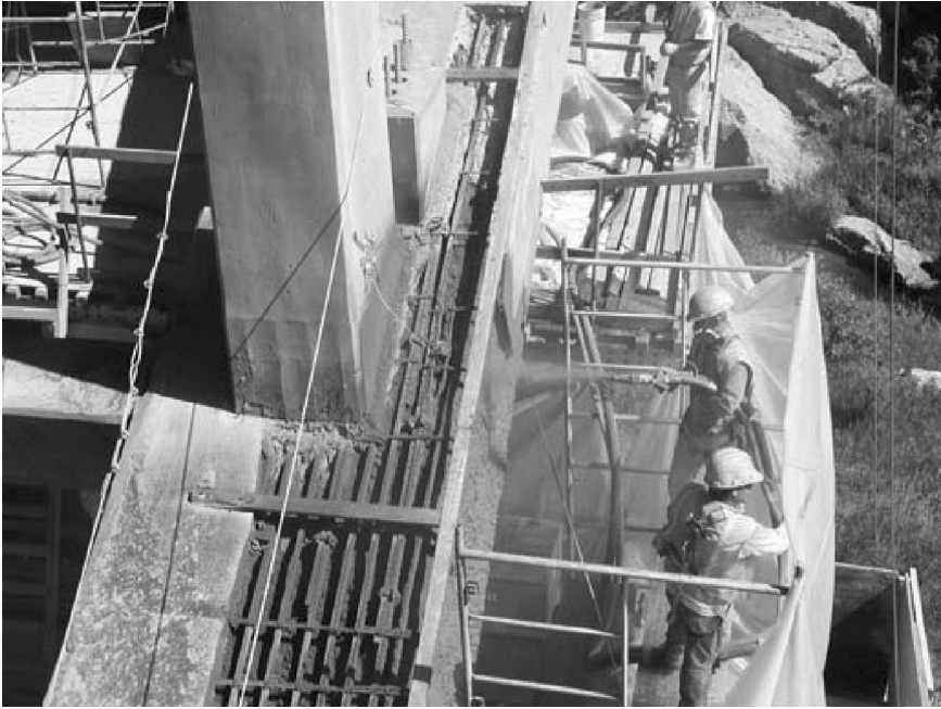
Figure 4.8 Application of shotcrete for repairing a concrete arch.
