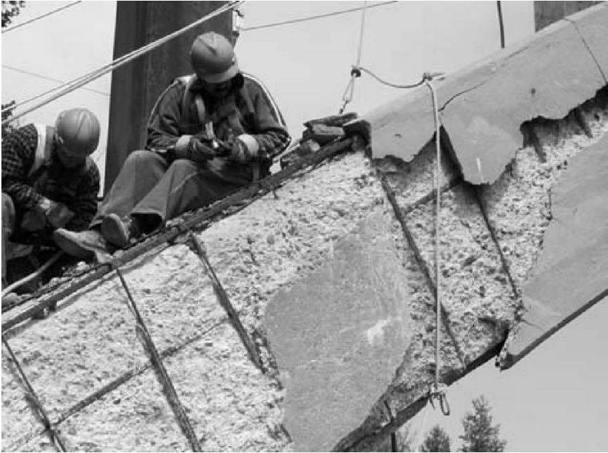
Figure 4.22 Removal of the concrete under corroded steel bars using hand tools.
