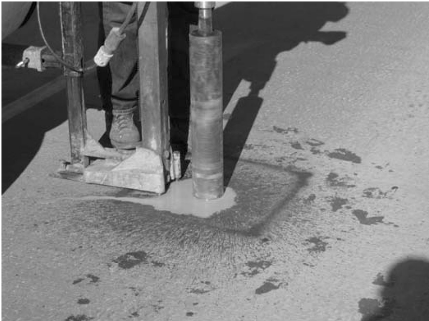
Figure 4.12 A concrete core is taken from a bridge deck.
