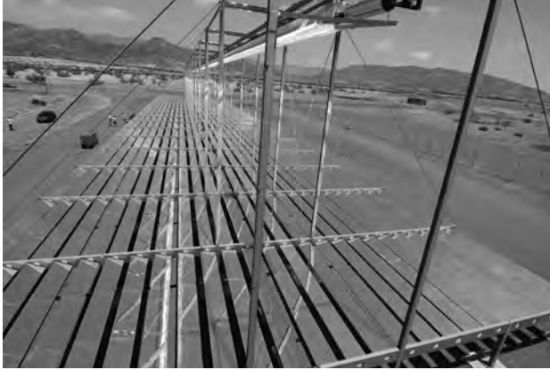
Figure 7.4 Linear Fresnel collector
