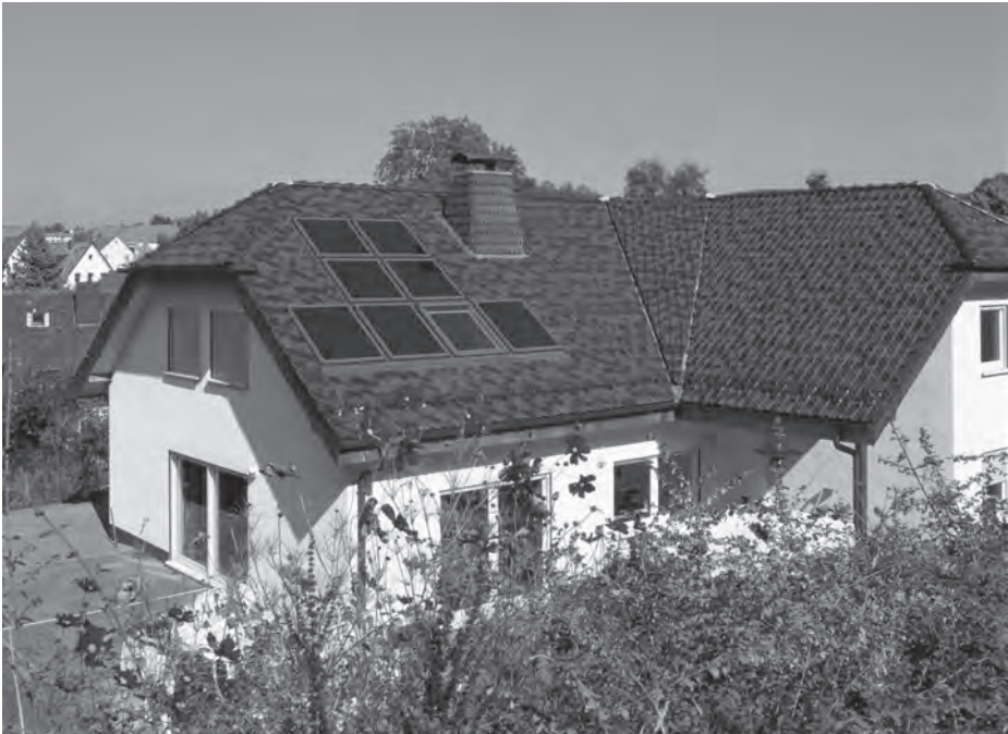
Figure 2.11 House with flat-plate collectors on the roof in Germany
