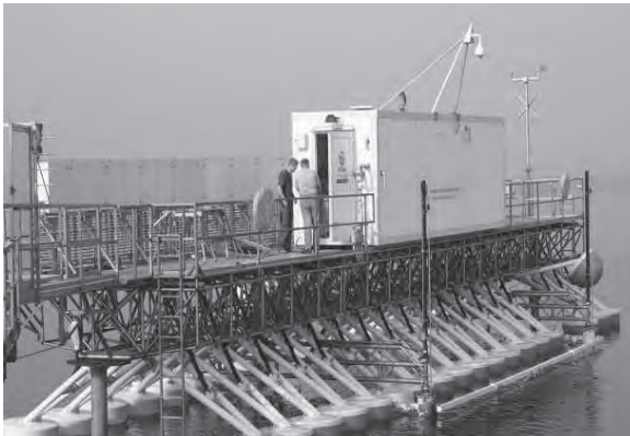
Figure 10.5 Wave Star, Nissum Bredning, Denmark (1:10 prototype, full scale 6MW) Source: Wave Star
