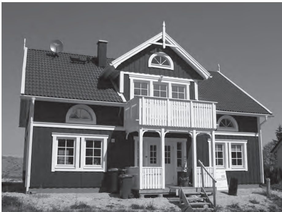
Figure 4.4 Small residential house Source: Ochsner
