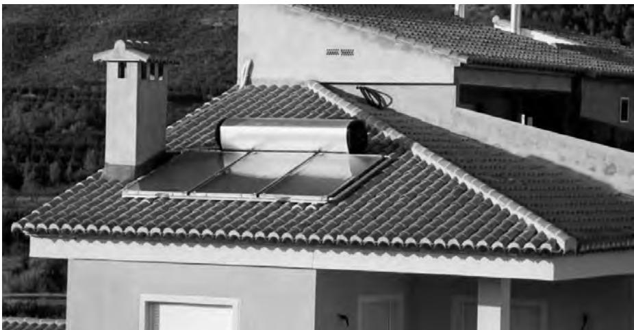
Figure 2.12 Spanish house with thermo-siphon system on the roof Source: Solahart
