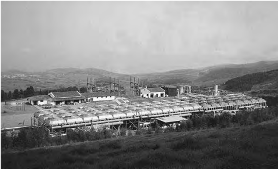
Figure 11.4 Geothermal power plant of Ribeira Grande, Azores, Portugal Source: EGEC (2008)
