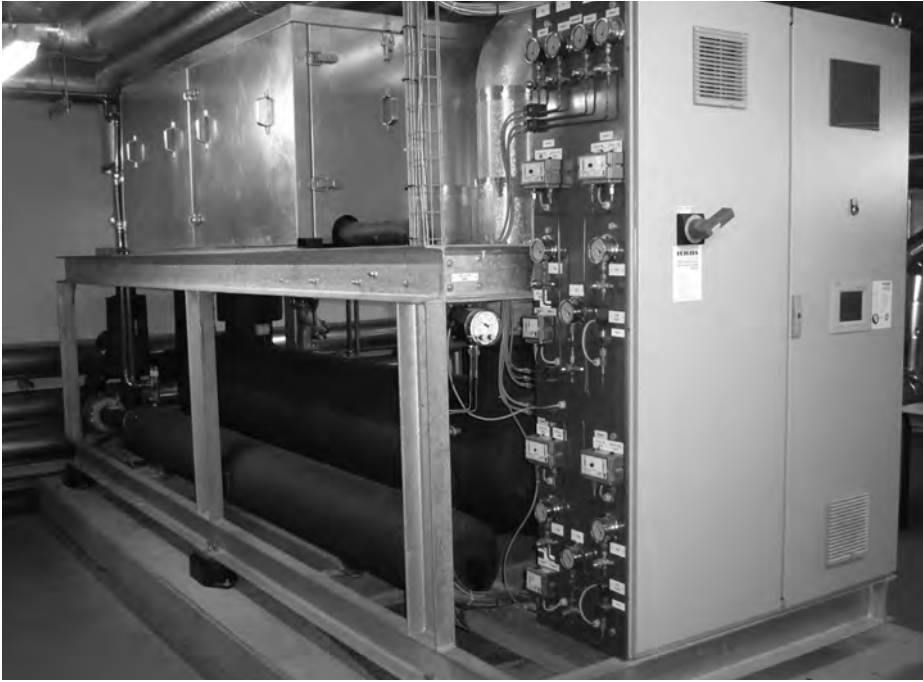
Figure 4.2 Large heat pump in an office building
