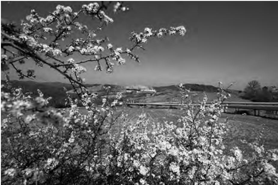
Figure 11.2 Larderello: Steam conduits through the valley Source: EGEC (2008)
