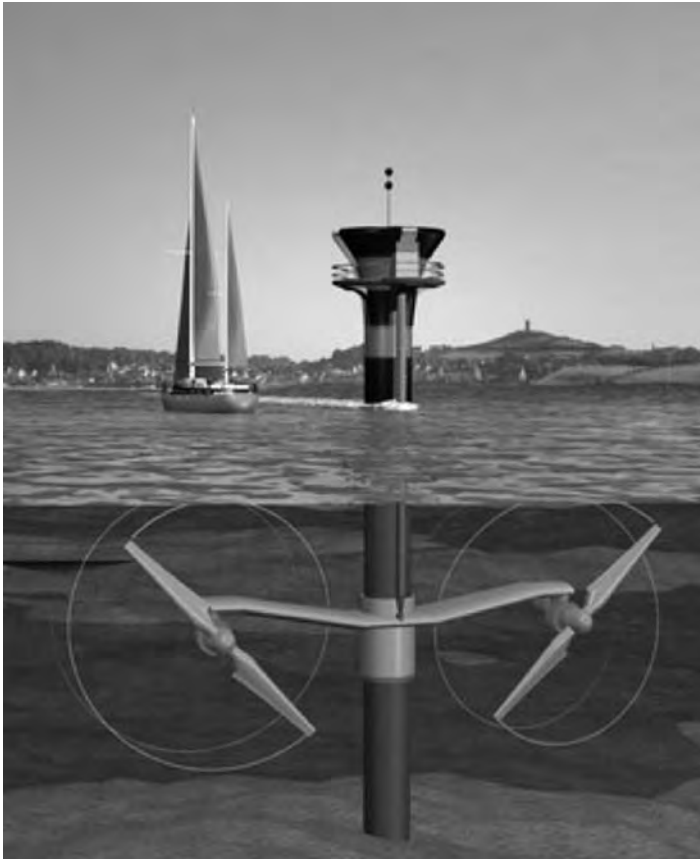
Figure 10.2 SeaGen, Marine Current Turbines, Strangford Lough, Northern Ireland (1.2MW) Source: Marine Current Turbines Limited
