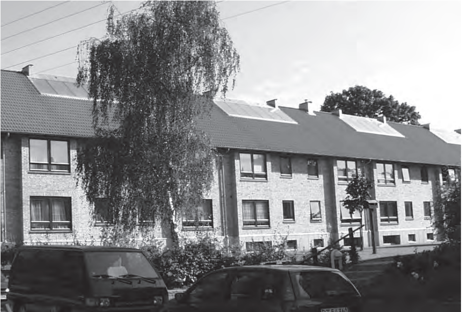
Figure 2.5 Residential building block in Denmark with flat-plate collectors on the roof Source: BATEC Solvarme
