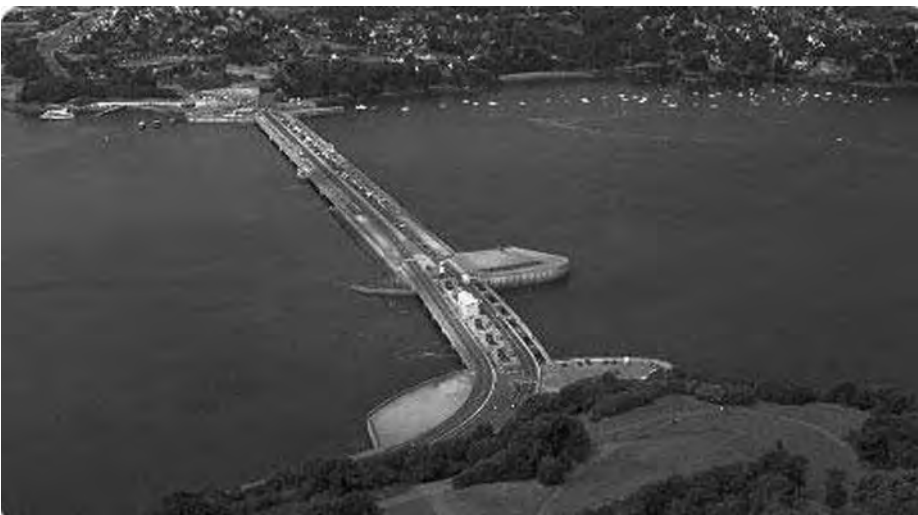
Figure 10.1 La Rance, St. Malo, France (240MW)
