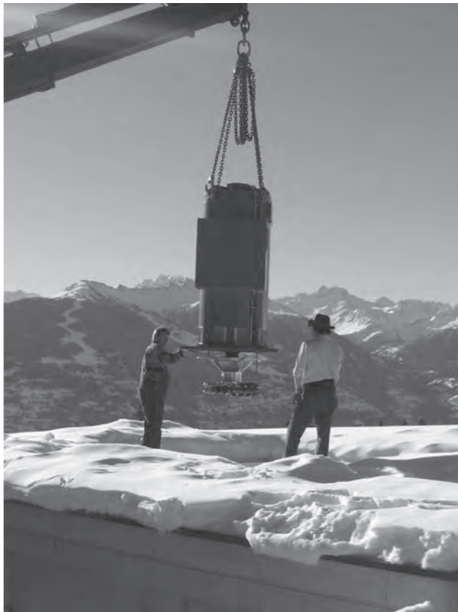
Figure 9.2 Setting of a Pelton Turbine
