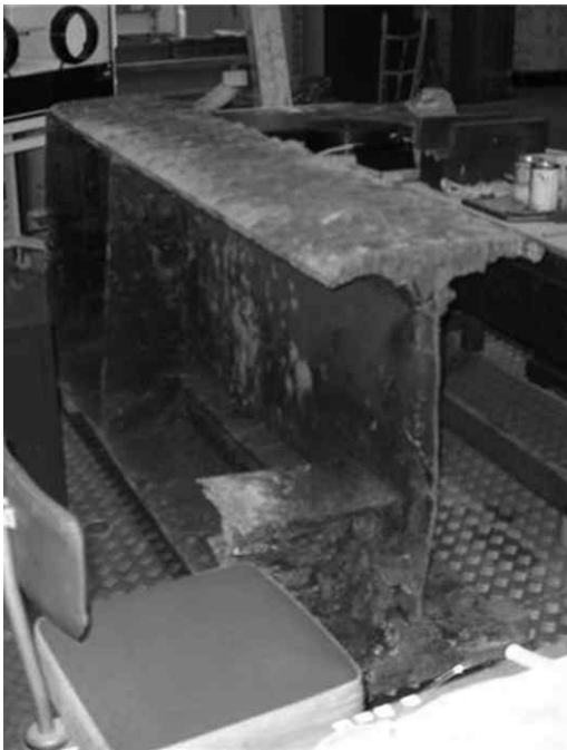
14.4 Wrought iron girder (2 m long) removed from demolished bridge.
