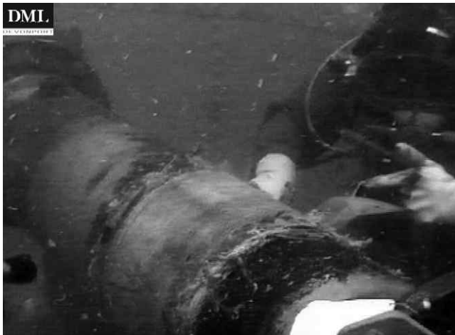
12.13 Repair of a submarine pipe (first published in Hollaway and Cadei, 2002).
