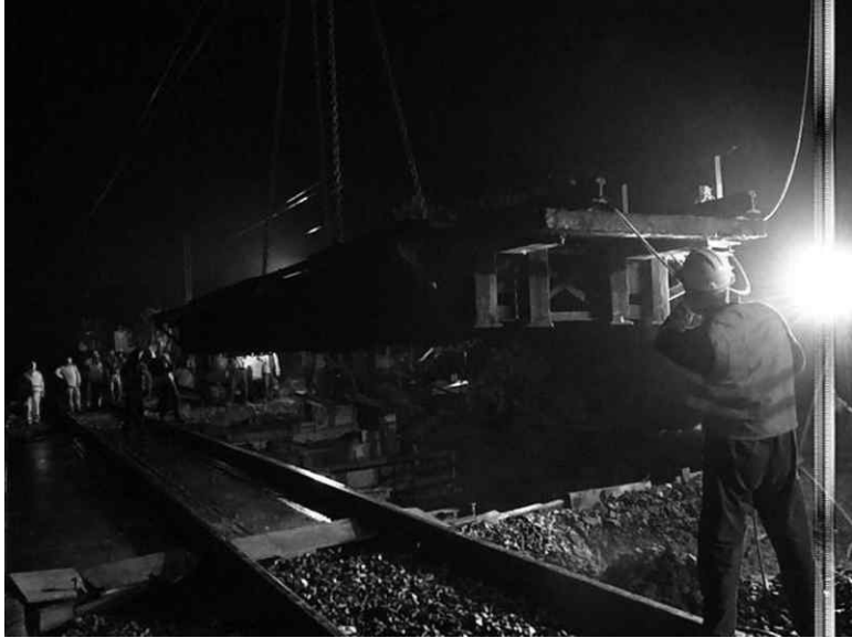
13.2 The Meschio Bridge, out of service, Italy (Pipinato et al. , 2009).
