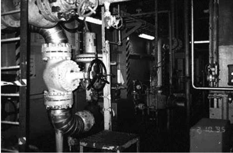
12.14 Blast strengthening of a universal column supporting a steel blast wall; strengthening material UHM carbon. (First published in Hollaway and Cadei, 2002.) (The columns are highlighted by chevrons to warn welders not to strike an arc on them.)
