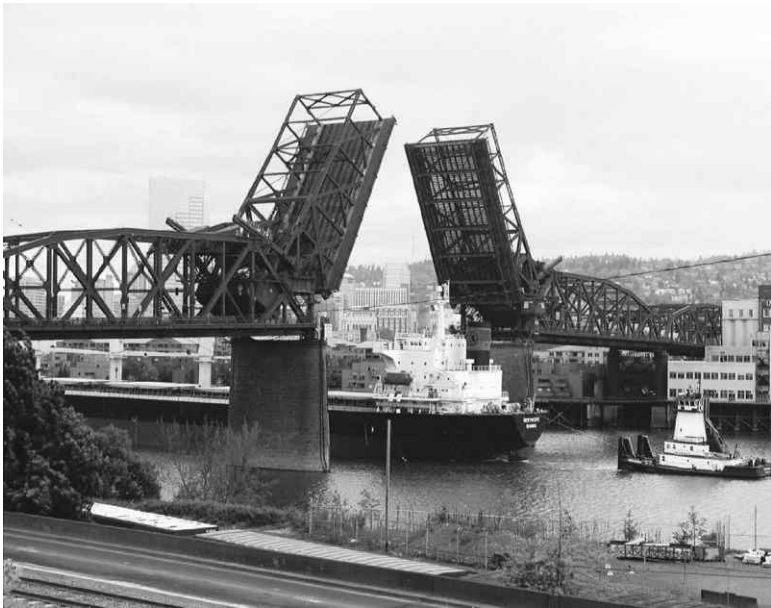
13.4 The Broadway Bridge, Portland, OR, USA.
