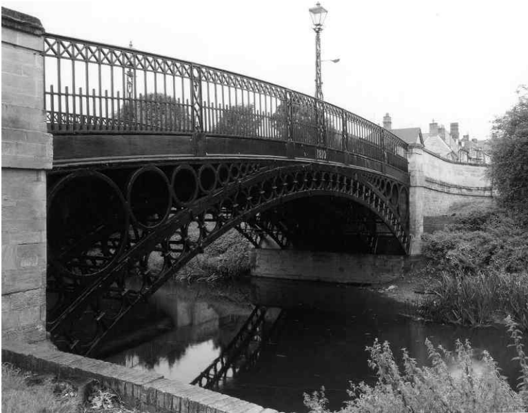
12.2 Tickford Bridge, Newport Pagnell, Northamptonshire, UK (courtesy of AECOM, UK).
