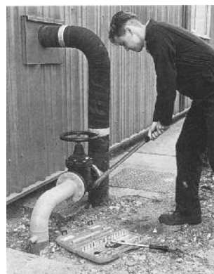
Using a torque wrench
