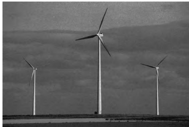
Figure 9.1.9c Wind turbines rated at 1.5 MW with 72-m-diam rotors at TVIG's Kimball wind farm installation in Nebraska. (Photo courtesy of Tennessee Valley Infrastructure Group Inc.)
