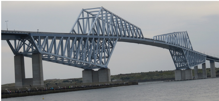
Fig. 1.21 The Tokyo Gate Bridge. (Photo by Lin.)
