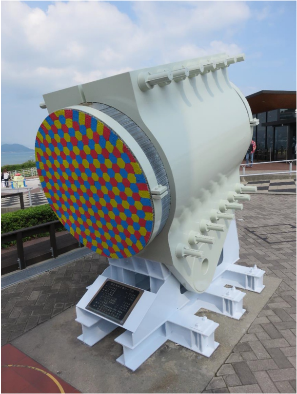
Fig. 11.16 Cross-section of the main cable in the Akashi Kaikyo Bridge. (Photo by Lin.)
