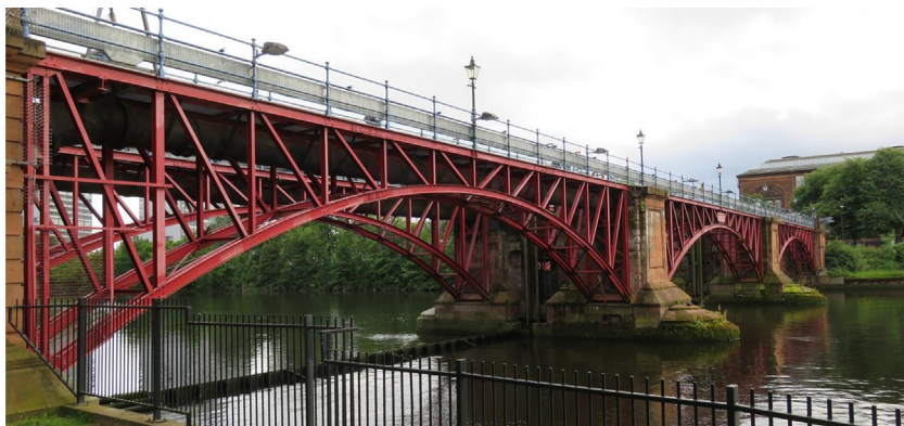
Fig. 9.15 An arch bridge with braced spandrel. (Photo by Lin.)
