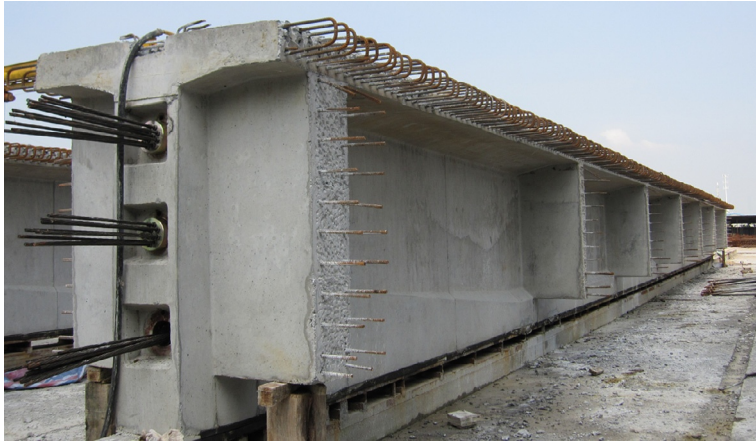
Fig. 6.7 T-section girder with prestressing. ( Photo by He. )
