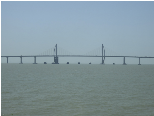
Fig. 10.6 The Jiuzhou Port Channel Bridge in Hong Kong-Zhuhai-Macao Bridge. (Photo by Lin.)
