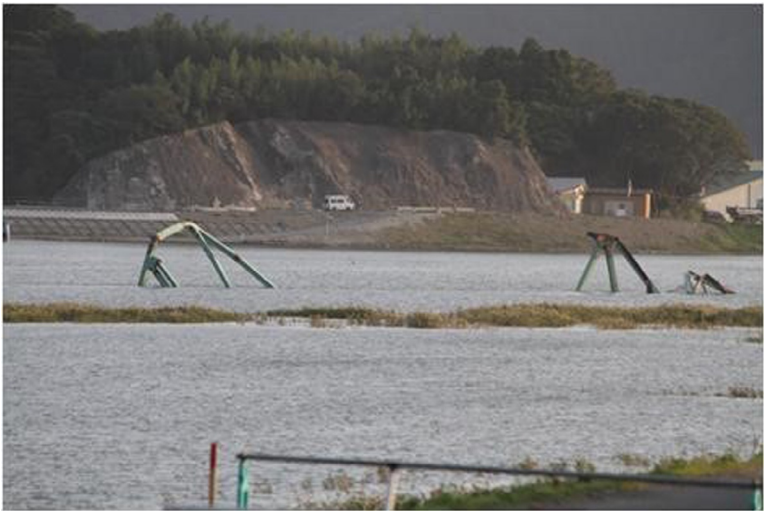
Fig. 2.9 Truss members being swept away.
