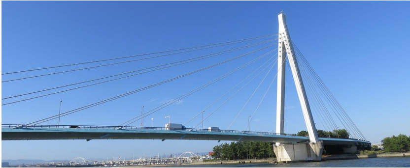
Fig. 10.9 The Tsuneyoshi Ohashi Bridge in Osaka. (Photo by Lin.)
