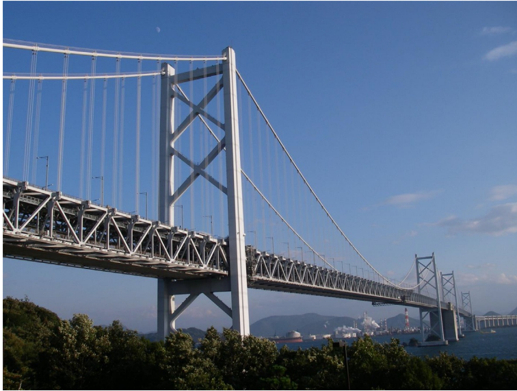
Fig. 11.19 The Seto Ohashi Bridge. (Photo by Taniguchi.)
