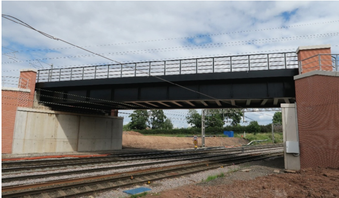
Fig. 13.8 Completed intersection bridge 5. (Photo courtesy of L.J. Butler, used with permission.)
