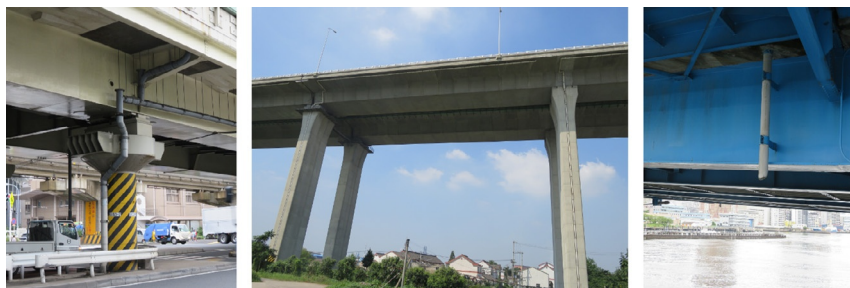
Fig. 5.2 Drainage pipes in bridges. (Photos by Lin.)
