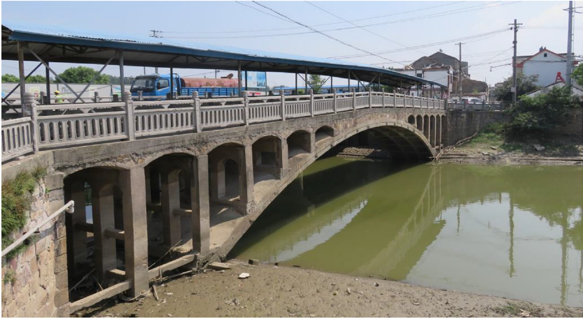
Fig. 9.6 The Stone Dock Bridge, Nanjing, China. (Photo by Lin.)
