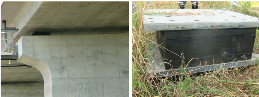
Fig. 12.12 Elastomeric bearing. (Photos by An.)
