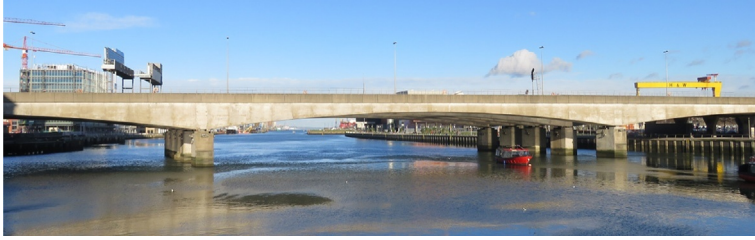
Fig. 1.16 Lagan bridge (concrete continuous girder bridge), Belfast.
