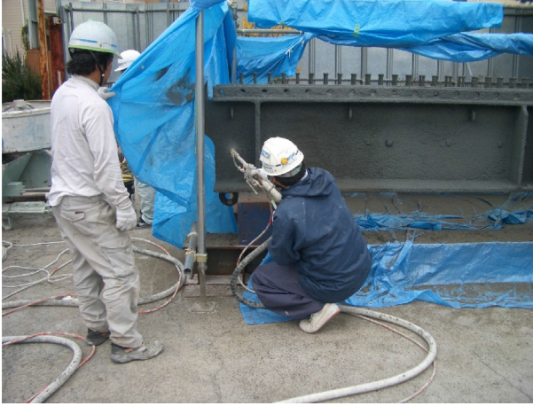
Fig. 7.20 Rubber-latex mortar coating.
