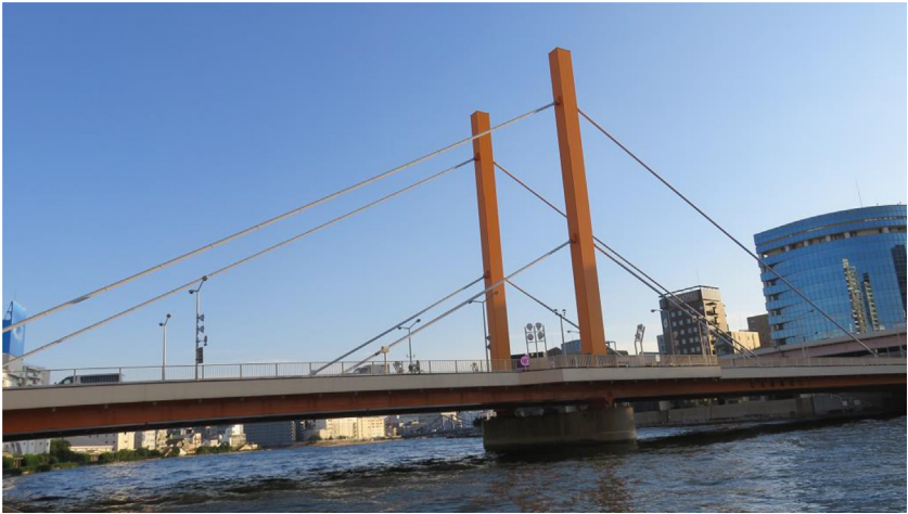
Fig. 10.3 The Shin-Ohashi Bridge in Tokyo. (Photo by Lin.)
