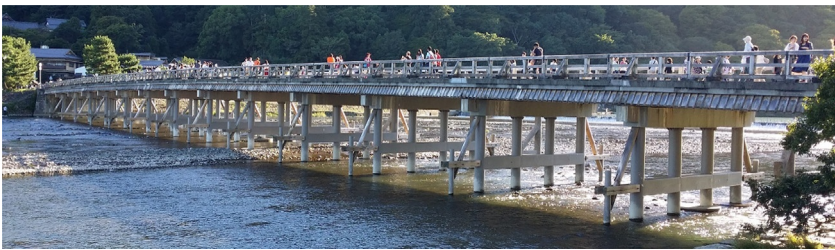
Fig. 3.3 The Togetsu-kyo Bridge in Kyoto, Japan. (Photo by Lam.)
