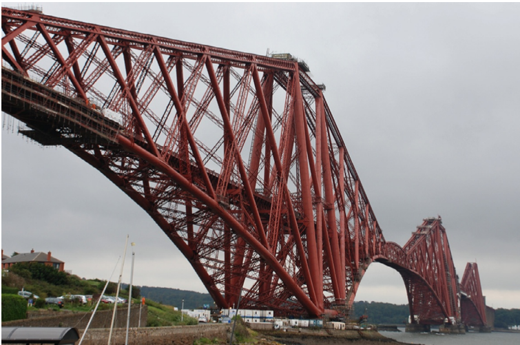
Fig. 1.8 The Forth Bridge in Scotland. (Photo by An.)
