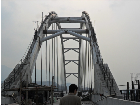
Fig. 9.20 The Guangyuan Jialing River Bridge. (Photo by Gui.)
