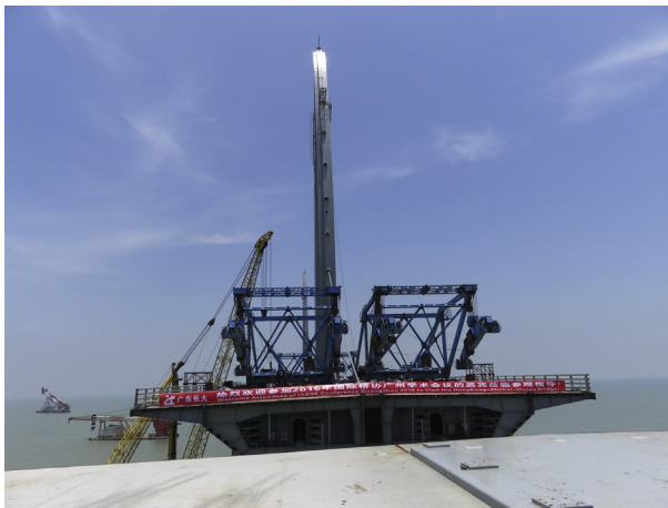
Fig. 10.21 The Jianghai Channel Bridge in Hong Kong-Zhuhai-Macao Bridge. (Photo by Lin.)
