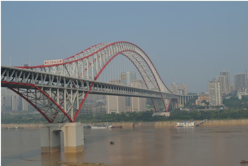
Fig. 9.2 The Chaotianmen Bridge. (Photo by Yan.)
