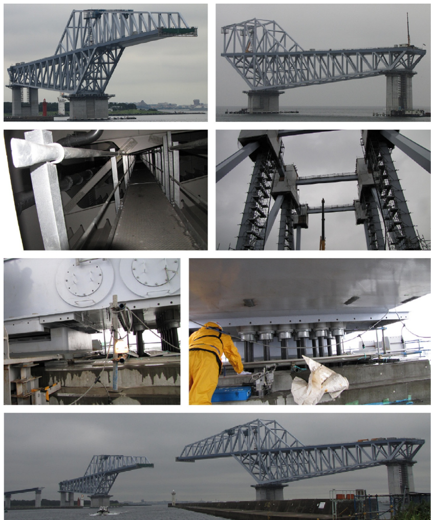
Fig. 8.12 Tokyo gate bridge during construction.
