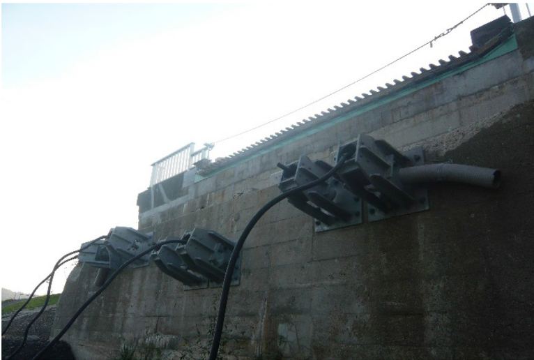
Fig. 2.7 Tearing off of fall-off prevention devices.
