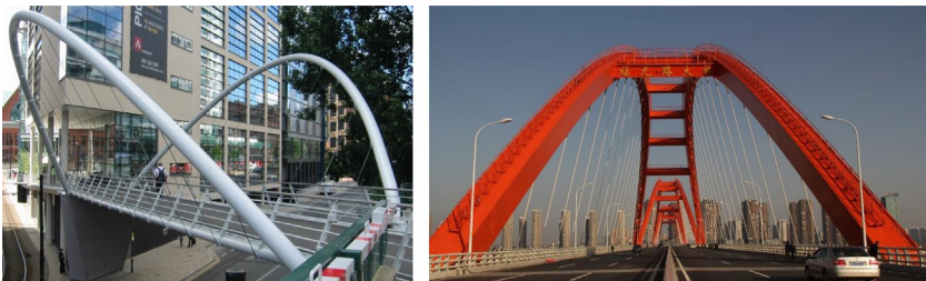
Fig. 9.17 Arch bridges with inclined ribs. (Photos by Taniguchi and He.)
