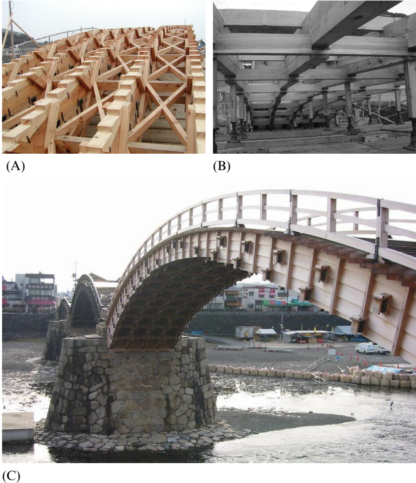
Fig. 14.10 Kintai-kyo Bridge reconstruction project. (A) New arch ribs. (B) Falseworks for arch construction. (C) After replacement. (Photos by Yoda.)
