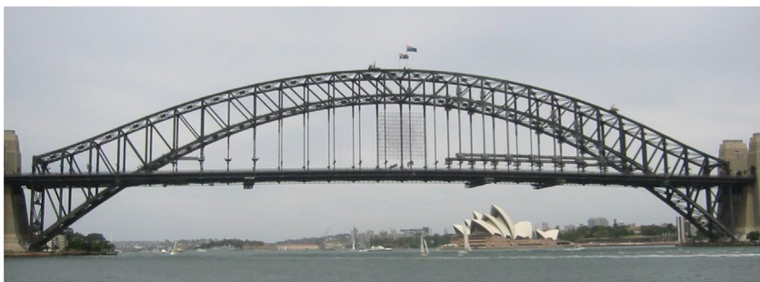
Fig. 9.18 The Sydney Harbour Bridge. (Photo by Taniguchi.)
