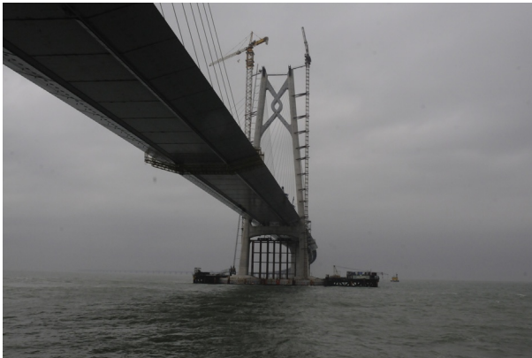
Fig. 10.18 The Qingzhou Channel Bridge in Hong Kong-Zhuhai-Macao Bridge. (Photo by Gui.)
