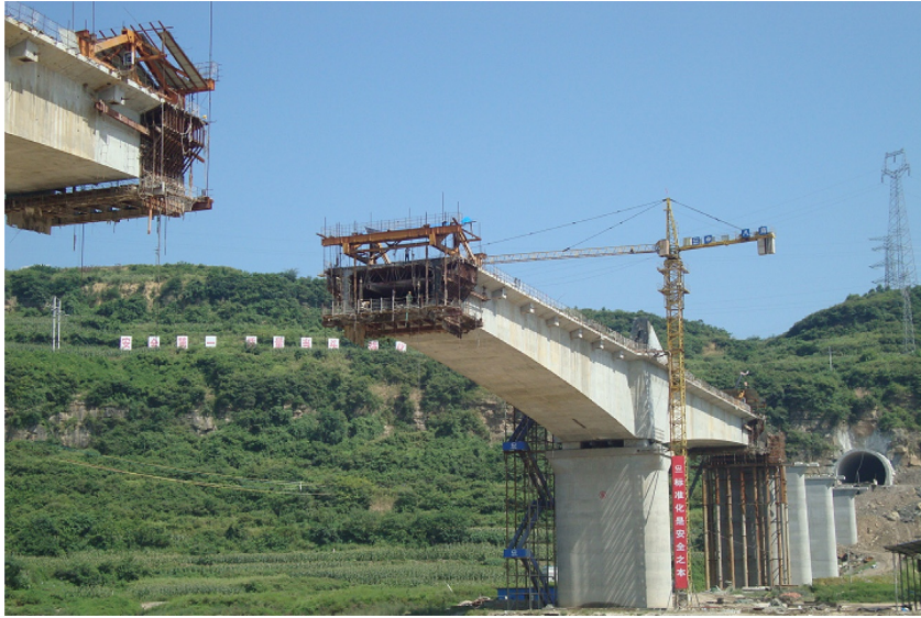
Fig. 6.10 Balanced cantilever construction. (Photo by Gui.)
