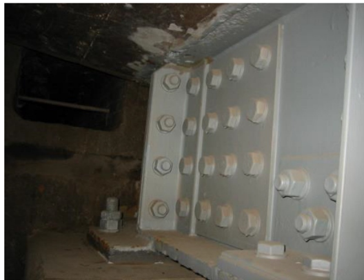
Fig. 14.8 Doubler plates strengthening examples.
