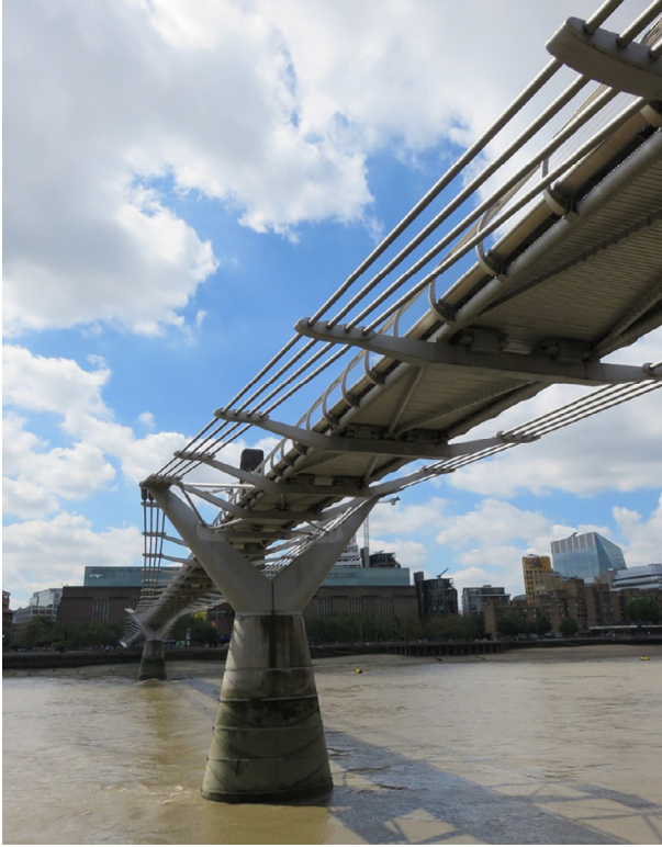
Fig. 1.12 London Millennium Footbridge. (Photo by Lin.)
