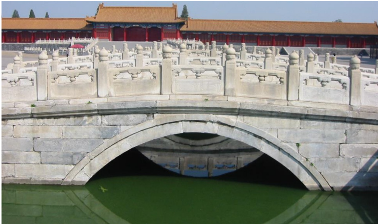
Fig. 9.5 An arch bridge in the Forbidden City, Beijing, China. (Photo by Yoda.)
