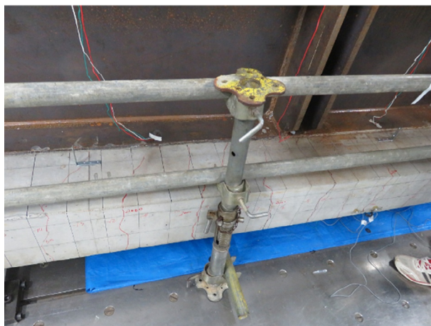
Fig. 7.11 Cracking of concrete slab under negative bending moment. (Photo by Lin.)
