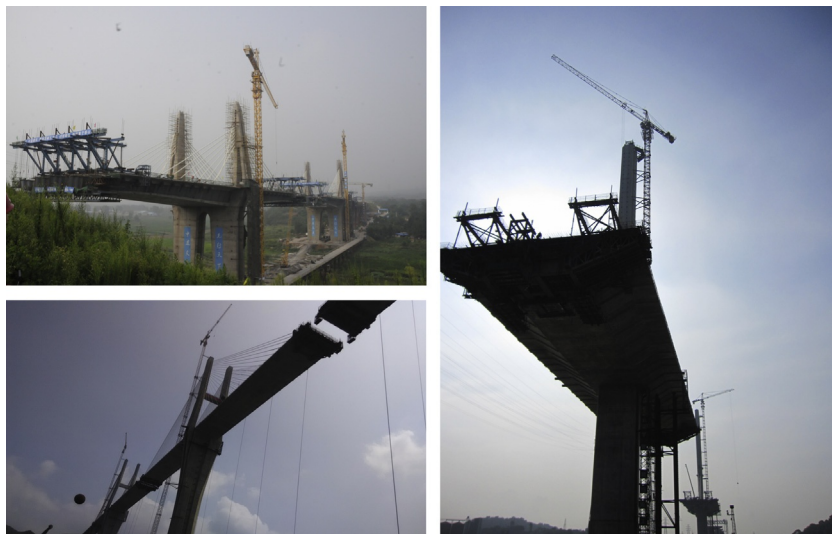
Fig. 10.27 Pictures of cable-stayed bridges during construction.
