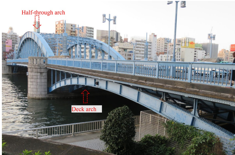
Fig. 9.11 Deck arch and half-through arch (the Komagata-bashi Bridge in Tokyo). (Photo by Lin.)
