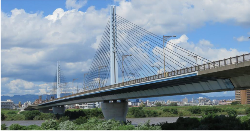
Fig. 10.15 The Sugaharashirokita Oohashi Bridge in Osaka. (Photo by Lin.)
