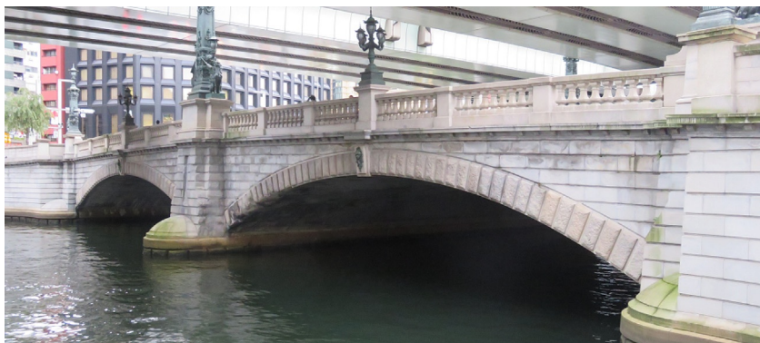
Fig. 3.1 The Nihonbashi bridge. (Photo by Lin.)
