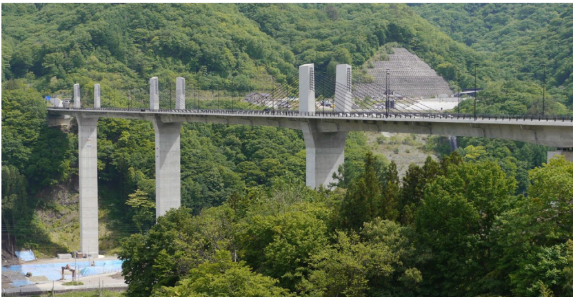
Fig. 10.16 The Yanba Bridge, Gunma Prefecture. (Photo by Taniguchi.)
