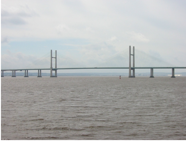
Fig. 10.17 The Second Severn Crossing. (Photo by Yoda.)
