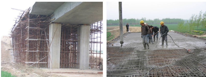
Fig. 6.9 Posttensioned concrete bridge, cast-in-place. (Photos by Ding.)
