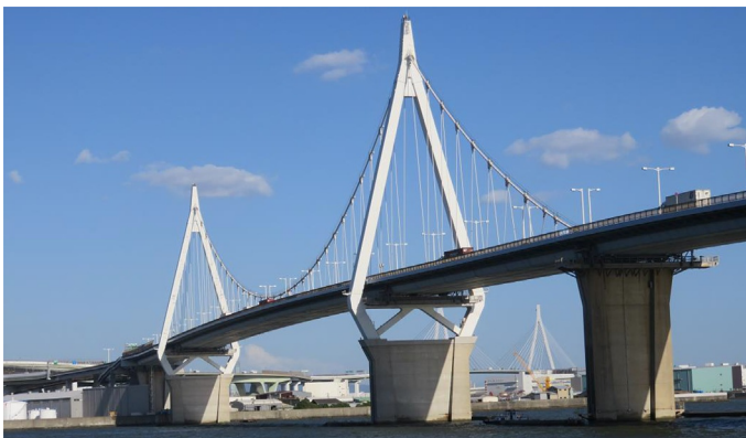
Fig. 11.12 The Konohana Bridge (self-anchored suspension bridge) in Osaka, Japan. (Photo by Lin.)
