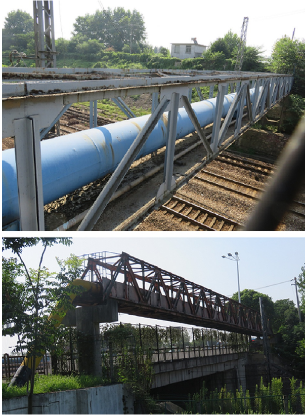
Fig. 1.15 Pipeline bridges. (Photos by Lin.)
