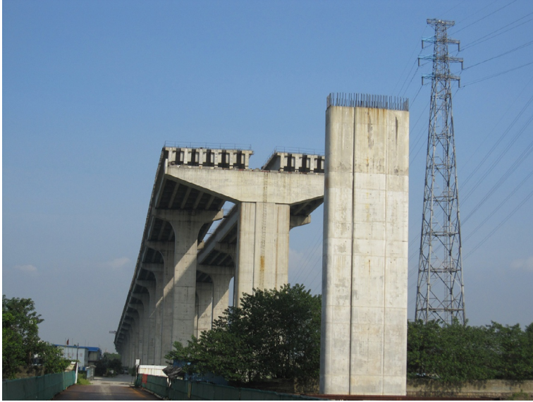
Fig. 6.11 Precast T-beams. ( Photo by He. )
