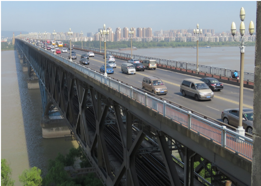
Fig. 5.1 The Nanjing Yangtze River Bridge. (Photo by Lin.)
