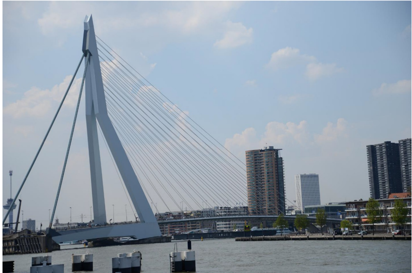
Fig. 10.8 The Erasmus Bridge in Rotterdam (1998). (Photo by An.)
