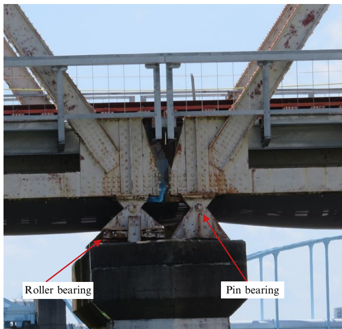
Fig. 12.4 Roller bearing and pin bearing. (Photo by Lin.)
