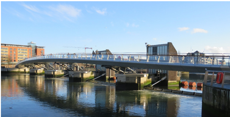
Fig. 1.13 Lagan Weir Footbridge. (Photo by Lin.)
