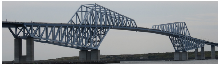
Fig. 8.13 Tokyo gate bridge after construction.
