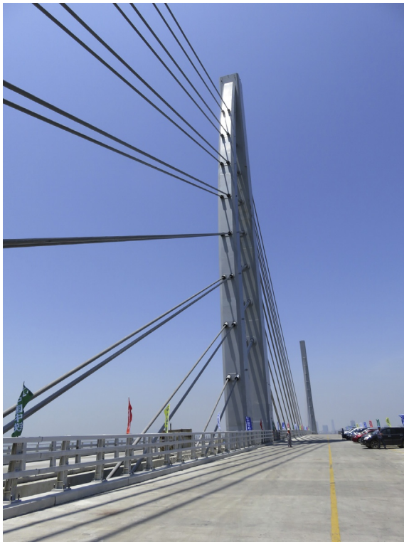
Fig. 10.20 The Jiuzhou Port Channel Bridge in Hong Kong-Zhuhai-Macao Bridge. ( Photo by Lin. )
