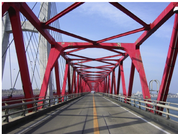
Fig. 14.9 The former Choshi Bridge (before removal).
