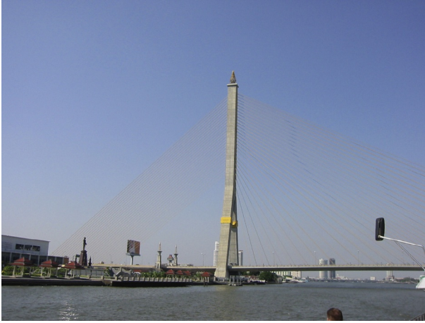
Fig. 10.19 The Bangkok Ring Road Cable-stayed Bridge, Thailand. ( Photo by Yoda. )
