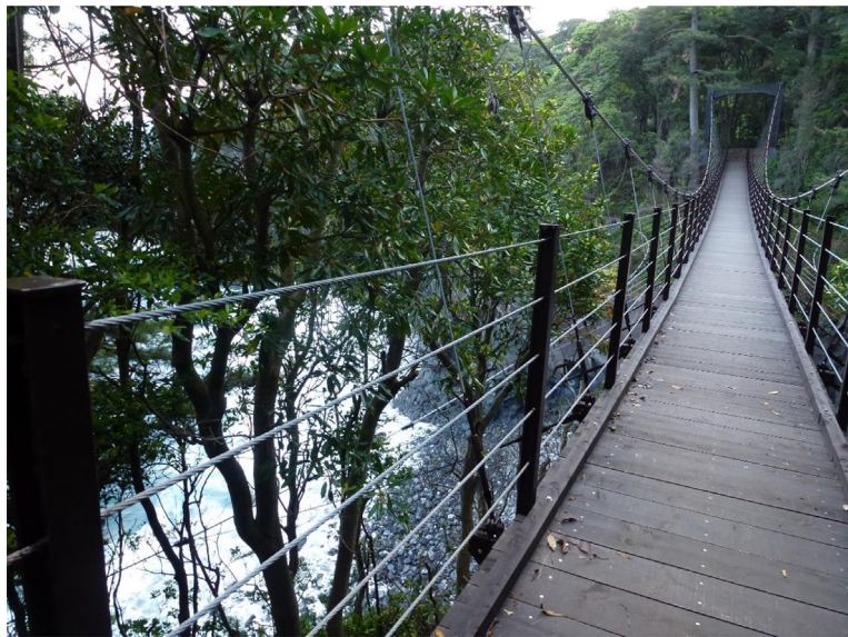
Fig. 11.4 A suspension bridge in Izu, Japan. (Photo by Lin.)
