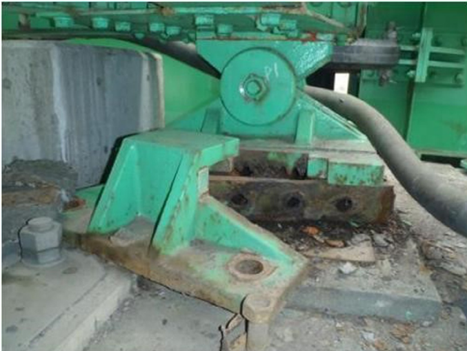
Fig. 2.4 Damaged bearing.
