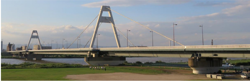
Fig. 10.4 The Toyosato-Ohashi Bridge in Osaka. (Photo by Lin.)
