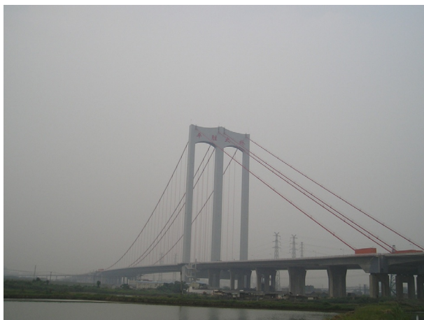
Fig. 11.8 The Pingsheng Bridge Guangdong, China. (Photo by He.)
