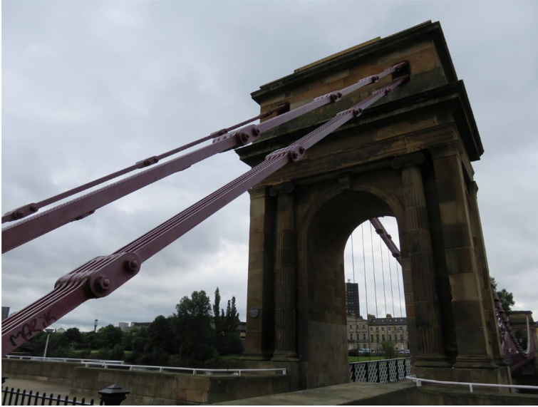
Fig. 11.14 The South Portland Street Suspension Bridge in Glasgow. (Photo by Lin.)
