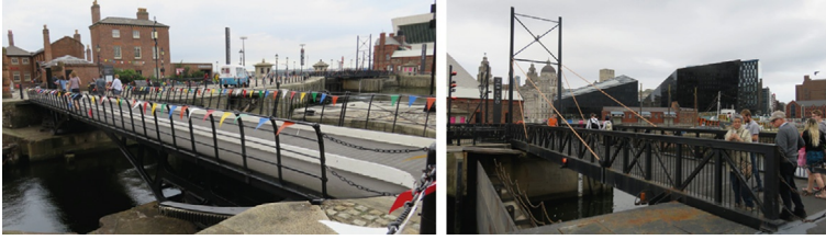
Fig. 1.5 Two swing bridges in Liverpool. (Photos by Lin.)
