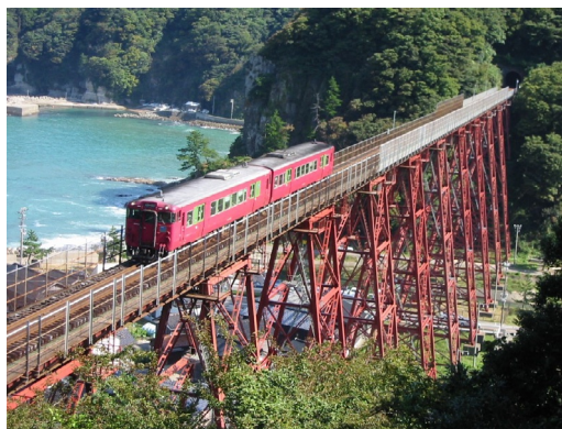
Fig. 1.11 The former Amarube Bridge (a steel trestle railway bridge). (Photo by Yoda.)
