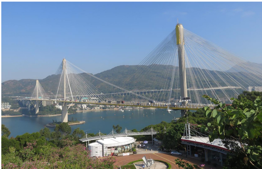
Fig. 10.12 The Ting Kau Bridge in Hong Kong. (Photo by Lin.)
