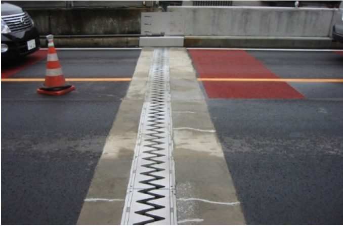
Fig. 5.4 Bridge expansion joint.
