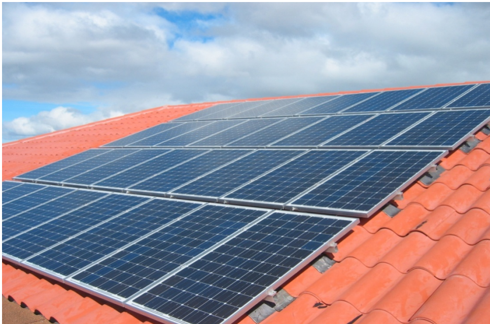
Figure 1 - Picture shown on a Spanish tile barrel roofing using lead flashings.
