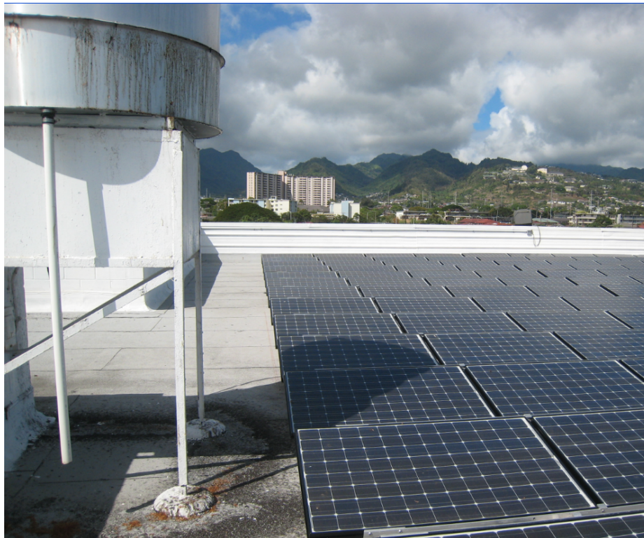
Figure 4-Shading of an array
