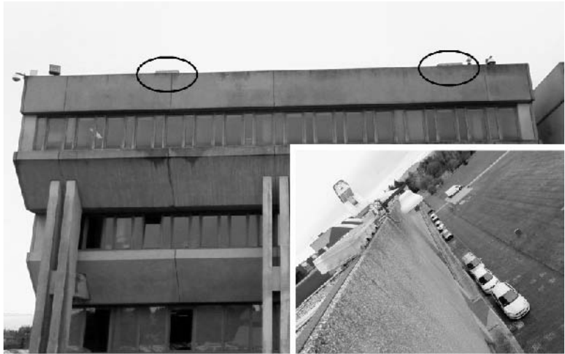
FIGURE 11.8 The prototype installed on the roof of the university building. Inside the circles, the two arrays. The microphones are protected from the weather by a waterproof box.
