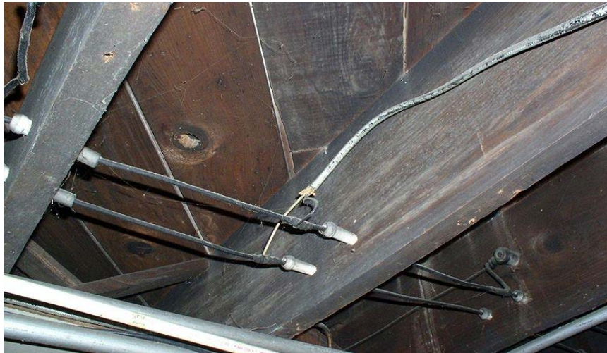
Wiring running through tubes, and turning a corner supported by a knob. Notice the direct splice with more modern (1950s-era) NonMetallic sheathed cable. This type of connection is forbidden by NEC electrical code, and other methods should have been used.
