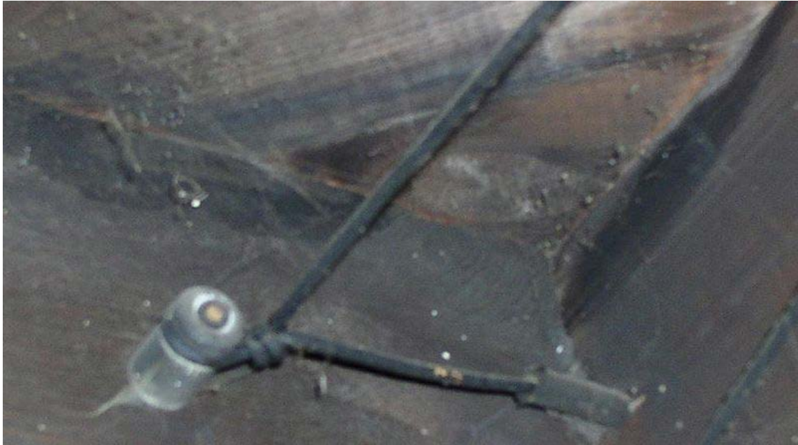
Knob supporting a wire change in direction.
