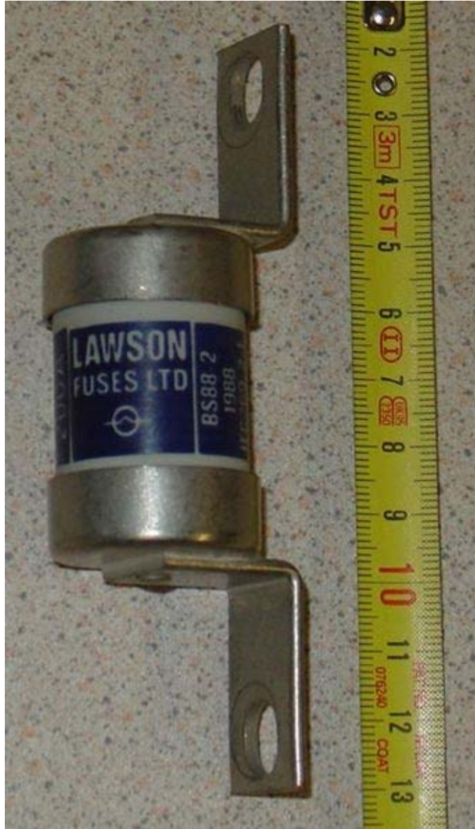
200 A Industrial fuse. 80 kA breaking capacity.
