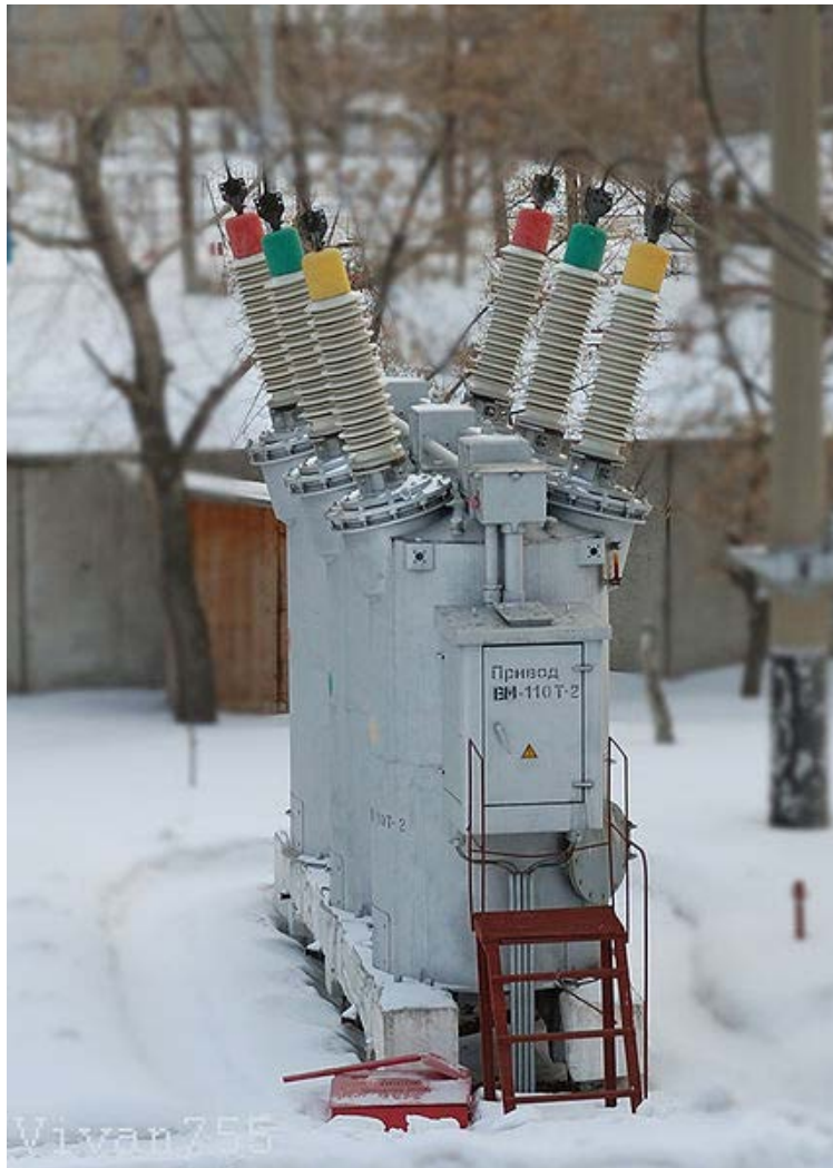
Russian 110 kV oil circuit breaker
