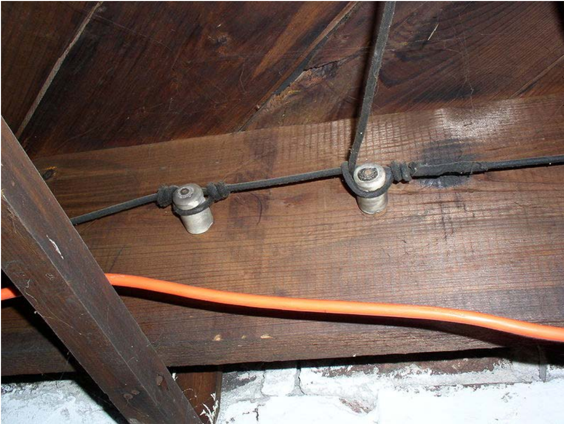
Knob-and-Tube wiring
