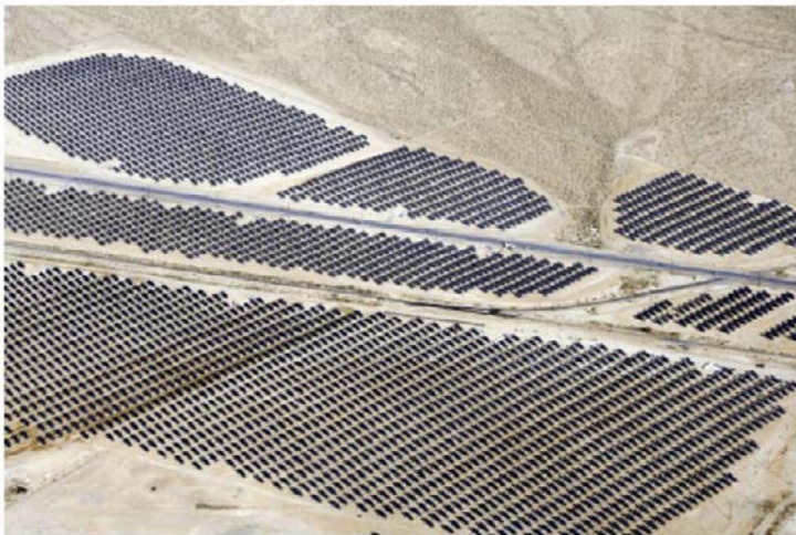
Figure 29. Representative Solar PV Plant: Nellis Air Force Base (Nevada)
