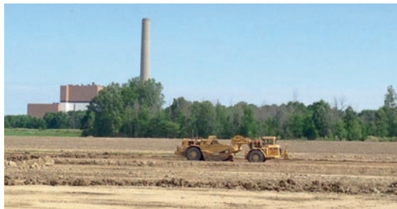
Fig. 6.9 Construction activity for the second canal expansion
