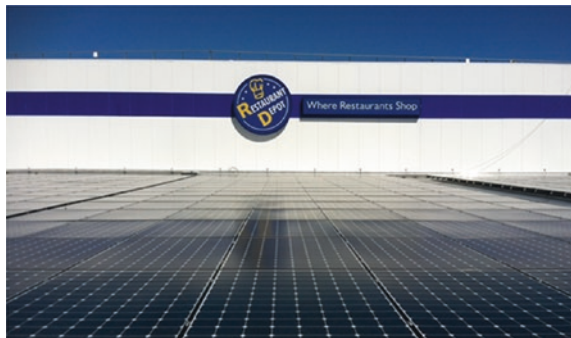
Fig. 4.3 View from the Jetro Cash and Carry rooftop. Source http://www.coned.com/newsroom/news/pr20131212.asp
