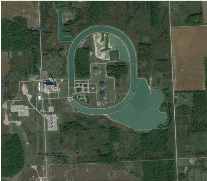
Fig. 6.13 Aerial view of Greenwood energy center shows the cooling canal (before the start of 2015 construction), the secondary impoundment basin, and James Bay
