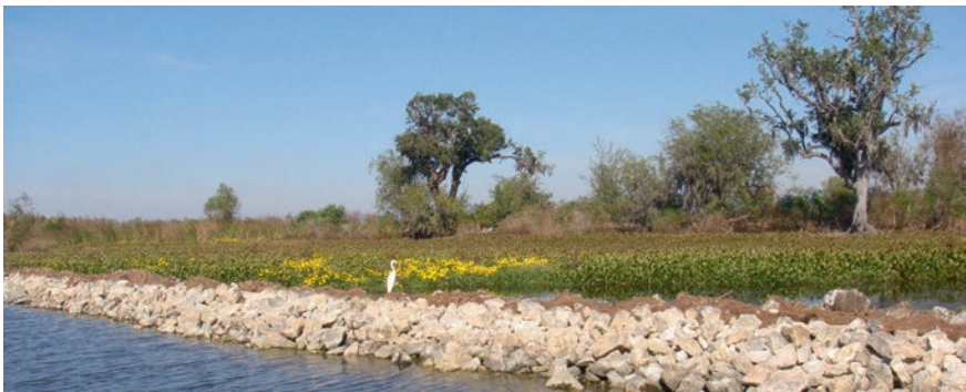
Fig. 8.11 The Bayou Segnette Cypress Reforestation project in the Barataria Preserve included construction of protective rock jetties to reduce erosion
