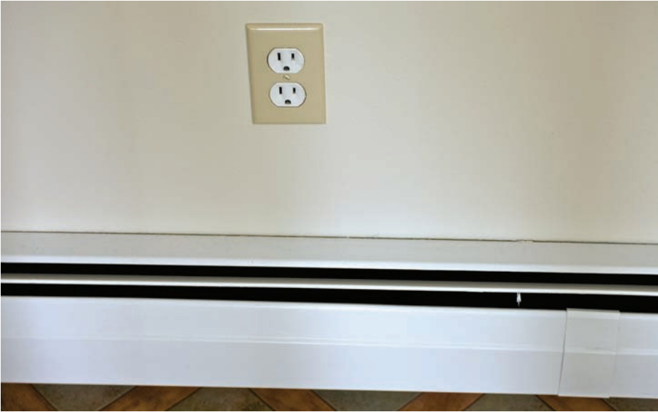
FIGURE G-16 This wall receptacle is improperly located above a baseboard heat unit.
