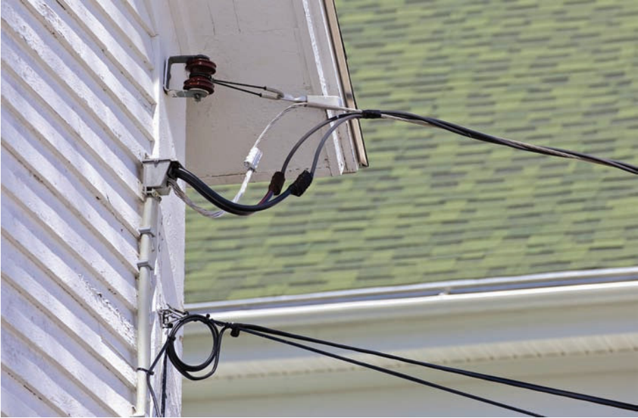
FIGURE G-18 Service drop with point of connection and weatherhead.
