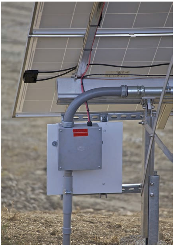
FIGURE 7-3 Underground raceway placement must be coordinated with equipment position if the conduit riser is to be plumb.
