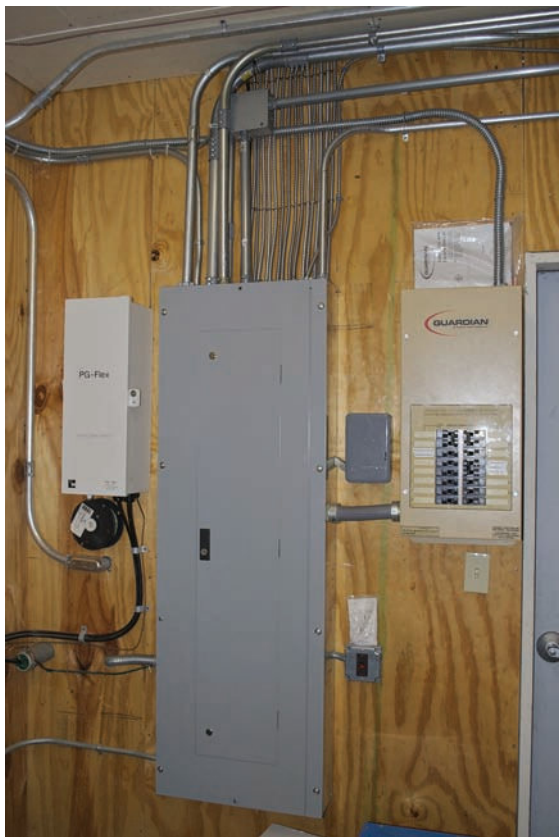
FIGURE 13-3 The automatic transfer switch often performs other functions, such as sensing a utility outage, starting the generator, and returning to utility power after the outage has ended.
