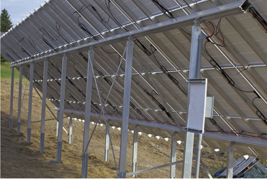
FIGURE 14-5 Sonotube concrete footings should not be too far out of the ground so as to limit pitting from the weather.
