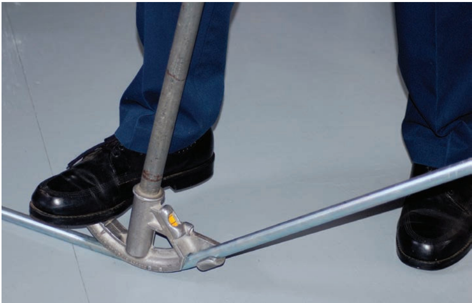
FIGURE 7-11 Bending EMT.
