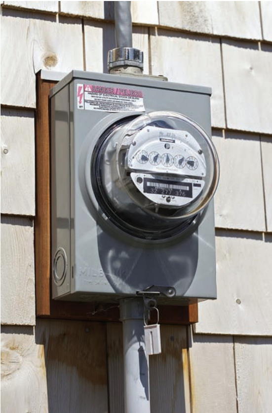
FIGURE 4-5 This meter socket is in back-to-back configuration with the entrance panel on the inside of the house. The polyvinyl chloride (PVC) conduit coming out of the bottom of the meter socket contains the grounding-electrode conductor.
