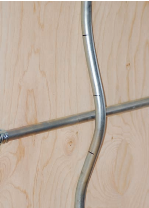
FIGURE 7-13 A three-point saddle bend, which is used where a single pipe must be crossed.
