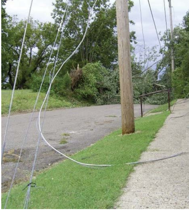
Figure 8.10 Sometimes fallen power lines appear to be harmless and de-energized because no arcs are occurring, when in fact they are energizing the ground and any other metal objects around them.
