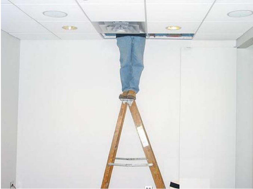
Figure 11.10 Never stand on the top platform of a stepladder. The odds of falling are dramatically increased.
