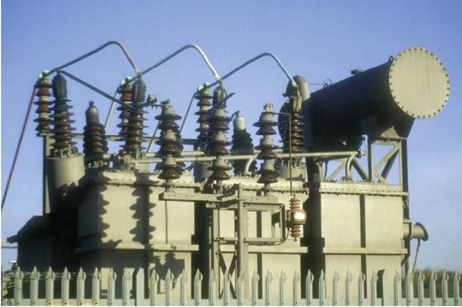
Figure 8.3 A voltage transformer is used to convert high voltage supply current to a lower voltage.
