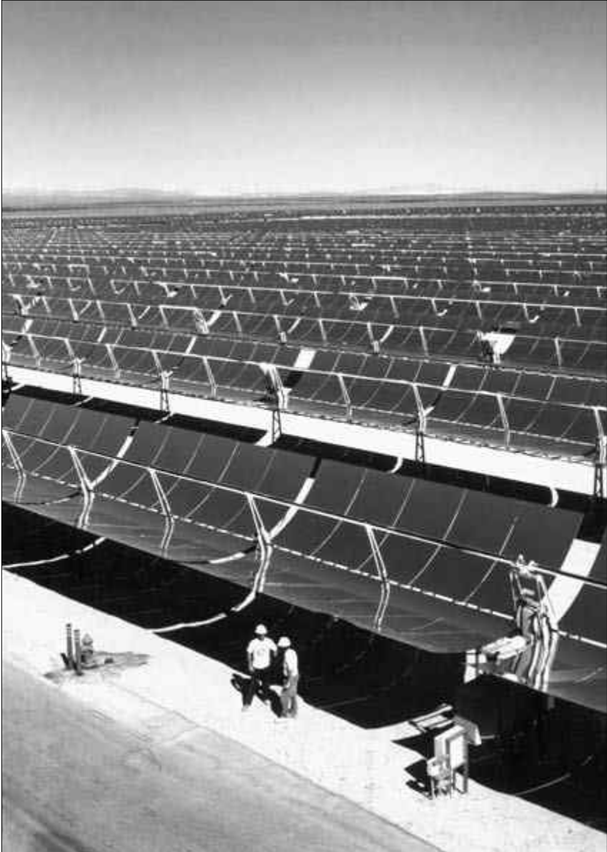
Solar thermal panels direct the sun onto pipes to heat fluid, which provides the steam that drive generators. (Courtesy of the National Renewable Energy Laboratory.)
