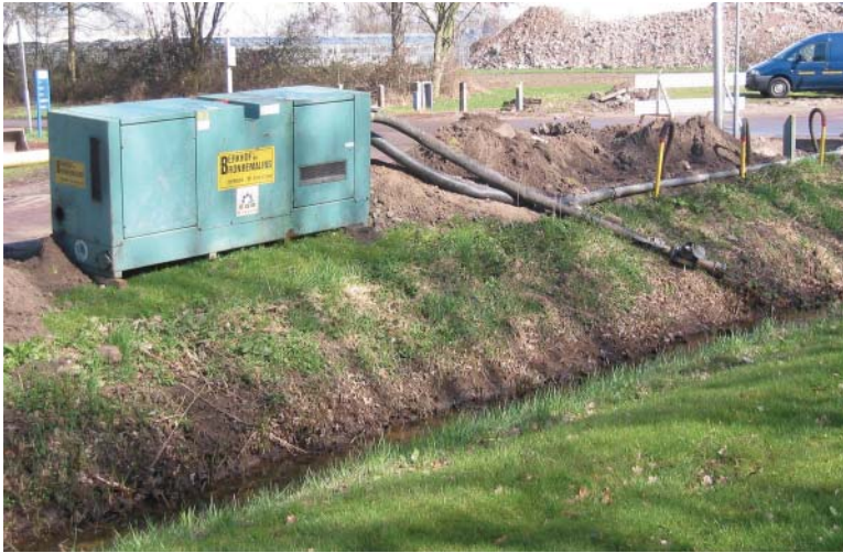
Figure 2.48 Spring dewatering. Source: Wikipedia.
