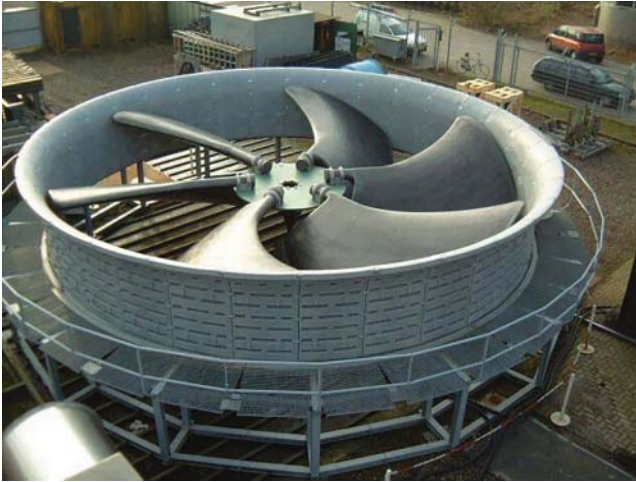
Figure 9.57 Hyper fan for refrigeration installation. Source: Howden.
