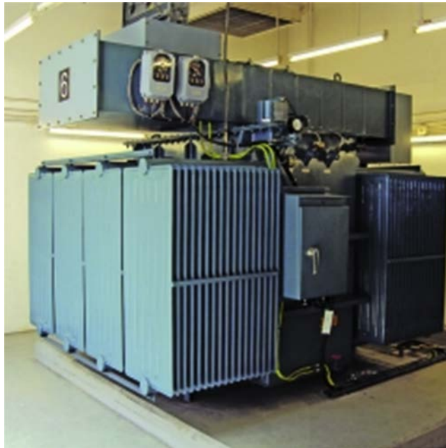
FIGURE 2.16.4 Oil-filled transformer.
