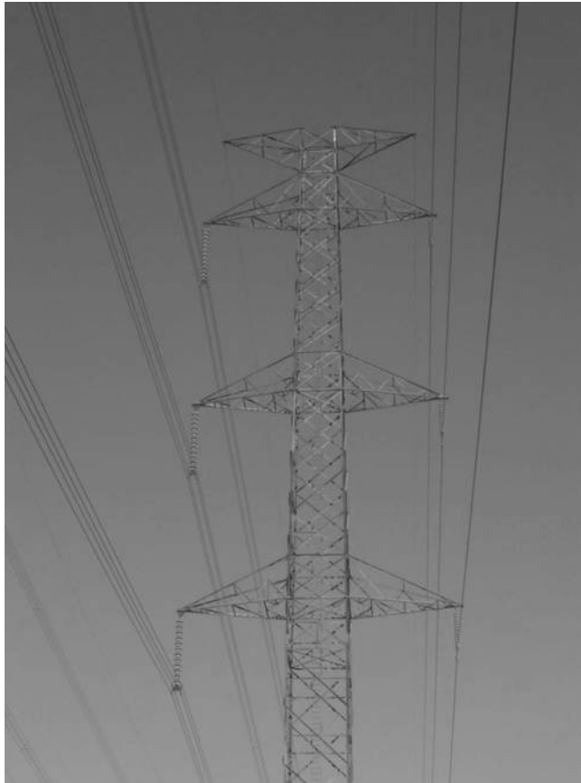
FIGURE 1.9 Typical high-power transmission line and tower.
