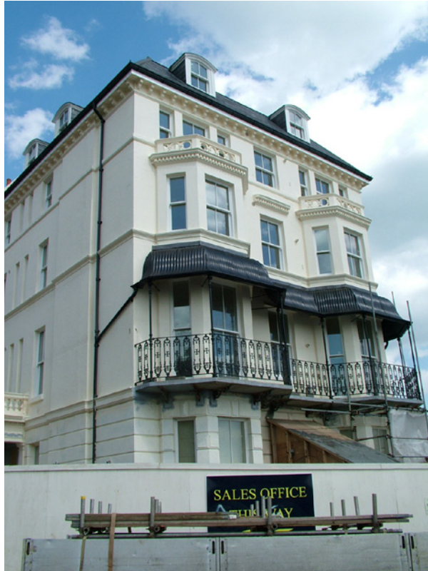
Figure 2.5 Marine Crescent, Folkestone. Reproduced by permission of The Concrete Centre.
