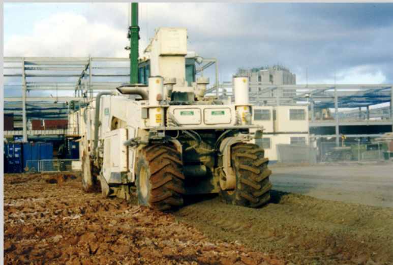
Figure 3.18 In-situ treatment of the site; The plant doses the soil with binder and then rotovates the soil immediately, thereby minimising dust levels. Courtesy of O'Keefe Soil Remediation.
