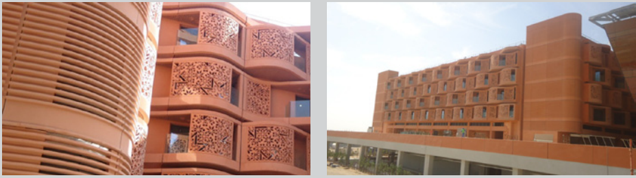
Figure 3.1 Masdar Institute Campus; Building (right) – Close up on the glass-reinforced concrete façade (left). Reproduced by permission of Gavrilis Ioannou.
