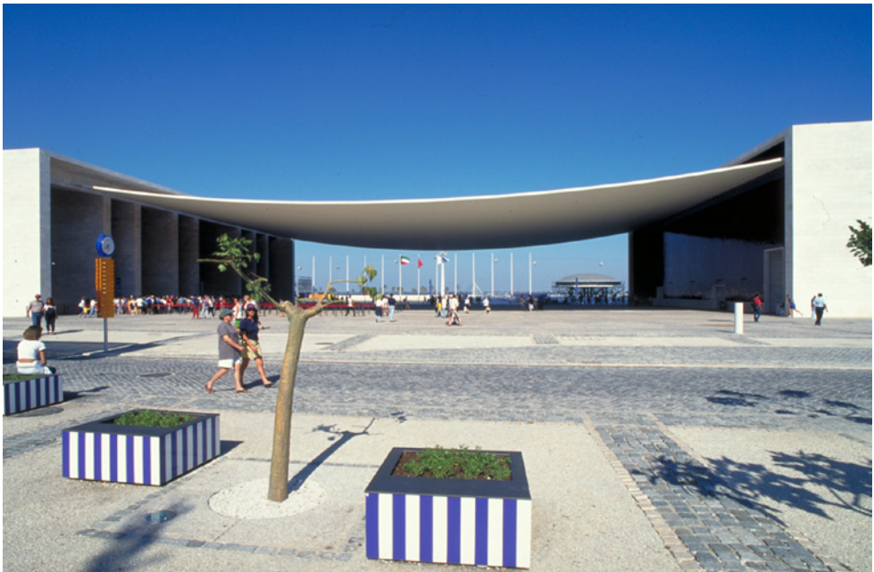
Figure 3.14 Portuguese National Pavilion, Lisbon Portugal; 200mm thick lightweight concrete ( 18\text{kN/m}^3 ) roof. Reproduced by permission of Arup.
