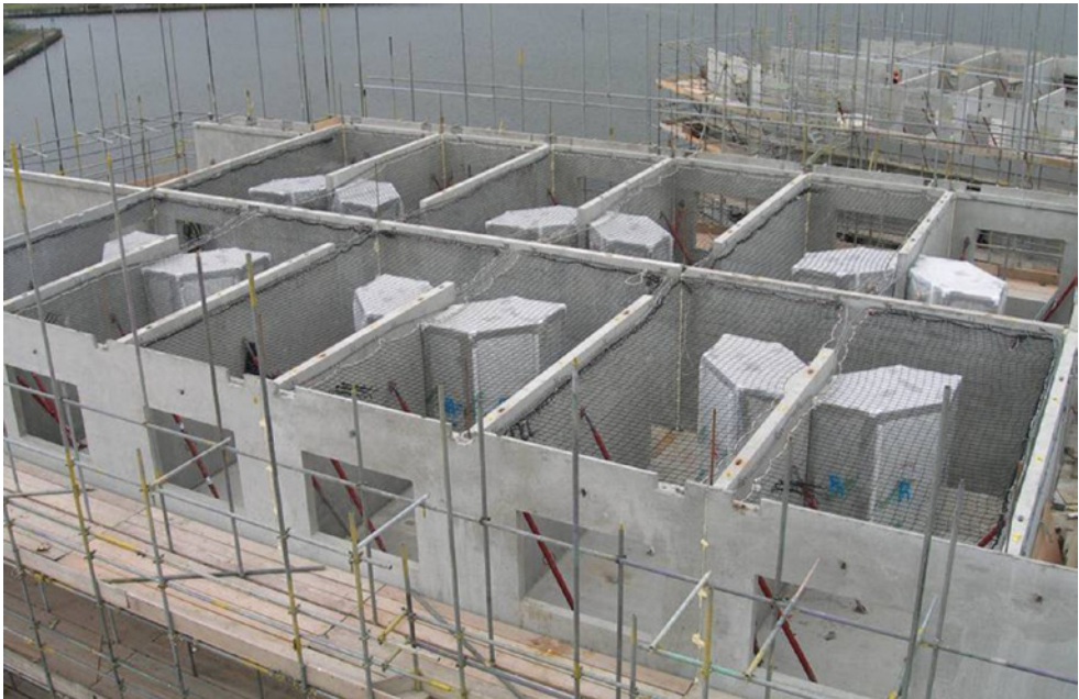
Figure 3.5 University of East London, UK; Multi-functional walls for student accommodation.
