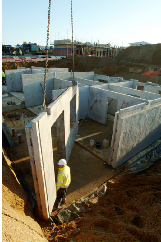
Figure 3.9 Martin Grant Homes, Cambridge, UK; basement construction. Reproduced by permission of The Basement Information Centre.
