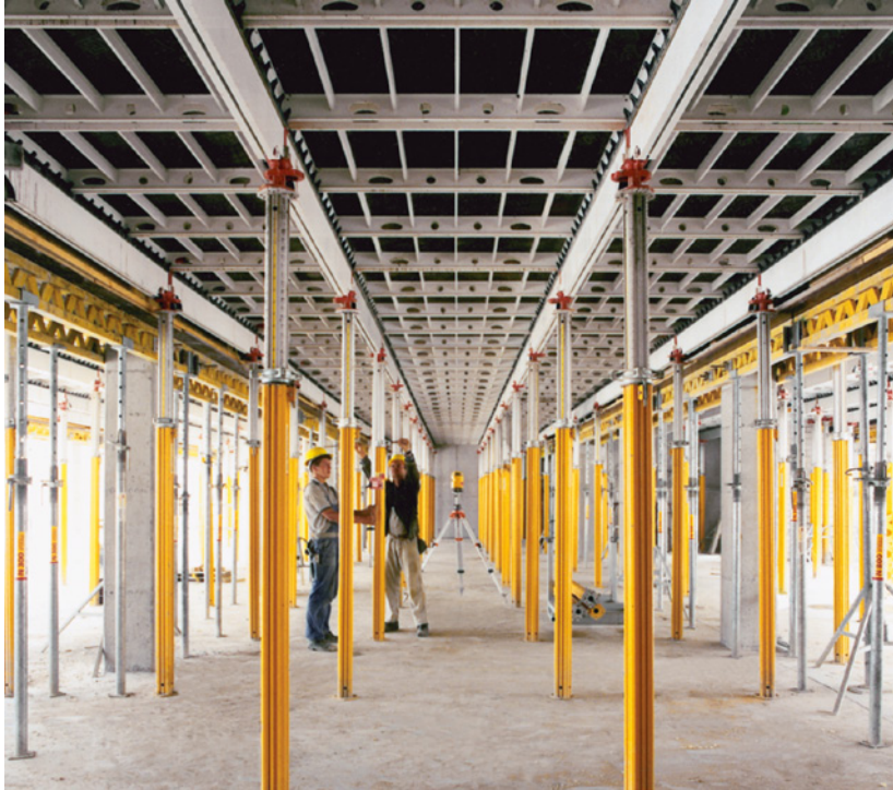
Figure 5.2 SKYDECK aluminium panel slab formwork. Reproduced by permission of PERI.
