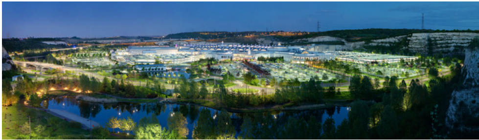
Figure 2.6 Bluewater shopping centre built on an old chalk quarry (before and after), Kent. Reproduced by permission of Gordon Edgar. Photo by DAVID ILIFF. License: CC-BY-SA 3.0.
