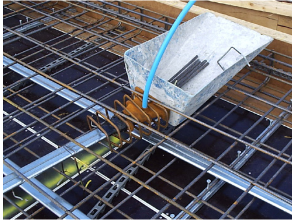
Figure C.7 Stressing pan to provide top access to post-tensioning strands. Reproduced by permission of Kevin Bennett.
