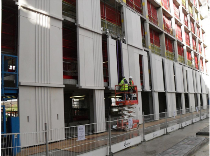
Figure 3.13 Olympic Village, London, UK; Precast concrete cladding was chosen for its long service life. Reproduced by permission of The Concrete Centre.
