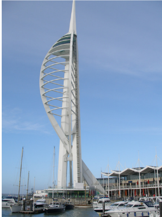
Figure 2.2 Spinnaker Tower, Portsmouth.
