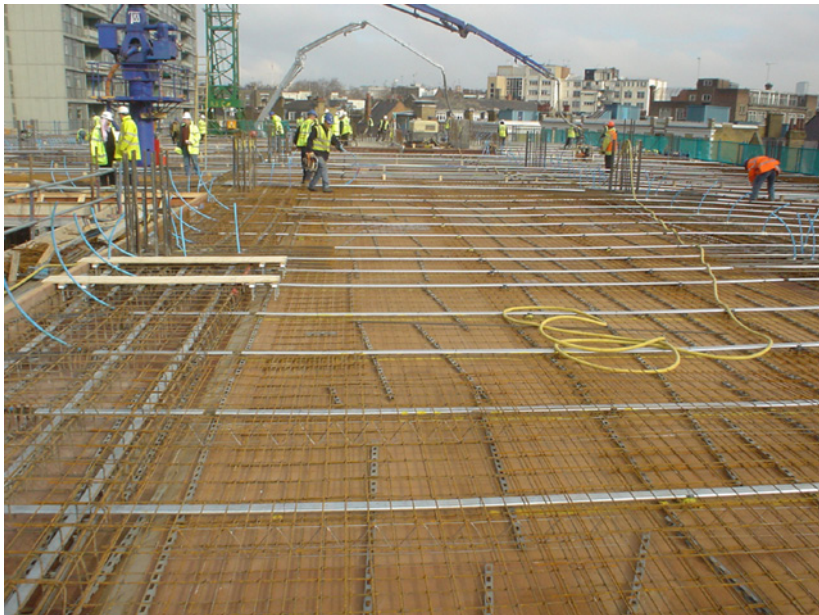
Figure C.6 A bonded PT slab just prior to concreting being placed. Reproduced by permission of The Concrete Centre.
