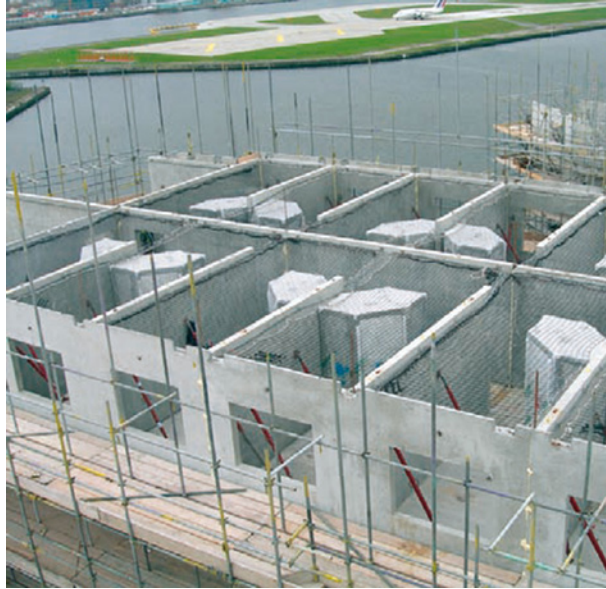
Figure C.10 Crosswall construction – University of East London. Reproduced by permission of The Concrete Centre.
