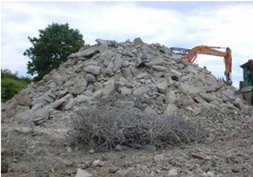
Figure 4.11 Separation of reinforcement and concrete following demolition and prior to RCA processing.
