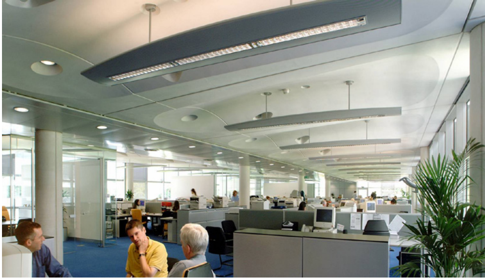
Figure 3.4 Toyota Office, Surrey, UK; Exposed soffits for thermal mass. Reproduced by permission of The Concrete Centre.
