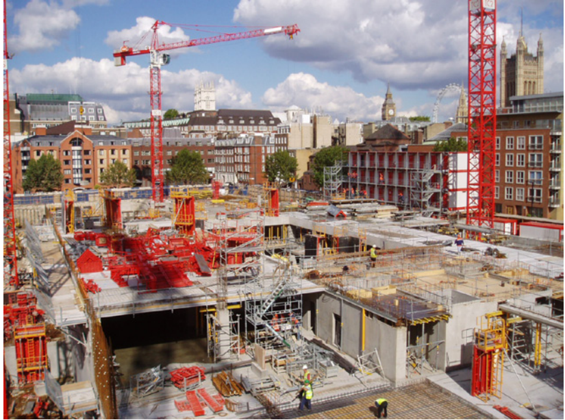
Figure C.9 The Home Office Project used precast elements as shown in option 5 of Figure C8 plus precast columns. Reproduced by permission of The Concrete Centre.
