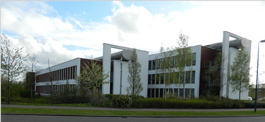
Figure 3.8 Innovate Green Office, Leeds, UK; An outstanding BREEAM rated speculative office comprises two parallel wings joined by a longitudinal atrium. Reproduced by permission of The Concrete Centre.
