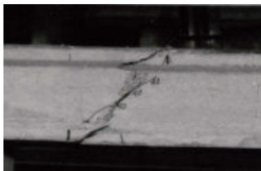
Fig. 9.3 Web crushing failure
