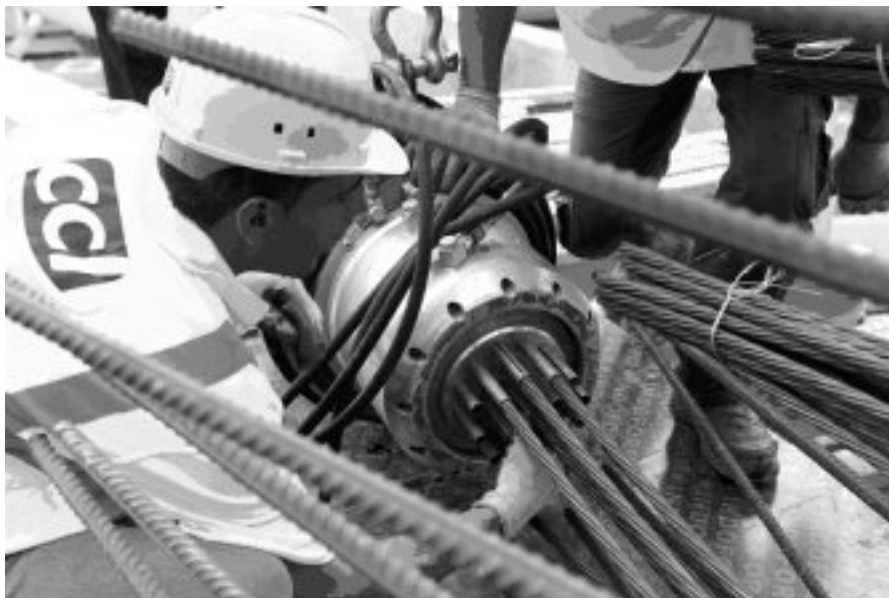
Fig. 2.19 Stressing the cable Photo Courtesy CCL
