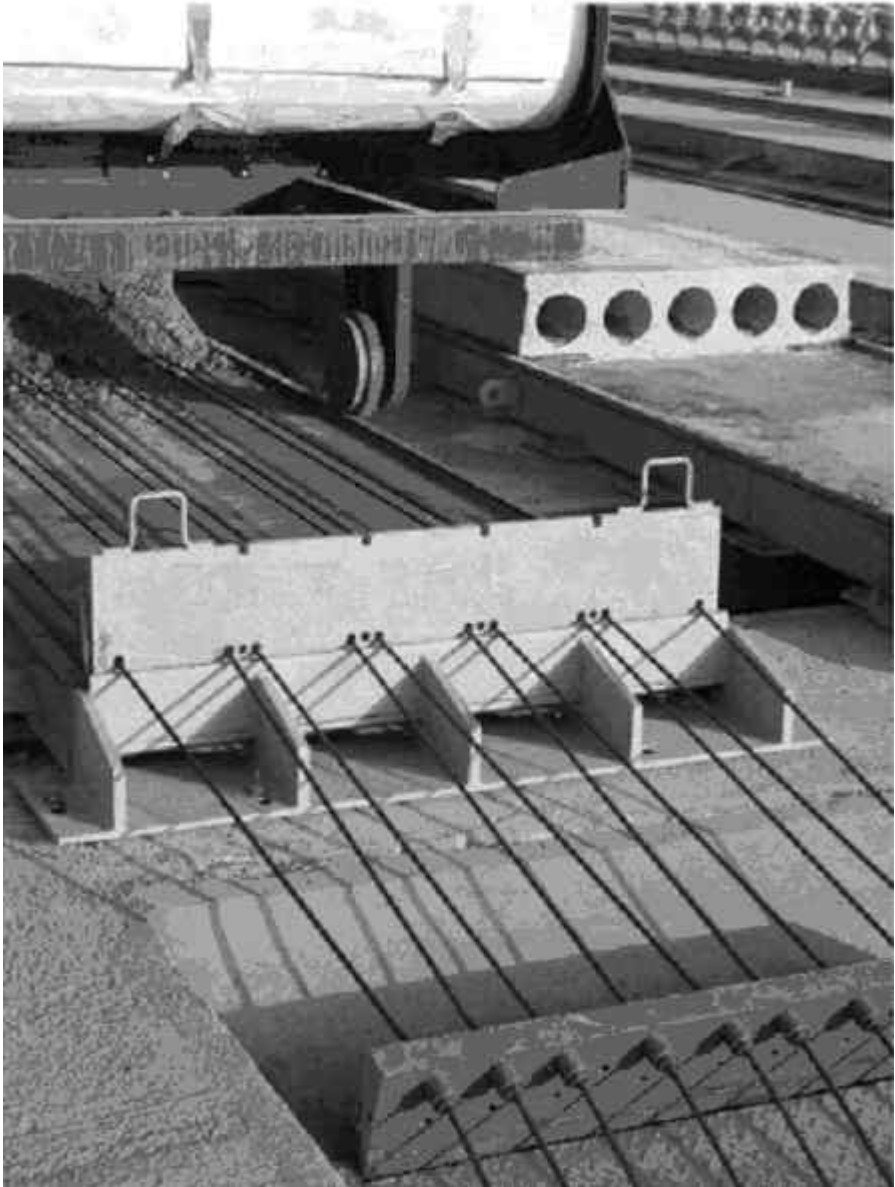
Fig. 2.2b Placing concrete after pre-tensioning the cables
