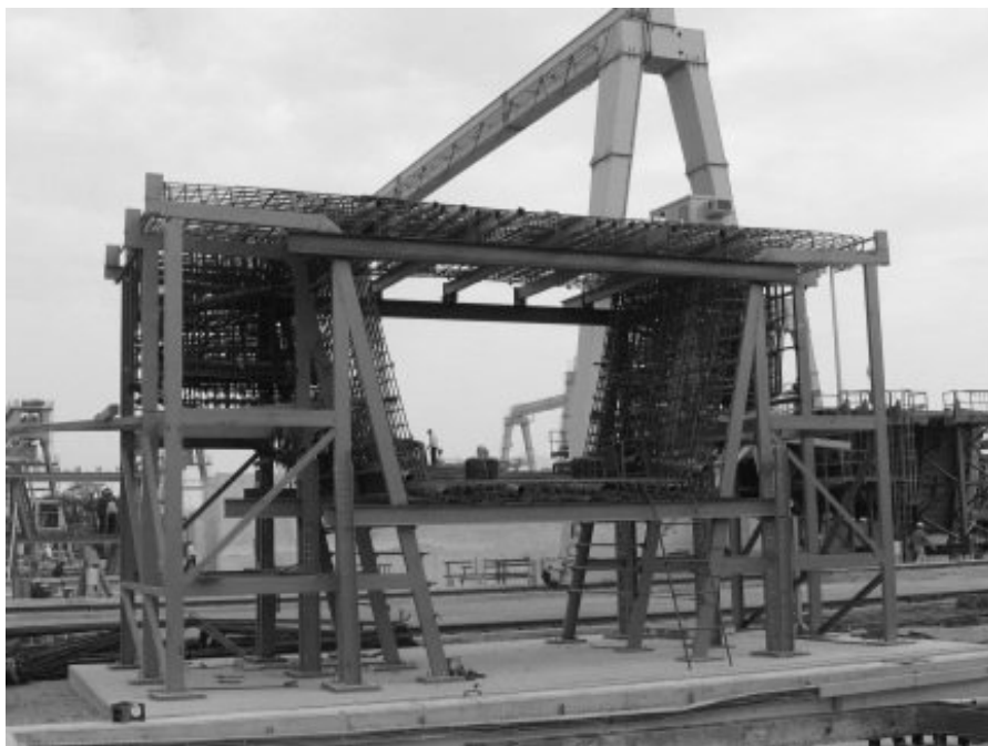
Fig. 16.7 Reinforcement for a segment Photo: Courtesy of CCL Ltd
