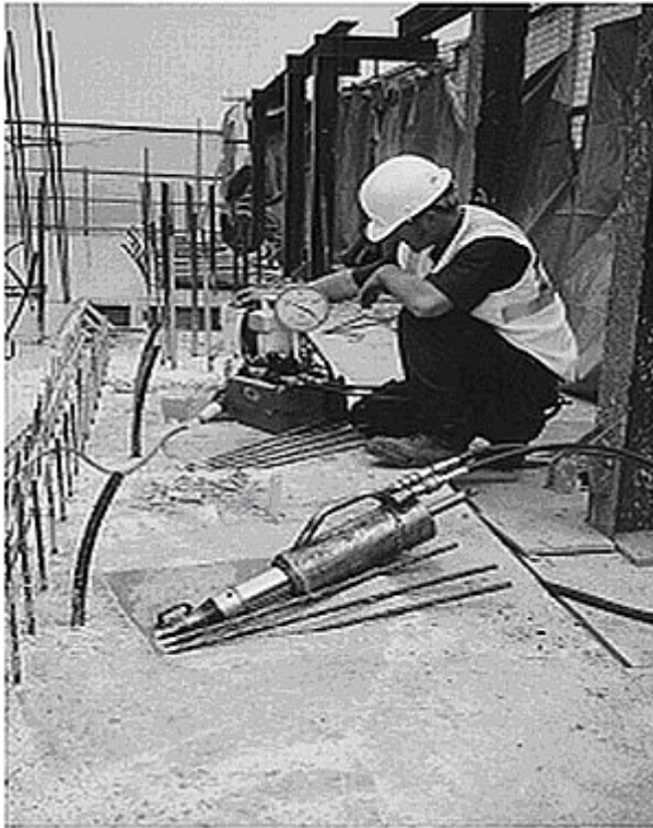
Fig. 12.91 Stressing the cables Photo Courtesy VSL
