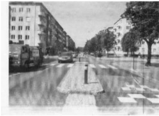
Malmö: After, speed limit: 40 km/h. New section
