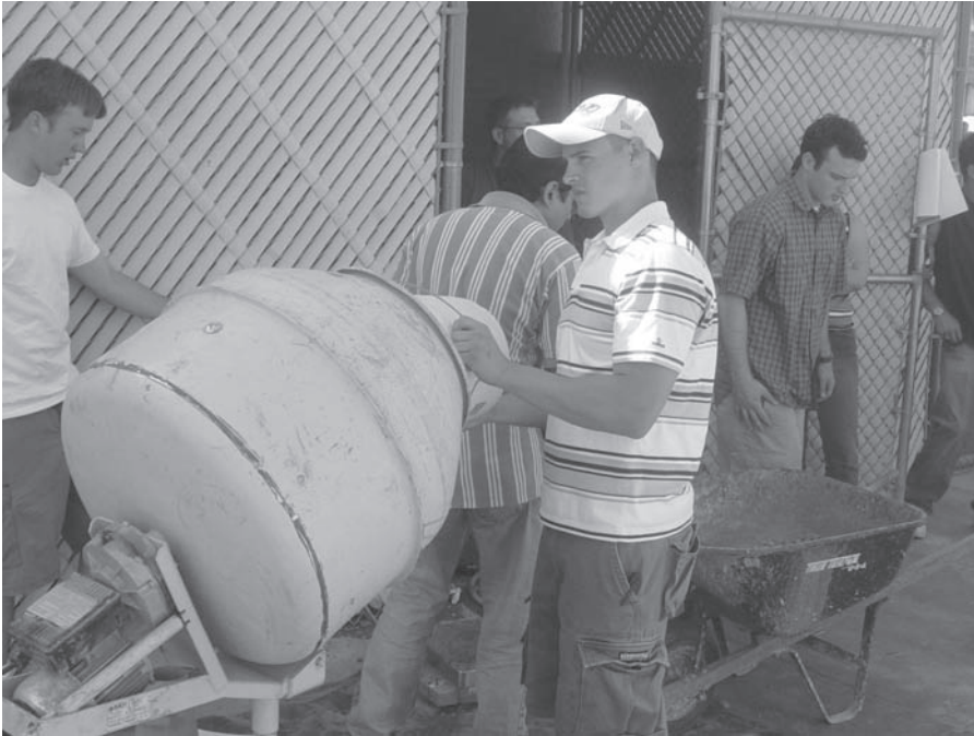
FIGURE A.30 Mixing concrete in a mixer.
