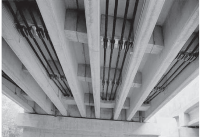
FIGURE 11.13 Strengthening a concrete bridge with FRP composite bars.
