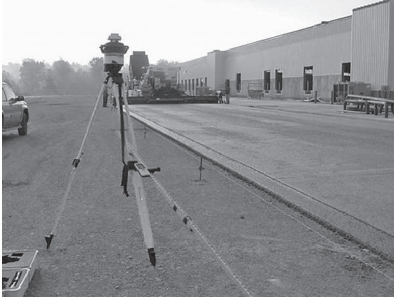
FIGURE 7.52 Placing roller compacted concrete with a vibratory screed. (Courtesy of A.G. Peltz Group, LLC)
