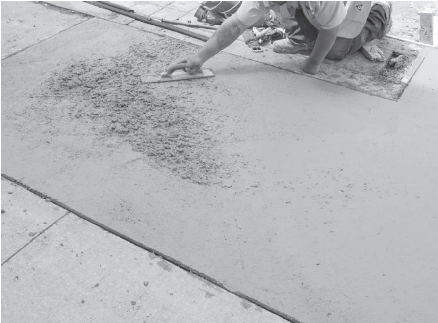
FIGURE 7.18 Finishing concrete with a trowel. (Fotolia/alisonhancock)
