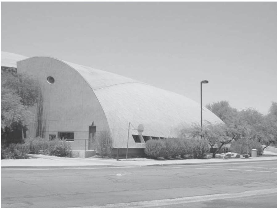
FIGURE 4.2 Building facade made of aluminum.
