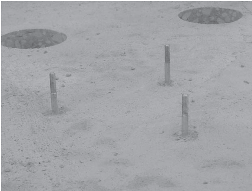
FIGURE A.49 Three probes driven into concrete.
