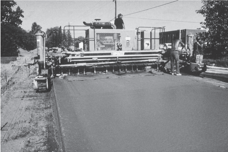
FIGURE 7.10 Placing concrete pavement with a slip-form paver.
