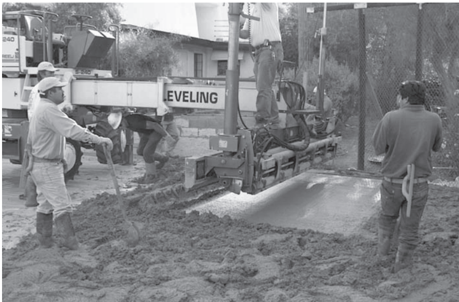
FIGURE 7.23 Using laser level to establish elevation for finishing concrete. (Courtesy of FHWA)
