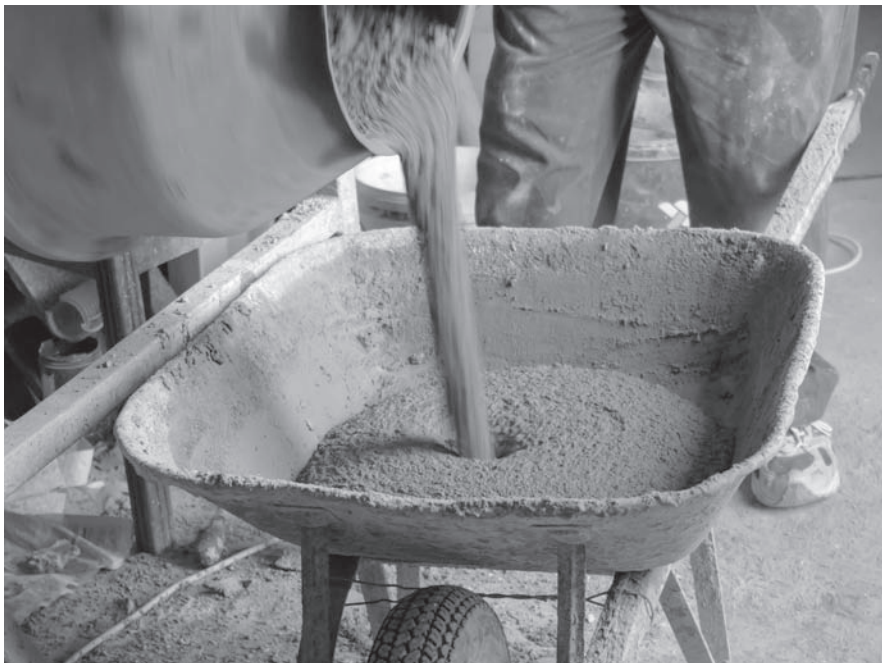
FIGURE 7.7 Loading concrete in a wheelbarrow. (Fotolia/Laure F)
