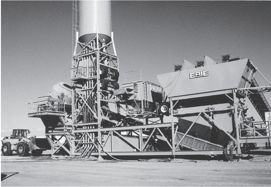
FIGURE 7.6 Mobile batcher mixer at the job site.
