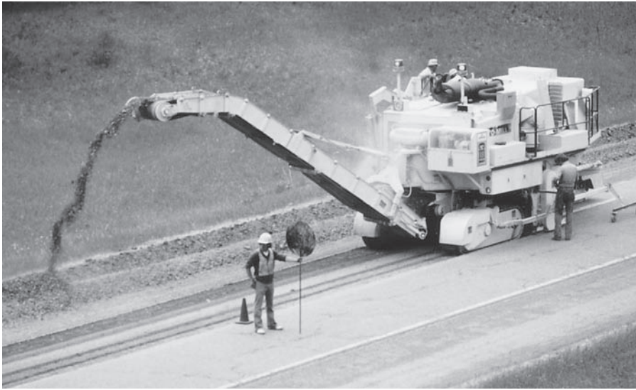
FIGURE 9.41 Milling old pavement.
