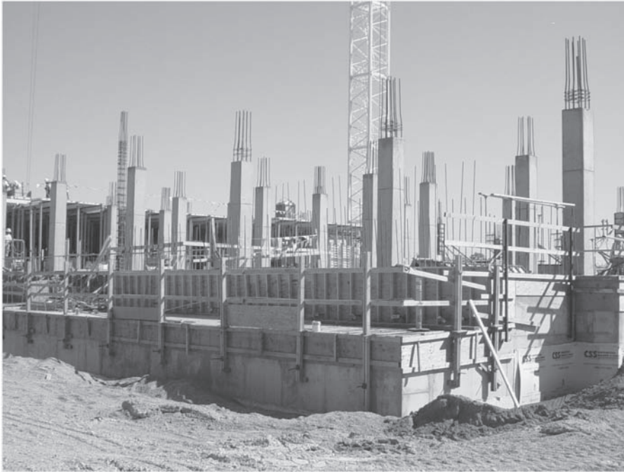
FIGURE 3.13 Steel rebars used to reinforce PCC columns.
