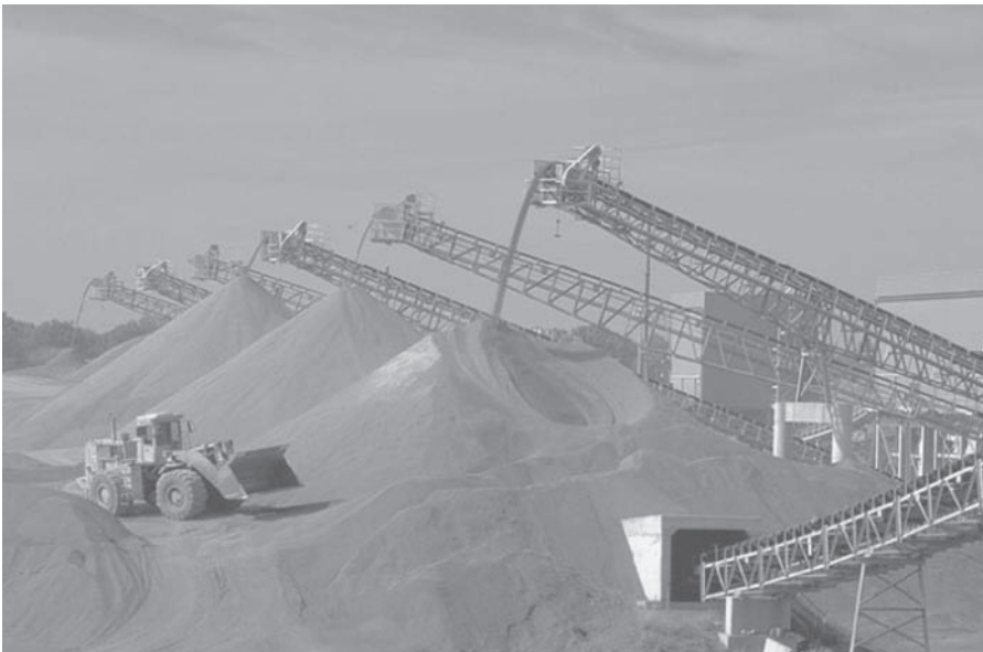
FIGURE 5.1 Aggregate stockpiling. (Courtesy of FHWA)
