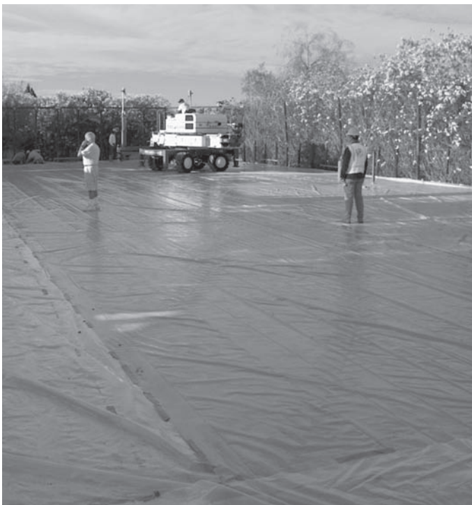
FIGURE 7.29 Curing concrete with plastic sheets.
