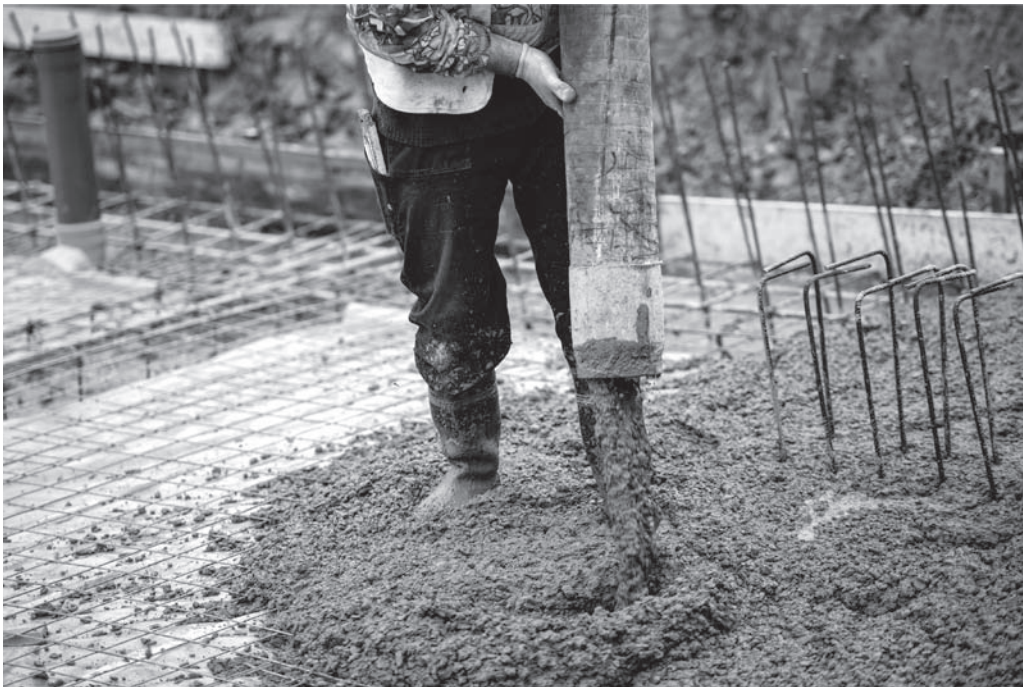
FIGURE 7.9 Placing concrete with Chute. (Fotolia/Hoda Bogdan)
