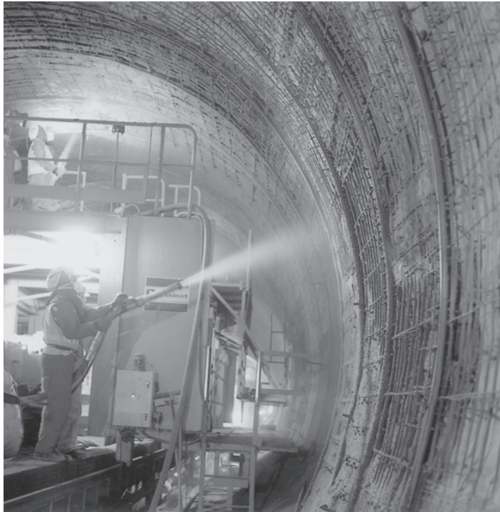
FIGURE 7.47 Shotcrete used in lining a tunnel. (Courtesy of the American Shotcrete Association)
