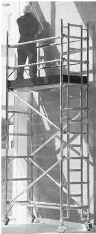
Figure 2.24 Mobile scaffold tower
