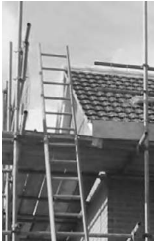
Figure 2.19 Safely lashed ladder
