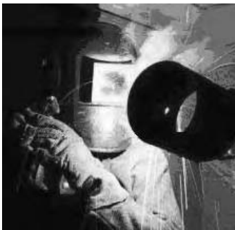
Figure 12.3 Welding of a large diameter pipe
