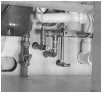
Figure 5.6 Internal stop valve
