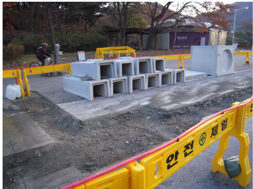
Fig. 11.4 Cutting work of selected road
