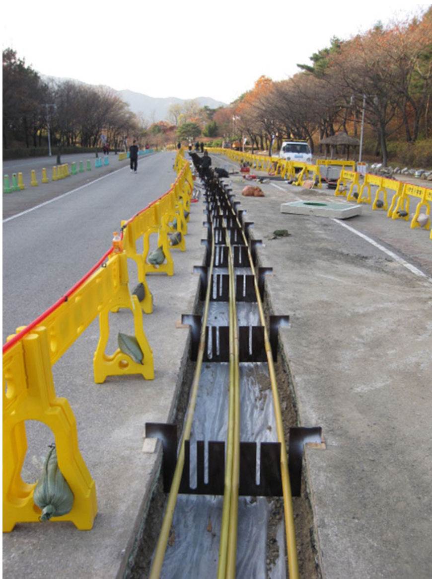
Fig. 11.6 Structure prepared to install power supply system
