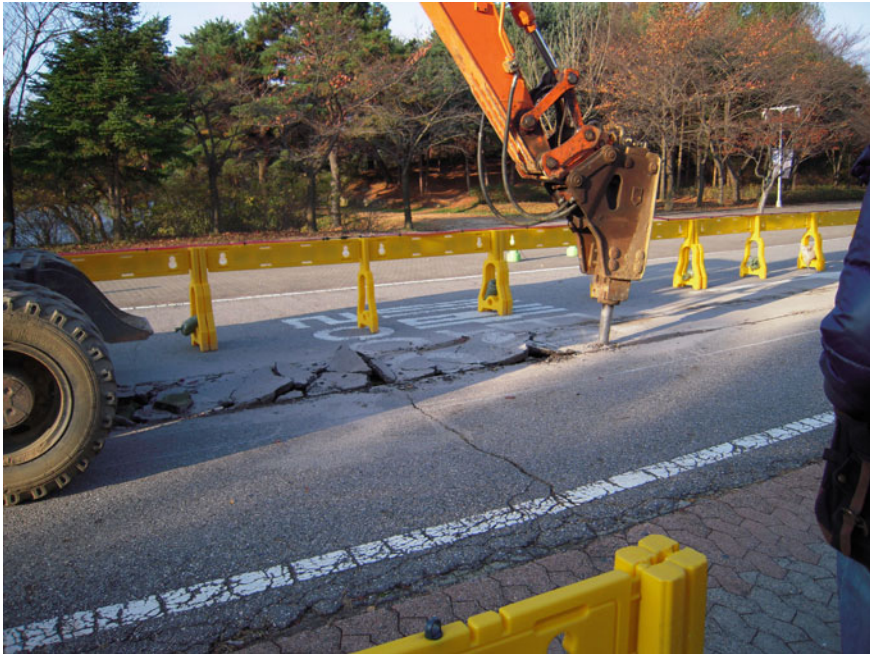
Fig. 11.5 Process for excavating existing road
