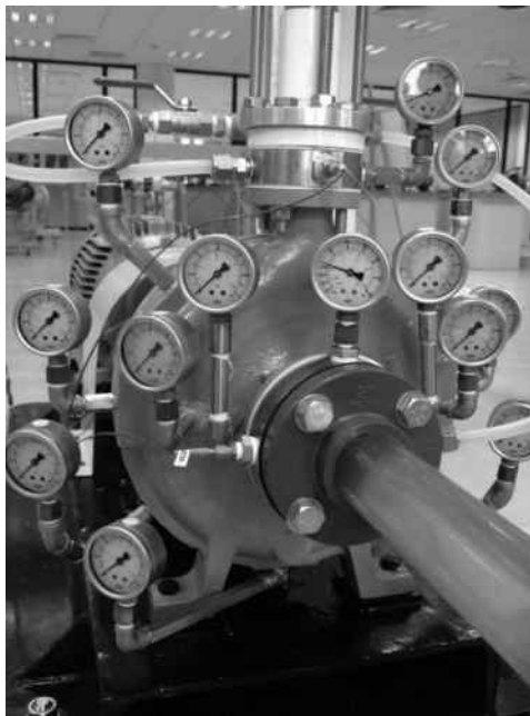
FIGURE 5.10 Pressure Gauges on a Centrifugal Pump (Photo from C.J. Schaschke.)
