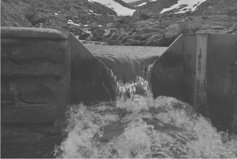
FIGURE 6.1 Triangular Notch (Photo by C.J. Schaschke.)
