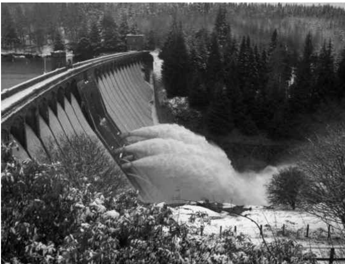
FIGURE 3.2 Open Discharge of Laggan Dam, Scotland (Photo from C.J. Schaschke.)
