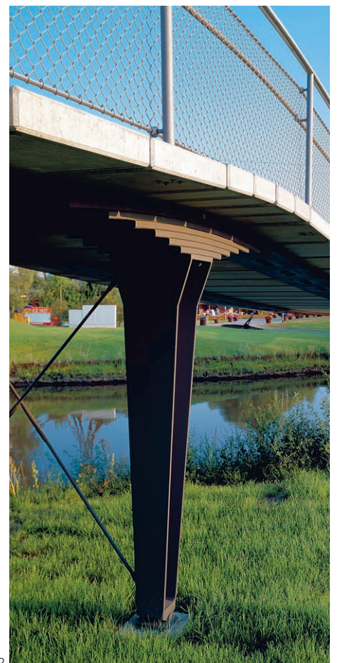
62 Haunch of a stress ribbon bridge with leaf spring 62
