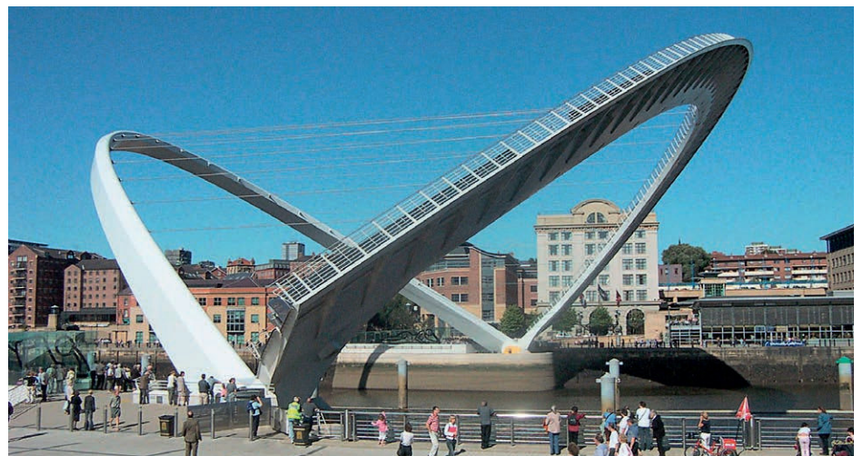
1 Turn and tilt bridge, Gateshead Millennium Bridge, Newcastle (GB) 2001, Wilkinson Eyre Architects; Gifford & Partners
