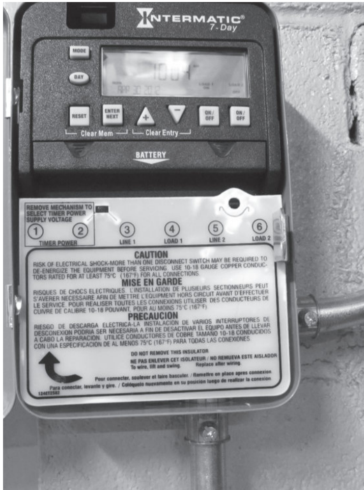
FIGURE 10-9 Synchronous clock timer.
