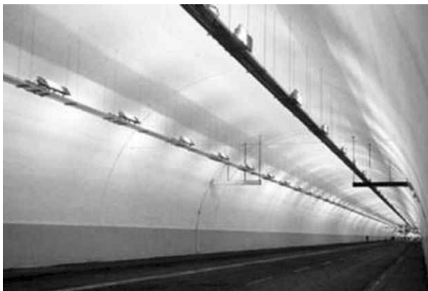
15.2 Umberto I tunnel in Rome.
