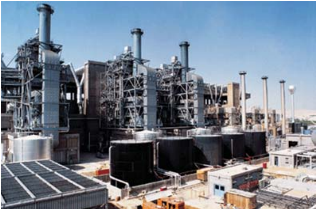
An overview of a thermal power station.
