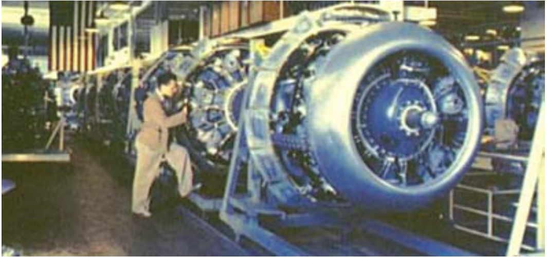
Aircraft engine is being assembled.
