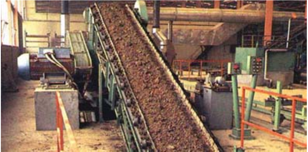
Material being moved via-belt conveyor.
