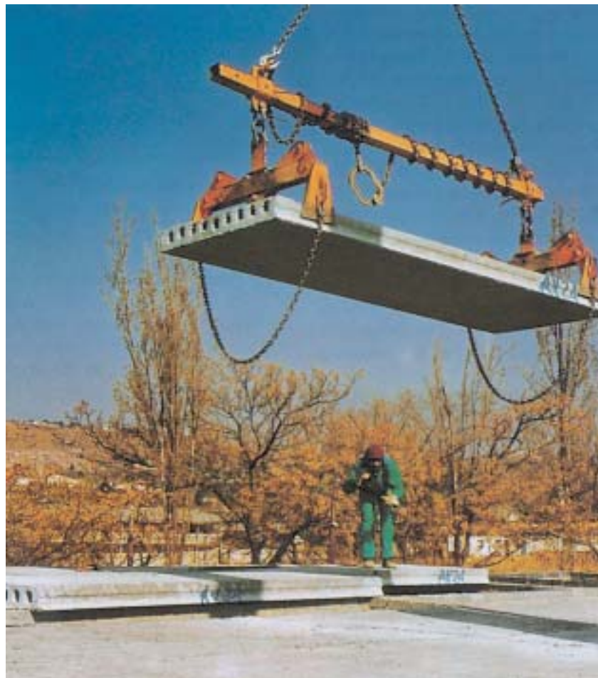
Fig 3: Hollow core slab being hoisted into position
