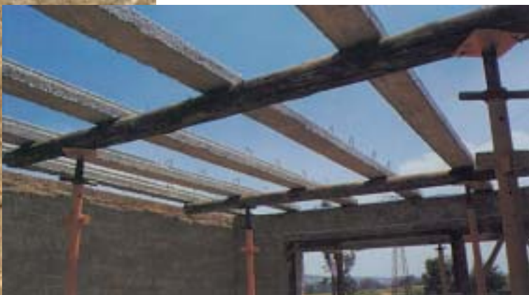
Figure 20: Prestressed beams in place with support.
