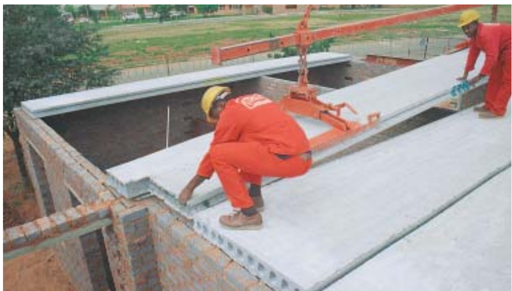
Figure 18: Erection of hollow core slab on masonry structure
