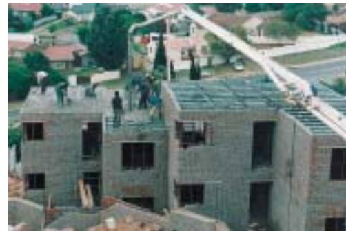
Figure 24: Casting concrete topping to beam and block slabs.
