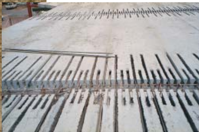
Figure 27 and 28: Tops of cores in hollow core slab opened up for reinforcement to form moment connection with beam.
