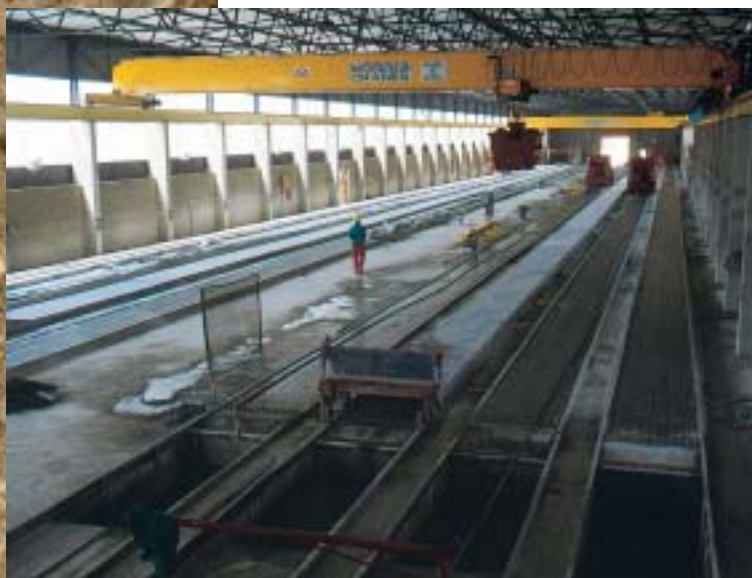
Figure 8: Manufacturing facility for prestressed hollow core slabs.
