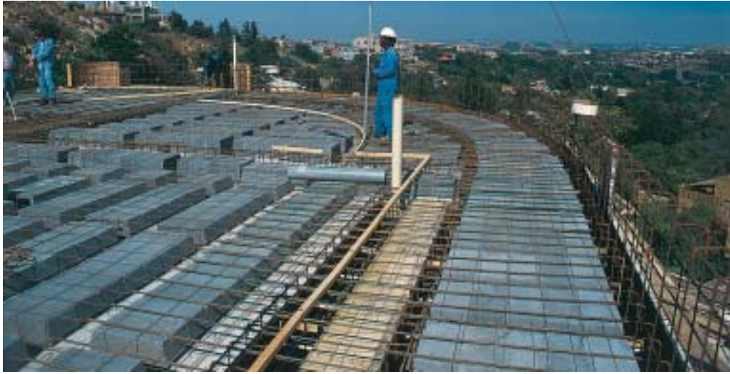
Figure 4: Beam and block slab on irregular-shaped building
