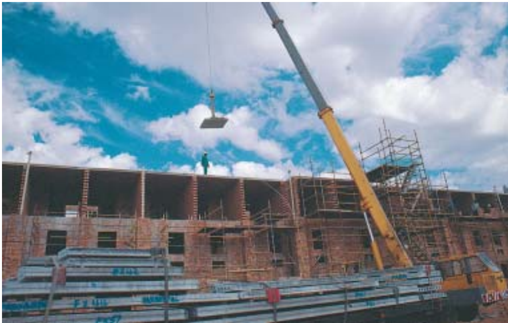
Figure 14: Hollow core slab for an hotel
