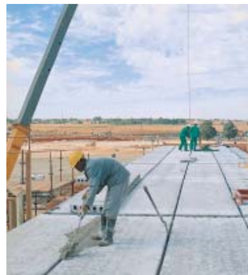
Figure 33: Grouting joint between hollow core slabs.
