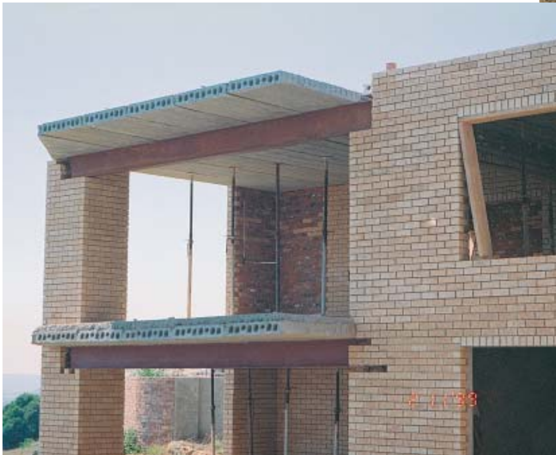
Figure 30 and 31: Steel beams used over large openings
