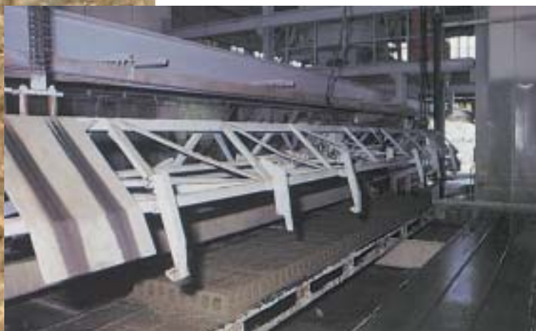
Figure 9: Manufacture of reinforced hollow core slabs.
