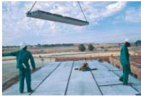
Figure 1: Erection of hollow core slabs
