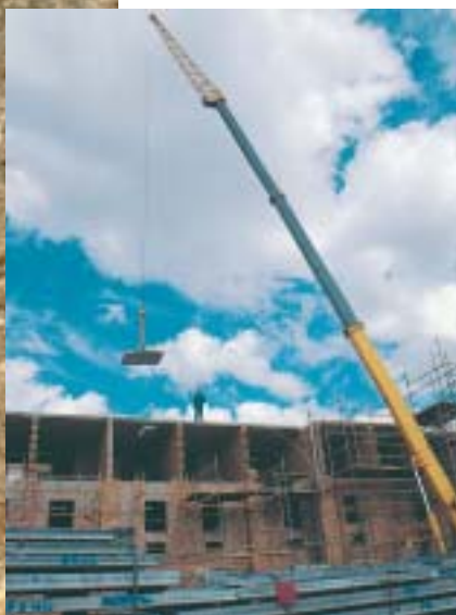
Figure 34 & 35: Hoisting slabs into position.
