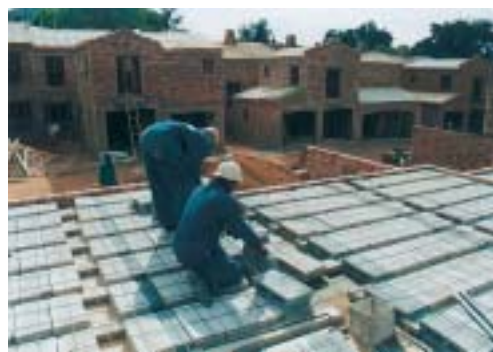
Figure 38: Mesh placed over blocks.
