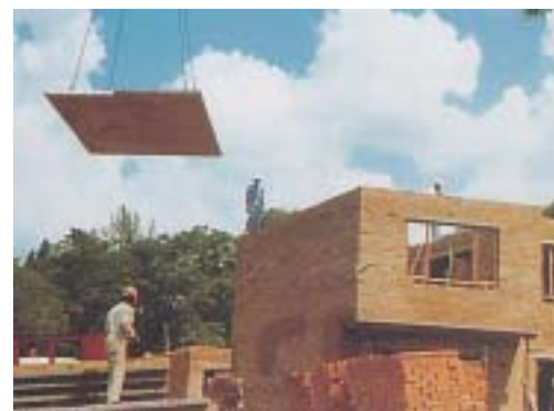
Figure 25: Wide panel being hoisted into position.
