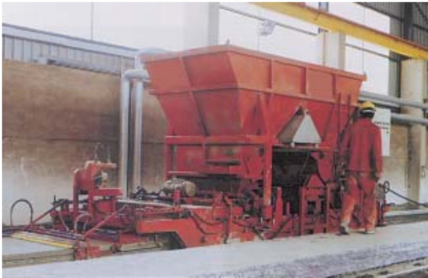
Figure 10: Manufacturing hollow core slabs.
