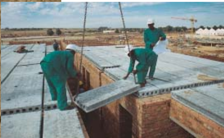
Figure 32: Placing of hollow core slabs directly onto masonry.
