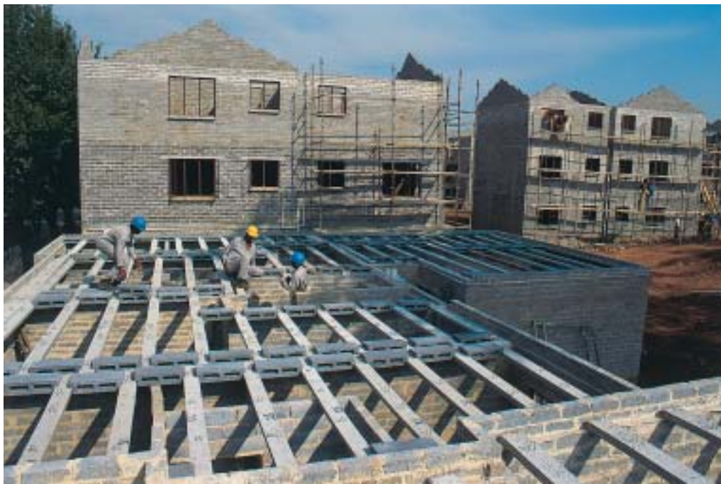
Figure 2: Prestressed beam and block slab under construction
