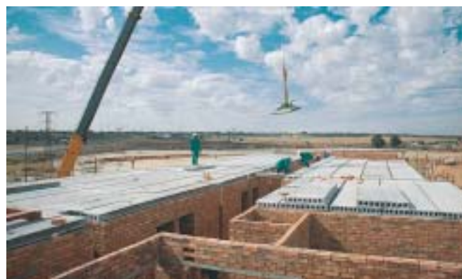
Figure 34 & 35: Hoisting slabs into position.
