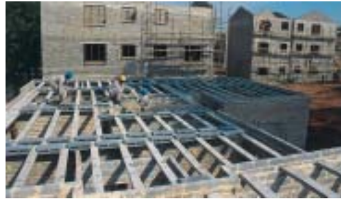
Figure 36: Setting out of beams.
