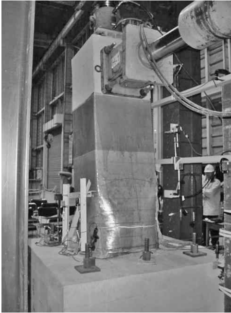
5.15 Typical failure of RC piers jacketed with LRS FRP composites within the hinge zone at the ultimate state.
