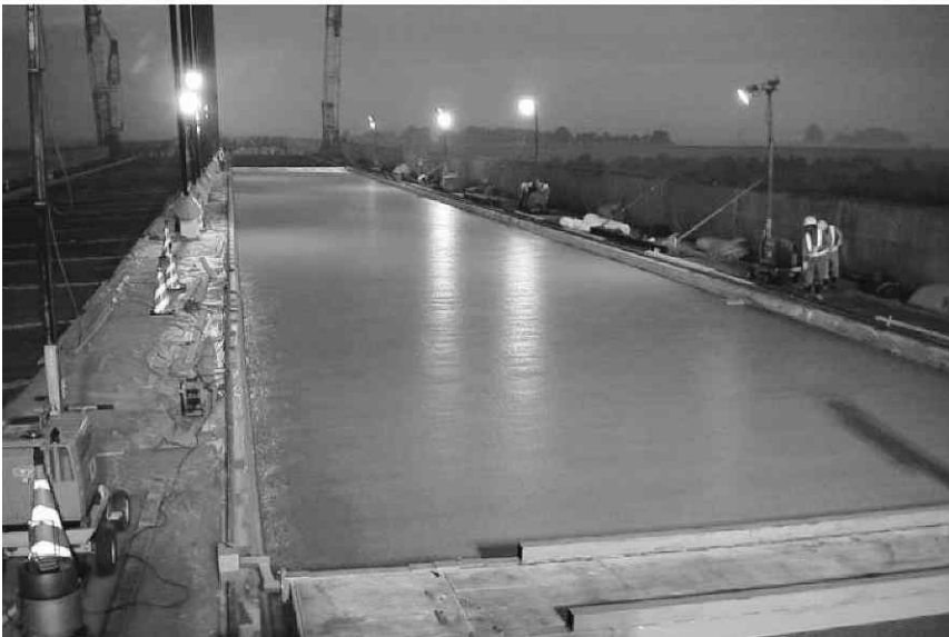
7.24 Mihara Bridge in Hokkaido, Japan, courtesy of Dr Tetsu Kanda. 77
