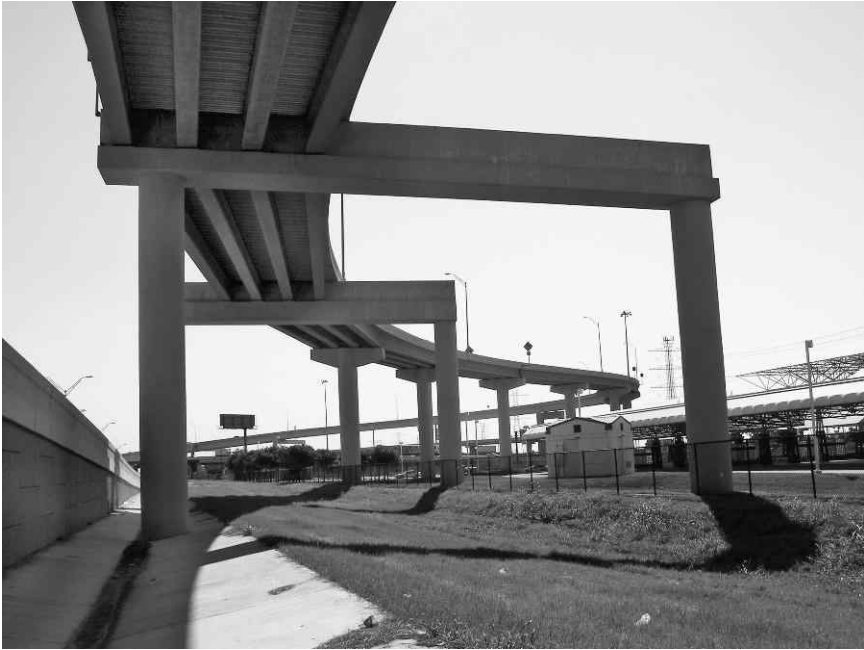
9.1 Overview of bridge and two substructure straddle bents.
