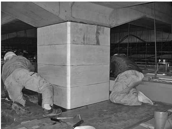
5.16 Seismic retrofit of a railway bridge pier using PET FRP composites.
