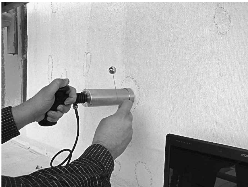
9.17 Impulse response testing to identify extent of CFRP delaminations.
