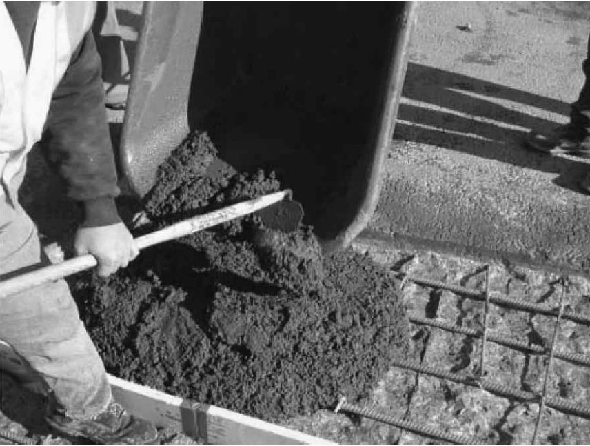
7.19 Placement of Thoroc 10-60. 16
