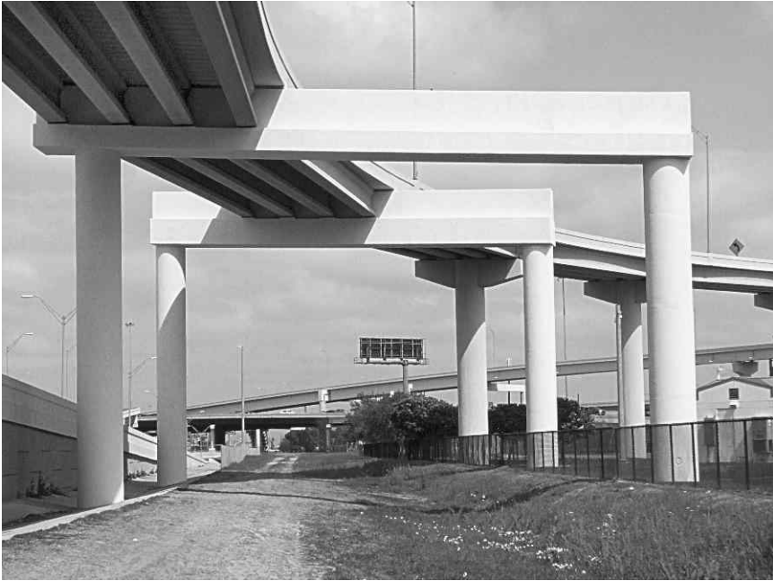
9.19 Overview of straddle bents after repair.
