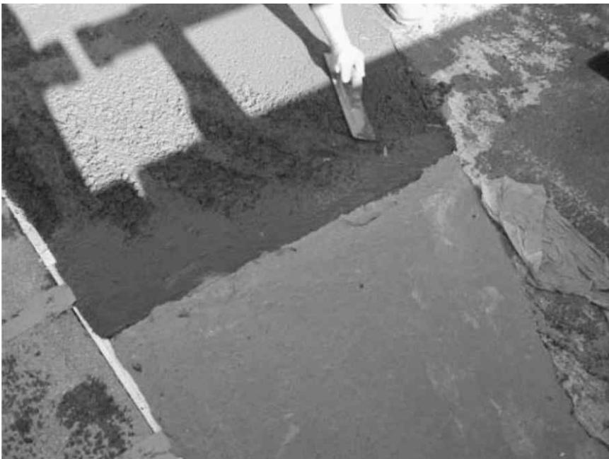
7.20 HES-ECC and Thoroc 10-60 patch repairs side by side. 16
