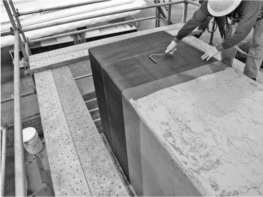
9.11 Application of CFRP composite U-wrap to the straddle bent beam end.
