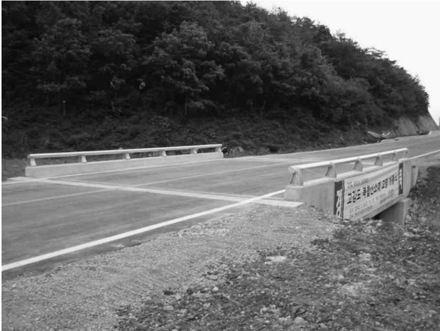
6.11 Completed FRP bridge.
