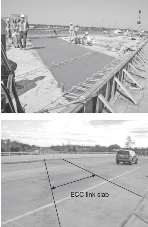
7.23 ECC link slab in Michigan to replace bridge expansion joints. 75
