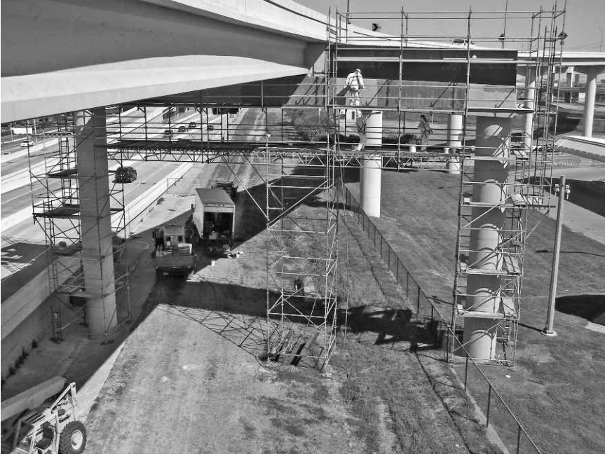
9.14 Overview of CFRP composite application to straddle bent beam.
