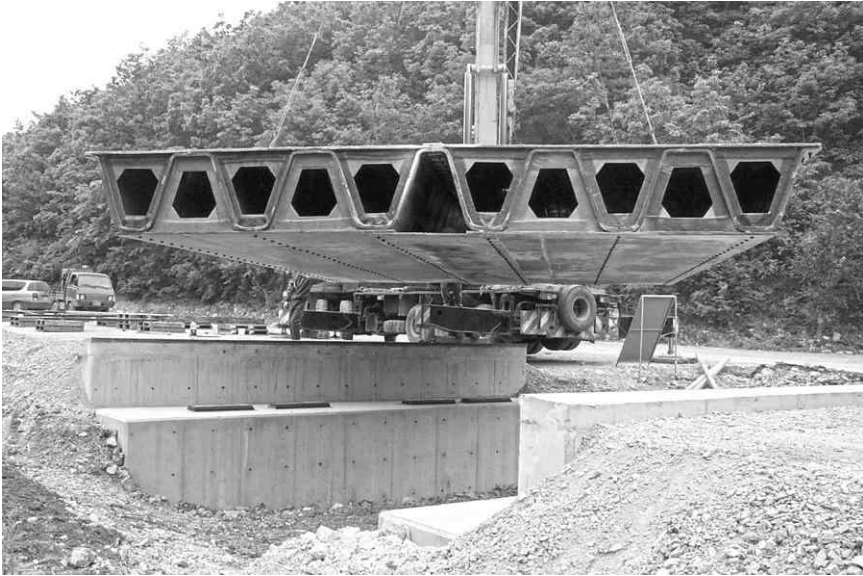
6.10 The entire FRP superstructure.
