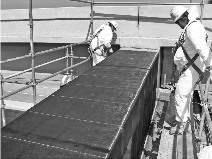
9.12 Application of CFRP composite U-wrap along straddle bent beam.
