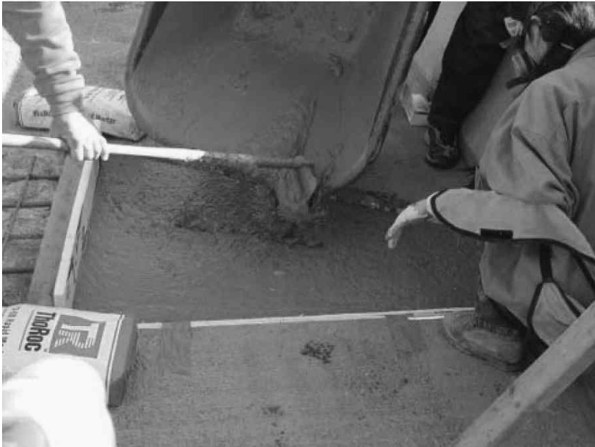
7.18 Placement of self-compacting HES-ECC. 16
