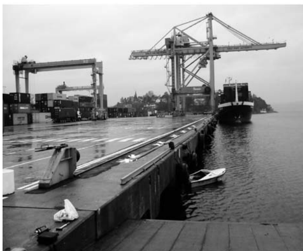
Figure 3.5.10 Ormsund quay—as seen from below at right.
