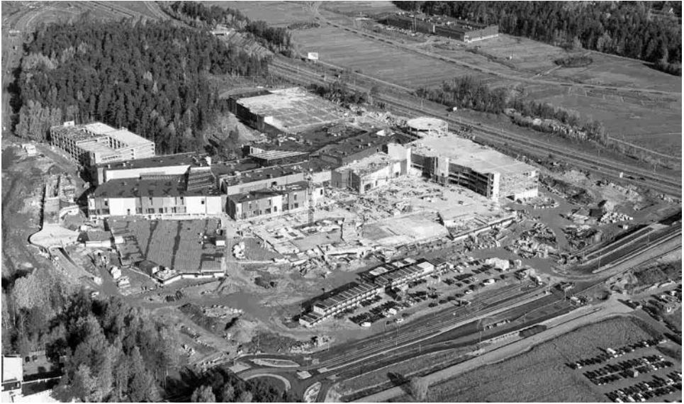
Figure 17.8 Skanssi retail centre—in construction
