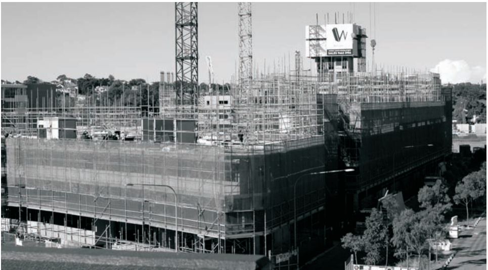
Figure 17.3 Victoria Park residential development—Form 302—in construction
