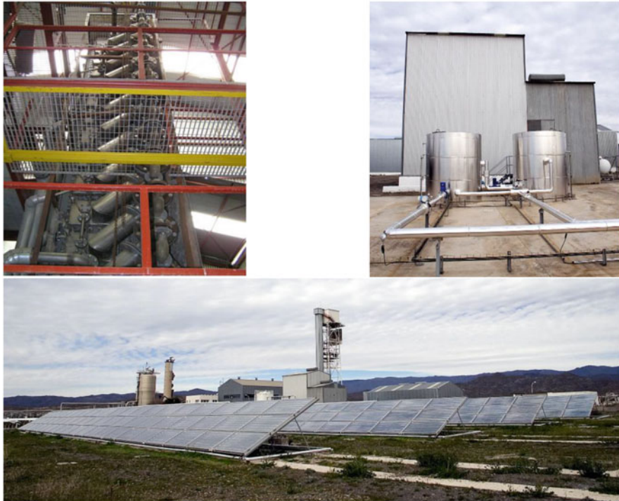
Fig. 1.8 Multi-effect distillation plant, storage system and compound parabolic collectors solar field at the Plataforma Solar de Almería
