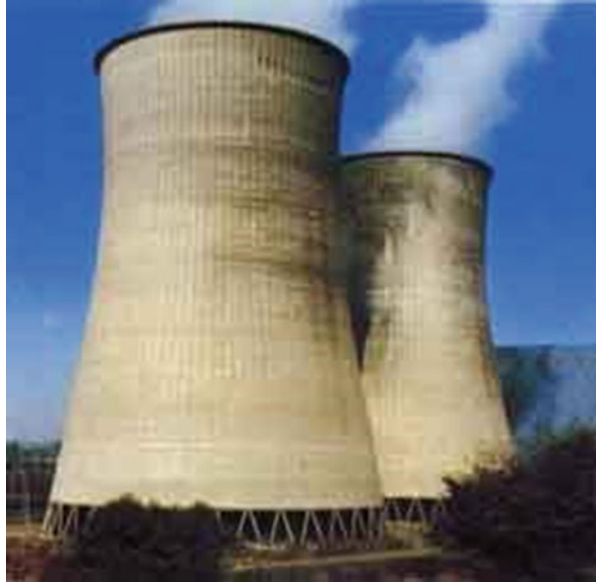
Fig. 2.17 Cooling towers in a CSP plant
