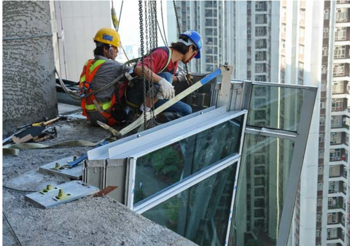
Figure 10. Cladding Elements Being Installed On Site by the Cladding Subcontractor (Courtesy of Gehry Technologies)
