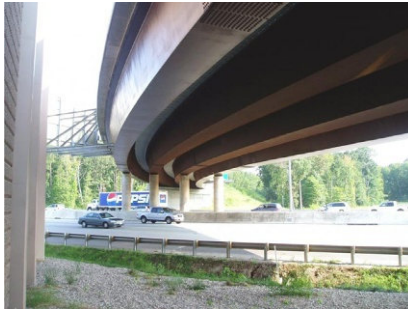
Figure 1.11 A box girder bridge ( alviassociates.com ).
