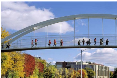
Figure 1.6 A pedestrian arch steel bridge ( photos.uc.wisc.edu ).
