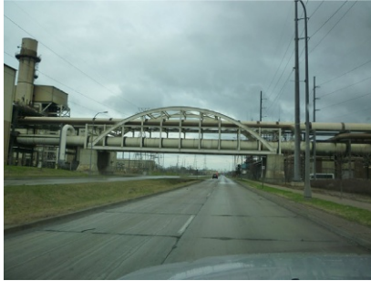
Figure 1.4 An arch steel bridge carrying pipelines ( civilenginphotos.blogspot.com ).
