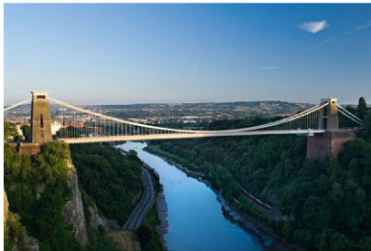
Figure 1.14 A suspension bridge ( ikbrunel.org.uk ).
