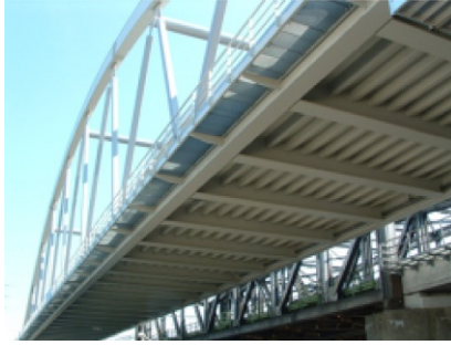
Figure 1.15 An orthotropic steel floor truss bridge ( steelconstruction.info ).
