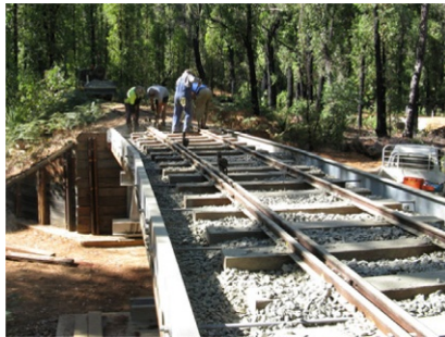
Figure 1.8 A ballasted floor bridge ( hothamvalleyrailway.com ).
