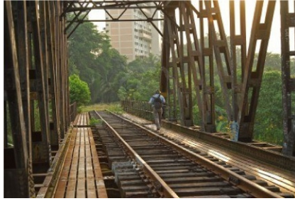
Figure 1.7 An open-timber floor bridge ( 123rf.com ).
