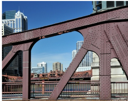
Figure 1.18 An old-fashioned riveted truss bridge ( pbase.com ).
