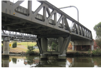
Figure 1.17 A pony truss bridge ( bphod.com ).
