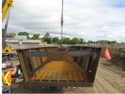
Figure 1.9 A steel-concrete composite box girder bridge under construction ( mto.gov.on.ca ).
