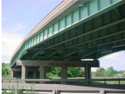
Figure 1.10 A multiplate girder bridge ( haks.net ).
