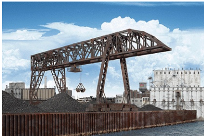
Figure 1.5 A crane truss steel bridge ( paperstreet.iobb.net ).
