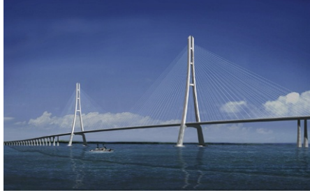
Figure 1.13 A cable-stayed bridge ( bridgemeister.com ).
