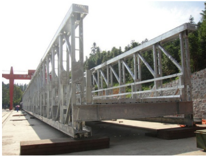
Figure 1.16 A semi-through truss bridge under construction ( steel-trussbridge.com ).
