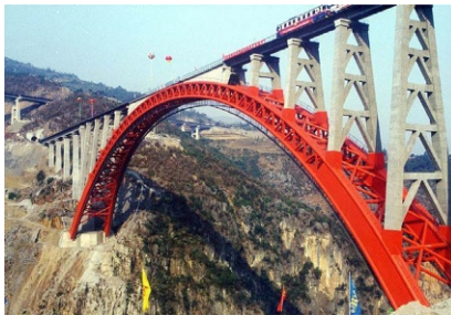
Figure 1.2 A railway arch steel bridge ( highestbridges.com ).
