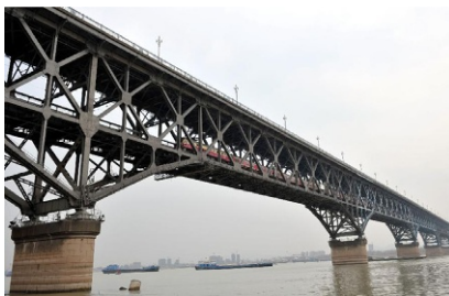
Figure 1.3 A combined highway-railway truss steel bridge ( chinatravelguide.com ).
