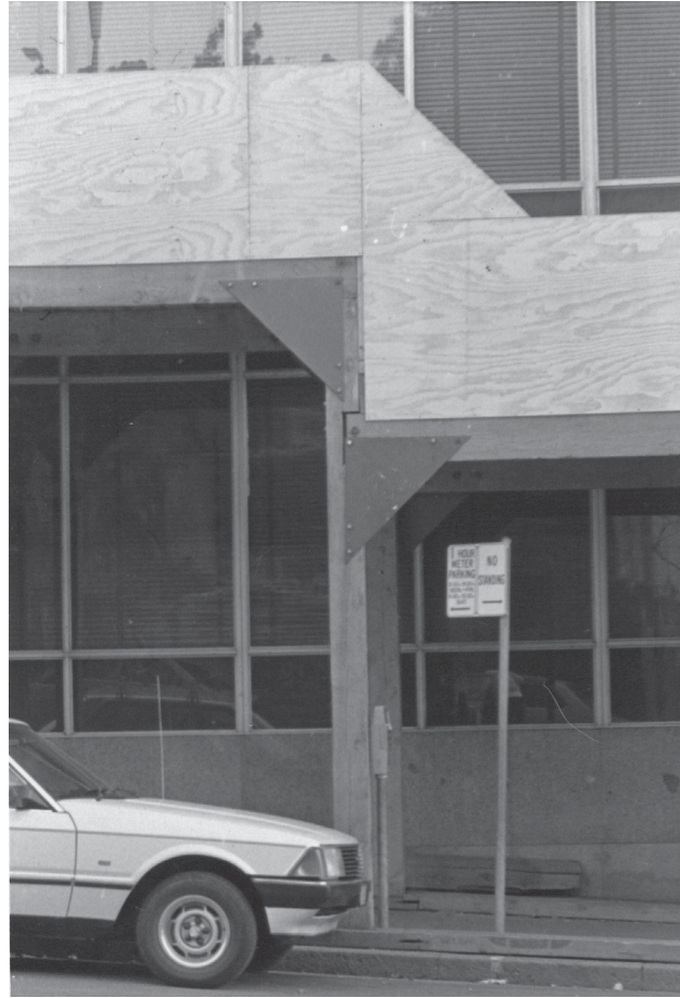
Large softwood posts and beams with waterproof plywood balustrade on a temporary footpath hoarding structure bolted together for ease of dismantling.
