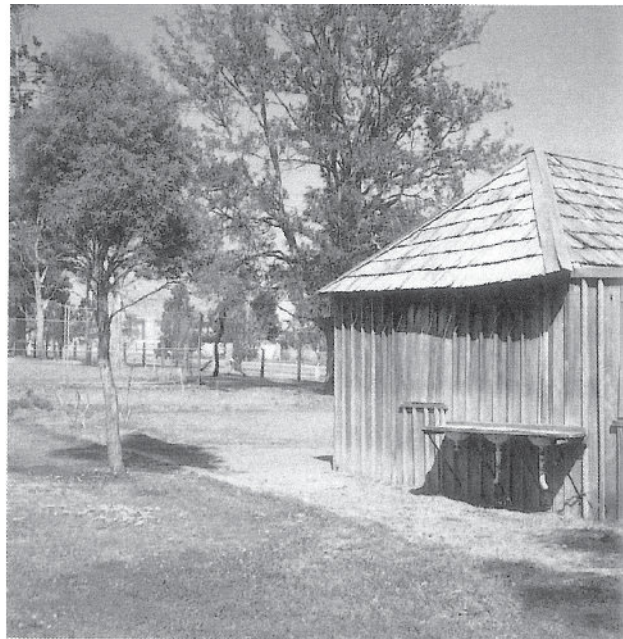
A roof of split timber shingles or 'shakes' on a small reconstructed pioneer schoolhouse.
