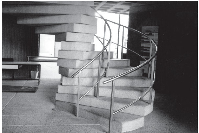
An unusual precast concrete stair with stainless steel balustrade.
