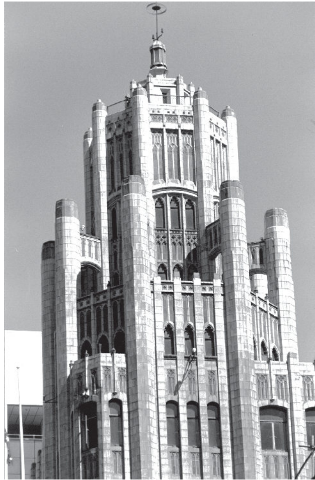
Finely detailed faience work executed about 1930. Now in a highly polluted atmosphere and showing deterioration.
