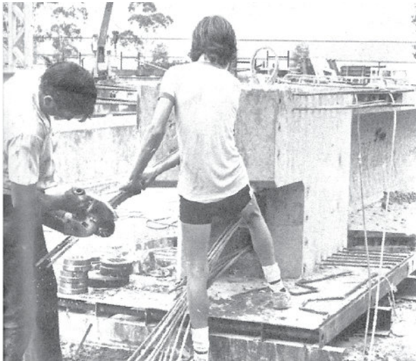
Preparing cables for tensioning.
