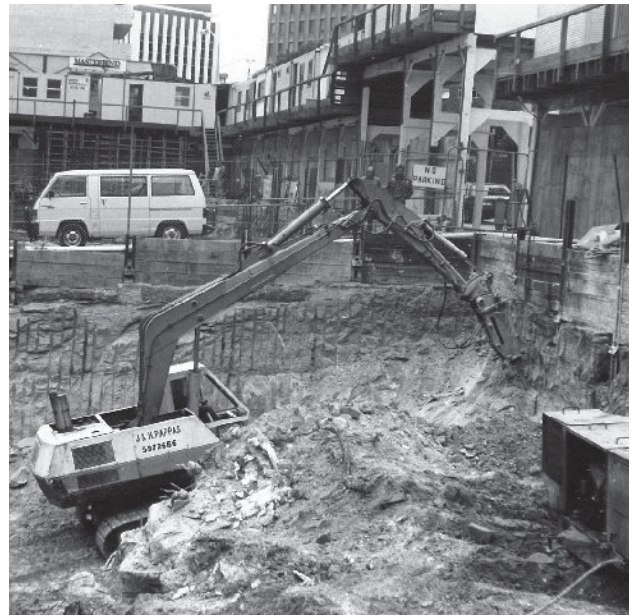
Heavy machinery excavating solid sandstone to a vertical face for a building basement.
