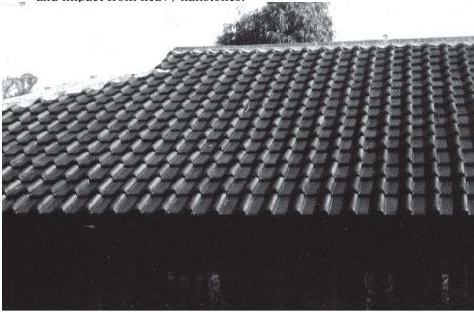
A terra cotta tiled roof using a dark manganese glaze.
