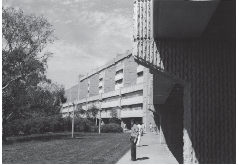
Heavily textured in situ concrete columns contrasting with smooth 'C-shaped precast beams.
