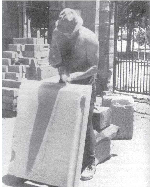
Traditional handworking of sandstone for restoration work.
