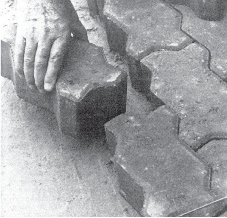
Interlocking paving blocks being laid. Many patterns are available.
