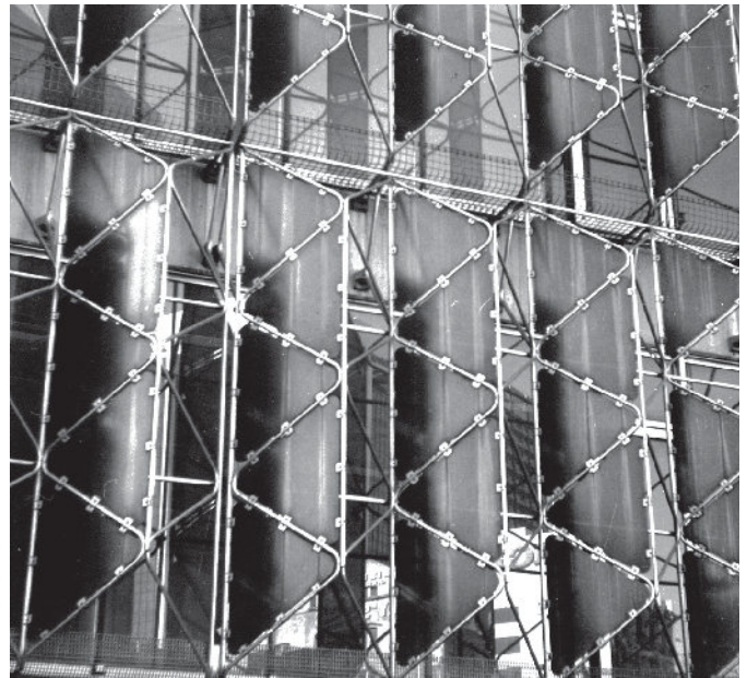
Polycarbonate sheets attached to stainless steel tubing to form sunscreens.
