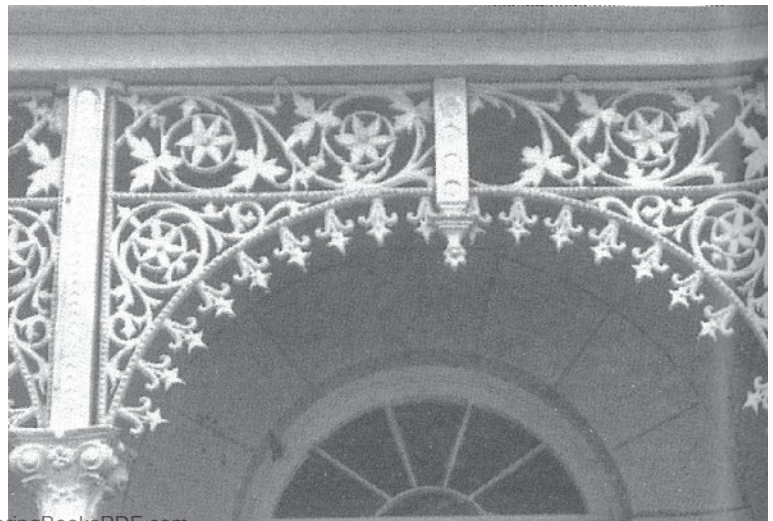
Cast iron verandah posts and lacework typical of late Victorian details.
