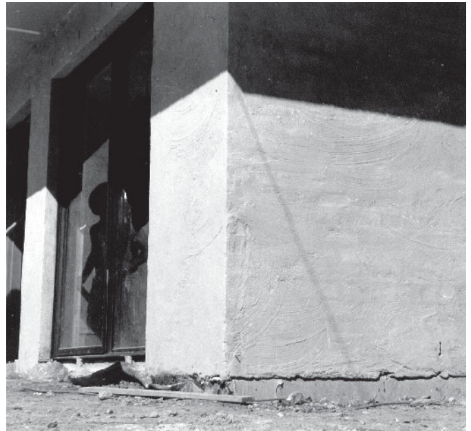
A light cement render coat such as this is not thick enough for a smooth finish but provides a pleasing texture or base for further finishes.
