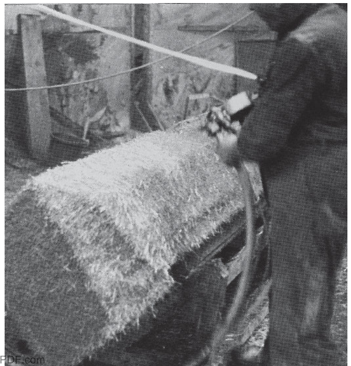
Cem FIL chopped fibres, cement and sand being applied by a gun process to produce GRC over a mould. Note the hairy nature of the surface produced on the gun side.
