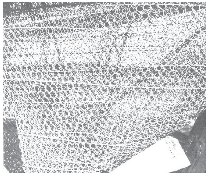
Galvanised wire mesh reinforcement ready to take the cement mortar to form a yacht keel of ferro cemento.
