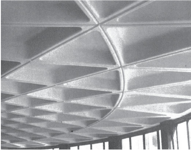
Complex and decorative ribbed ceiling achieved by use of ferro cement moulds as permanent formwork.
