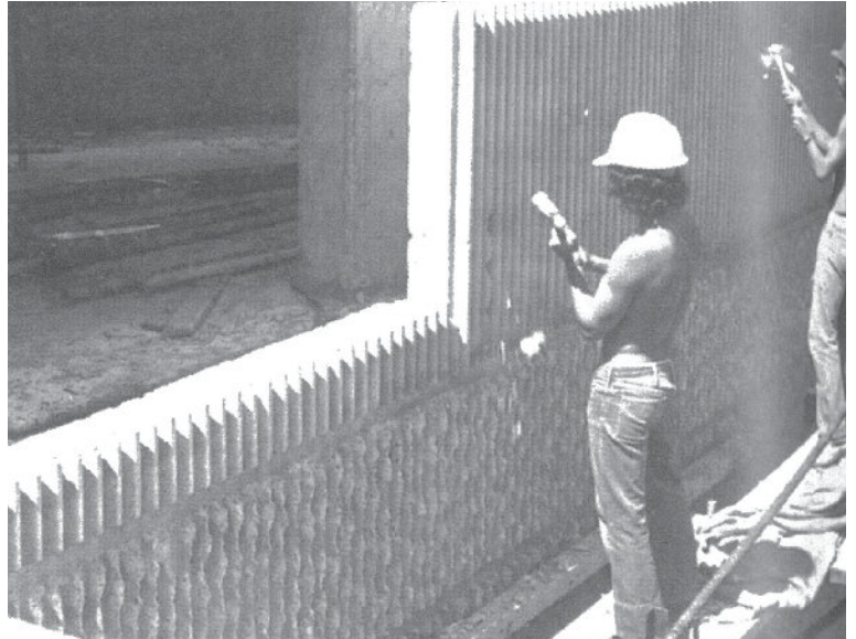
Method of achieving heavy texture by hand hammering finely ribbed concrete.
