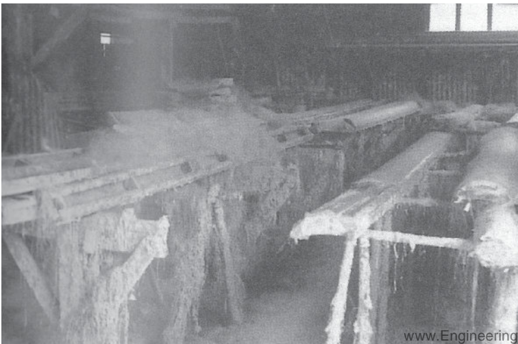
Casting benches for fibrous plaster cornices.
