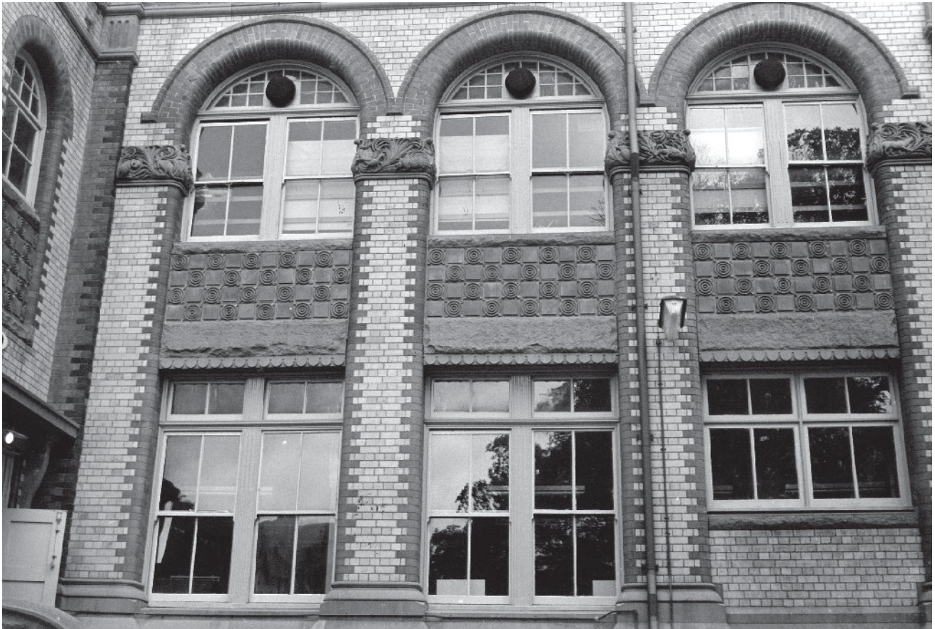
Late 19th-century decorative masonry walling incorporating contrasting coloured and moulded bricks, sandstone and terra cotta panels.
