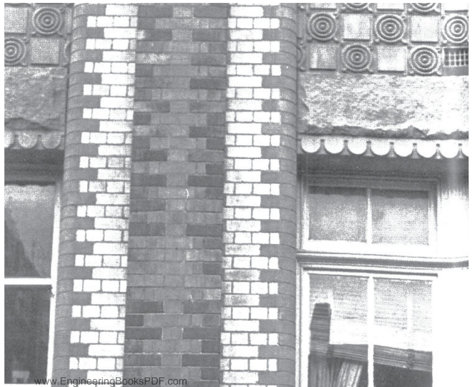
A 19th-century building showing the compatibility of brick, stone and ceramics as masonry materials.
