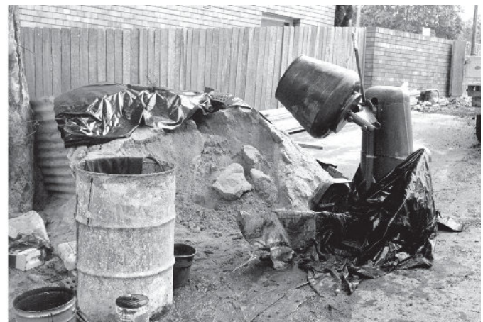
Sand heap and equipment for mortar and plaster mixing on a building site.
