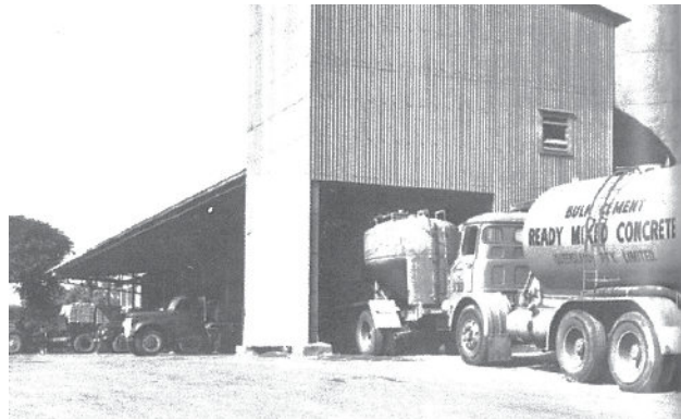
Trucks loading bulk and bagged cement at factory. Note also the corrugated asbestos cement cladding to walling.
