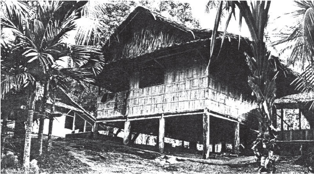
Elevated floor framing using round timbers. Wall covering uses split bamboo sheathing.
