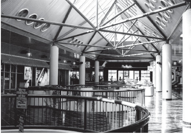
Steel pipes used as structural components. Balustrades incorporate lightweight pipes and steel rods welded together.
