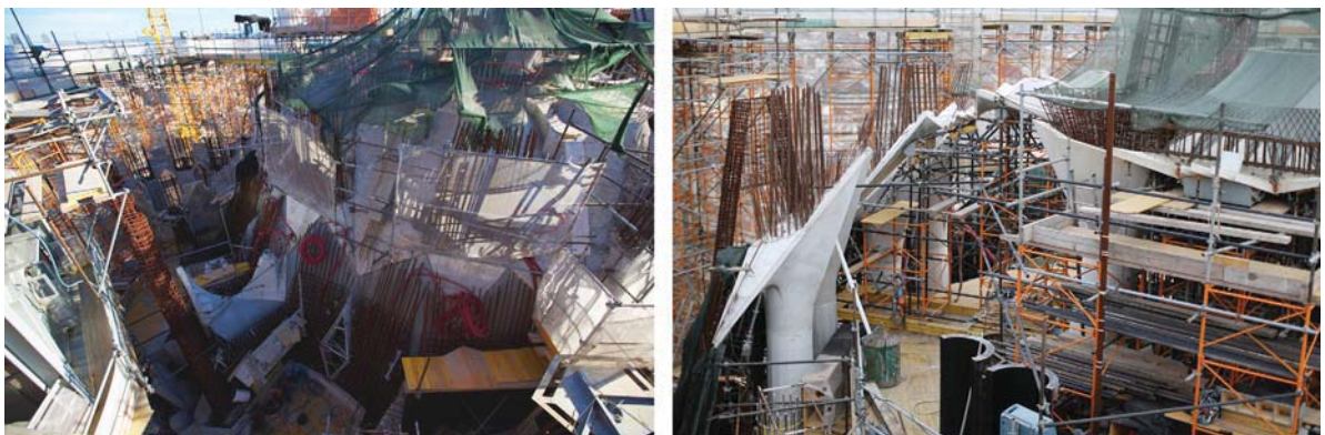
FIGURE 26.13 Looking down toward the nave roof construction (left); column capitals joining the perimeter of the ceiling vaults within (right).
