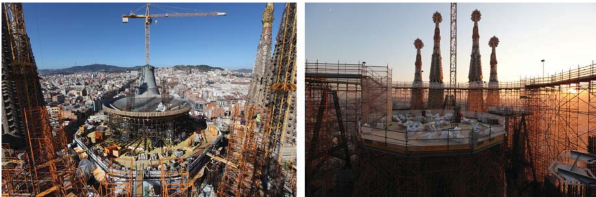
FIGURE 26.10 The formwork for the Sala Creuer auditorium seen from the crane (left); platform used to marshal the precast and cut stone elements (right).
