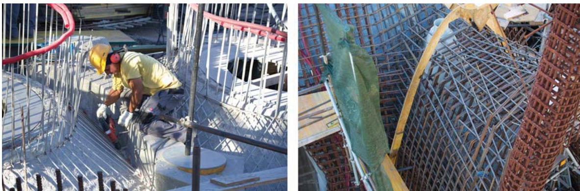
FIGURE 26.15 Exterior view of completing the vaults. Note the reinforcement exactly follows the straight-line rulings of the constituent hyperboloid of revolution geometries (left). Each rebar is drawn in 3D in Rhino (right).
