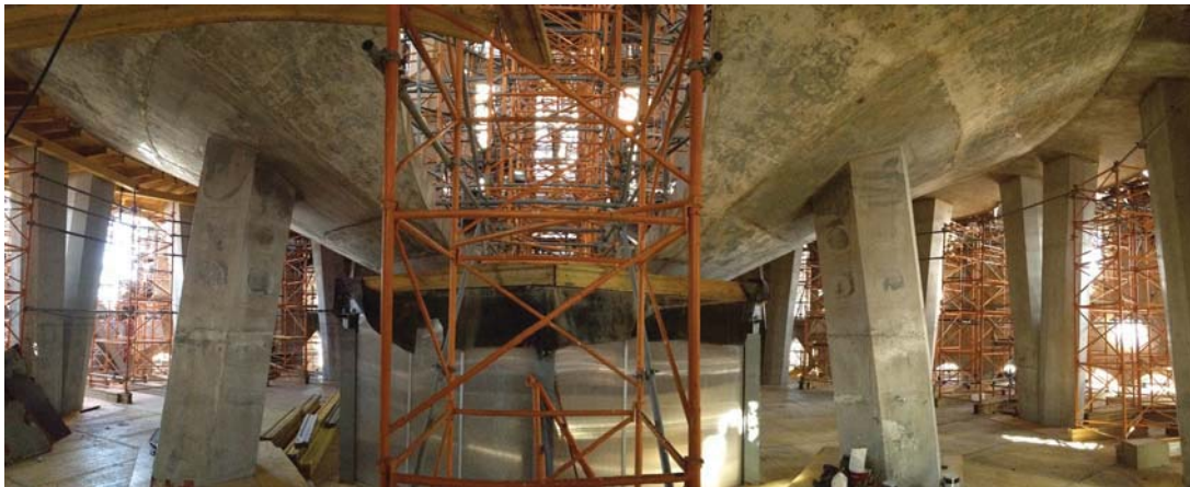
FIGURE 26.14 Undercroft of the auditorium.
