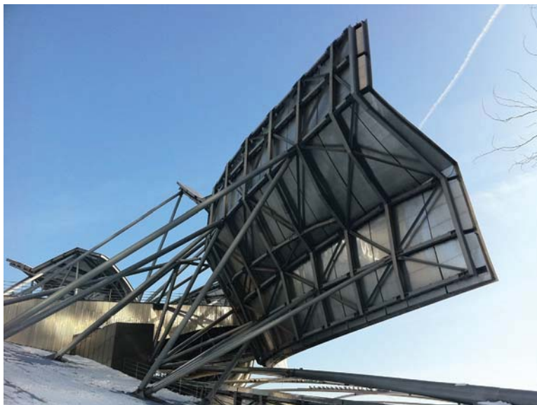
FIGURE 16.5 Pritzker Pavilion, Chicago, Illinois, 2004.
