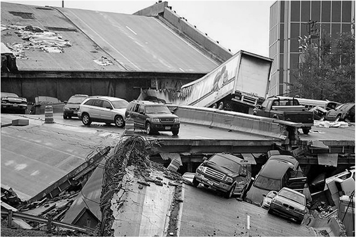
Figure 8.4 I-35 Bridge collapse, Minneapolis, Minnesota. (Photo by U.S. Coast Guard.)
