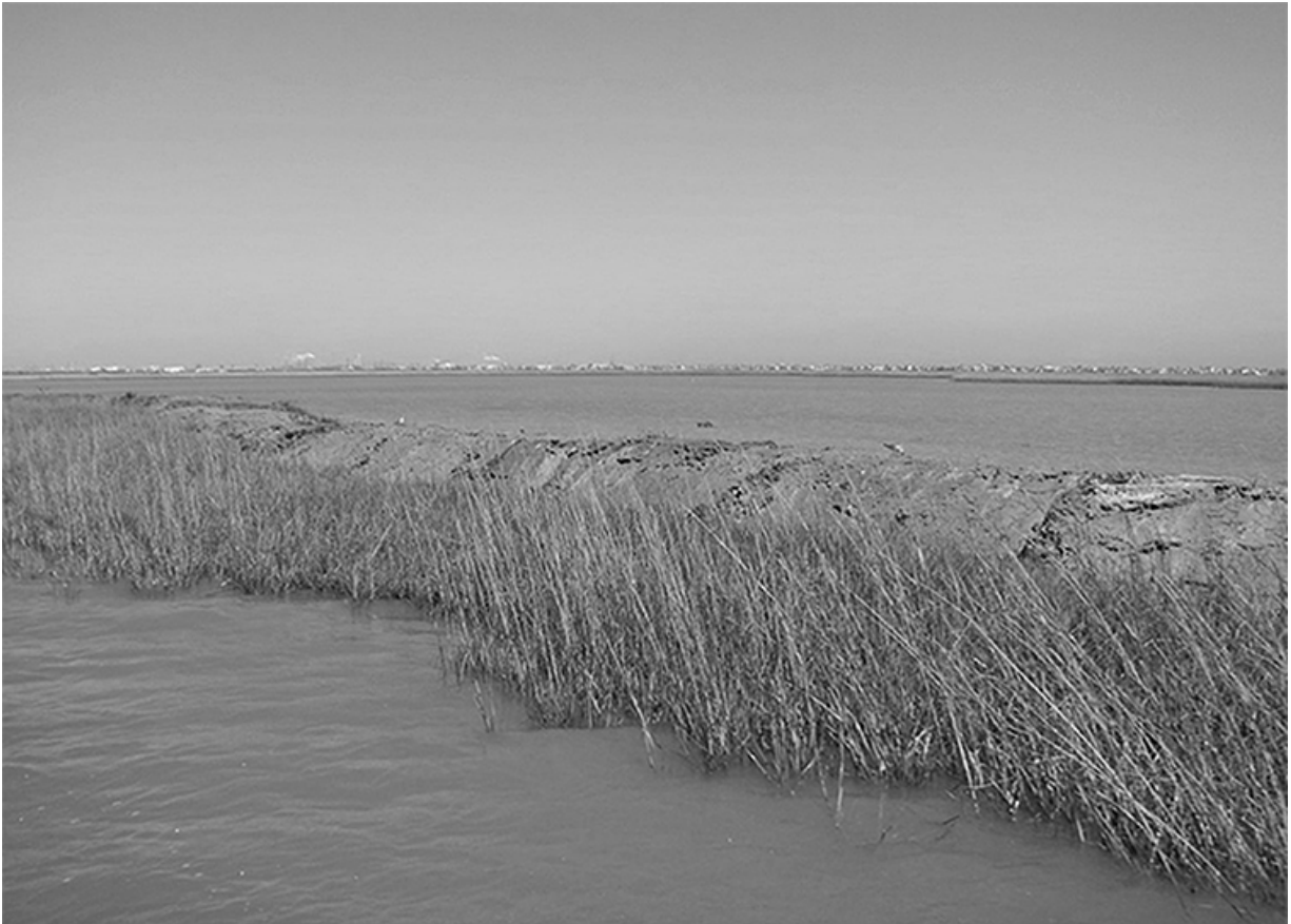
Figure 9.9 A small levee constructed in Pierce Marsh in Hitchcock, Texas. (Photo by National Oceanic and Atmospheric Administration.)
