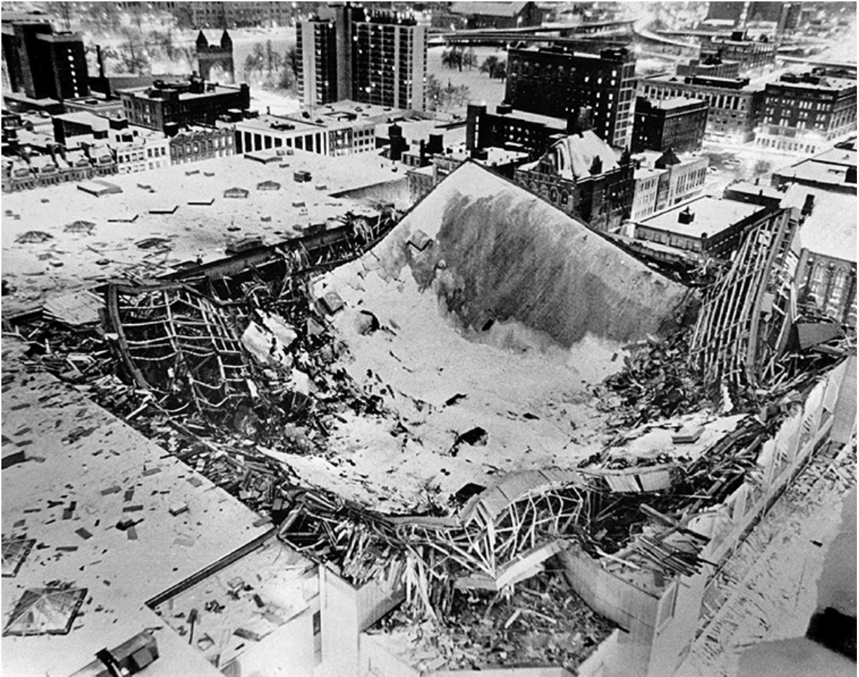
Figure 8.3 Hartford Civic Center Stadium in Hartford, Connecticut, after the roof collapsed on January 18th, 1978. (Photo courtesy of the Connecticut Historical Society.)
