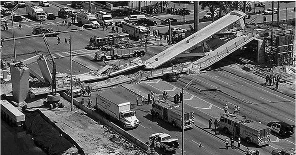
Figure 8.5 Eighth Street pedestrian bridge collapse, Miami, Florida. (Image from U.S. Department of Labor/OSHA Report prepared by Mohammad Ayub, July 2019.)
