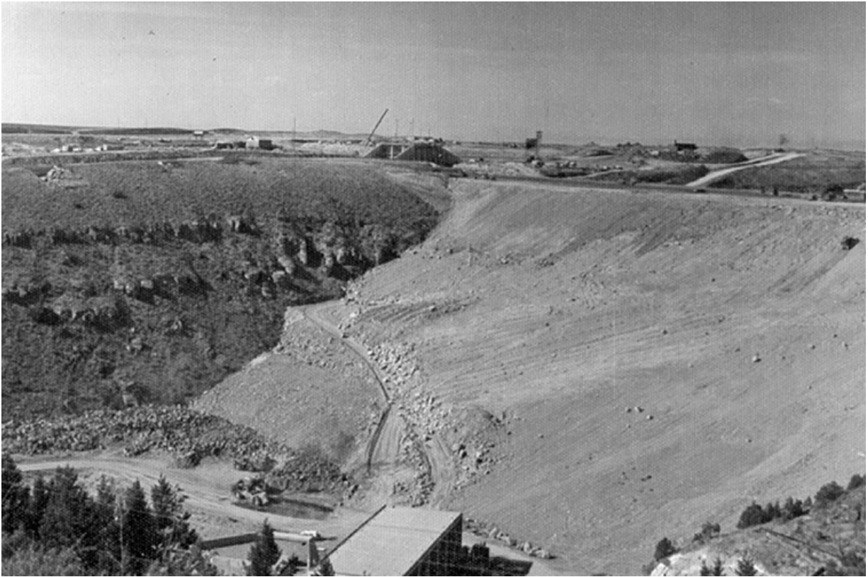
Figure 8.2 Downstream view during construction of the Teton Dam, Newdale, Idaho. (Image from “Lessons Learned from Dam Incidents and Failures,” Association of State Dam Safety Officials.)
