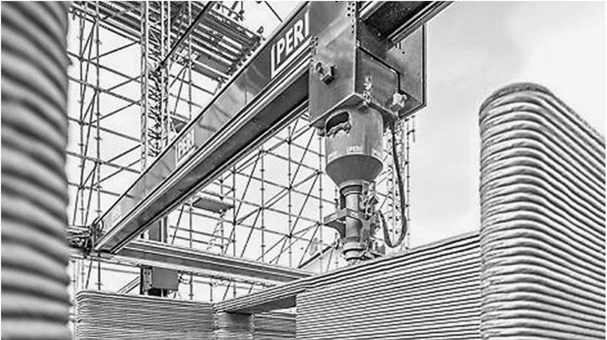
Figure 9.10 A 3D concrete printed residential building in Beckum, North Rhine-Westphalia, Germany. (Image by PERI GMBH.)
