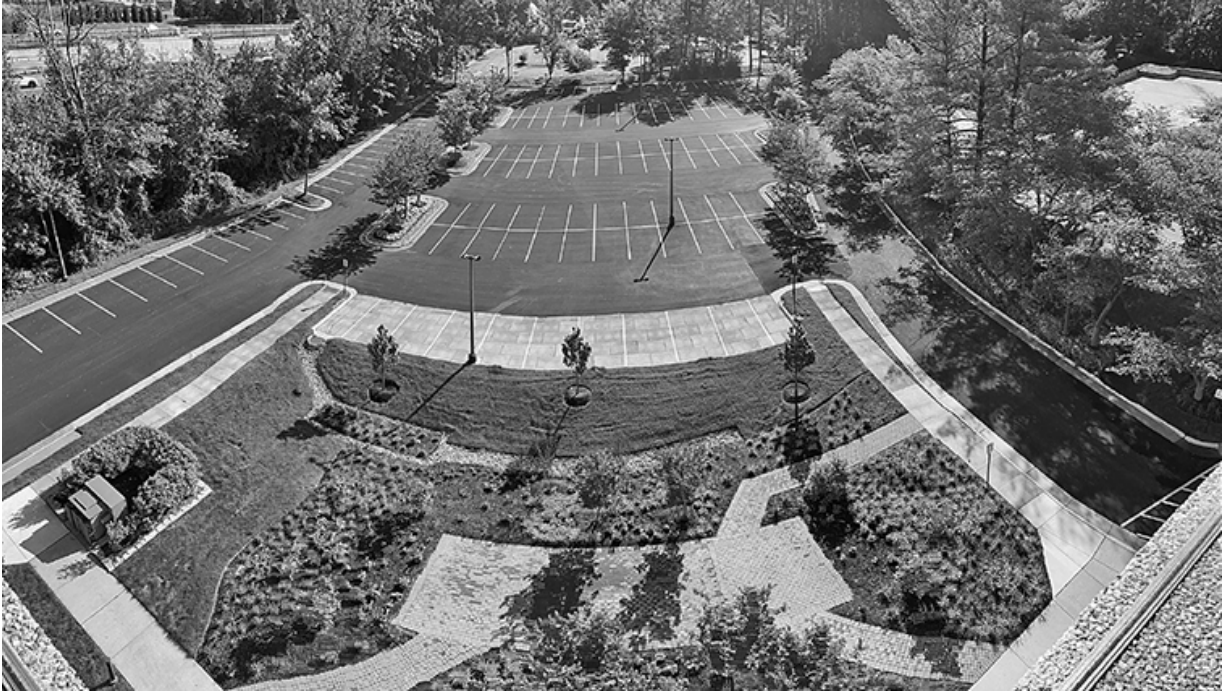
Figure 9.8 Courtyard area in the parking lot at ASCE headquarters in Reston, Virginia, with precast porous concrete panels and a biofilter for storm water treatment. (Courtesy ASCE Foundation.)
