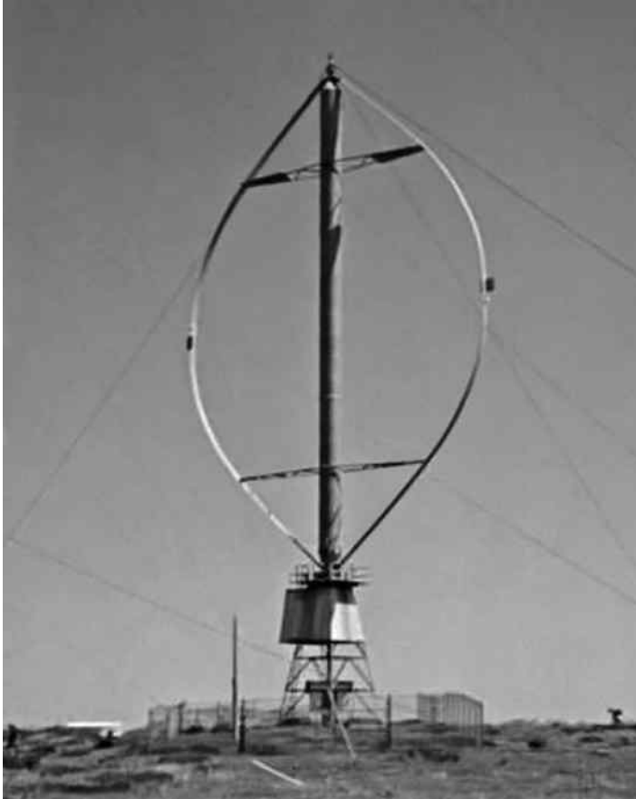
Figure 2.3 (See color insert.) Vertical axis wind turbine.
