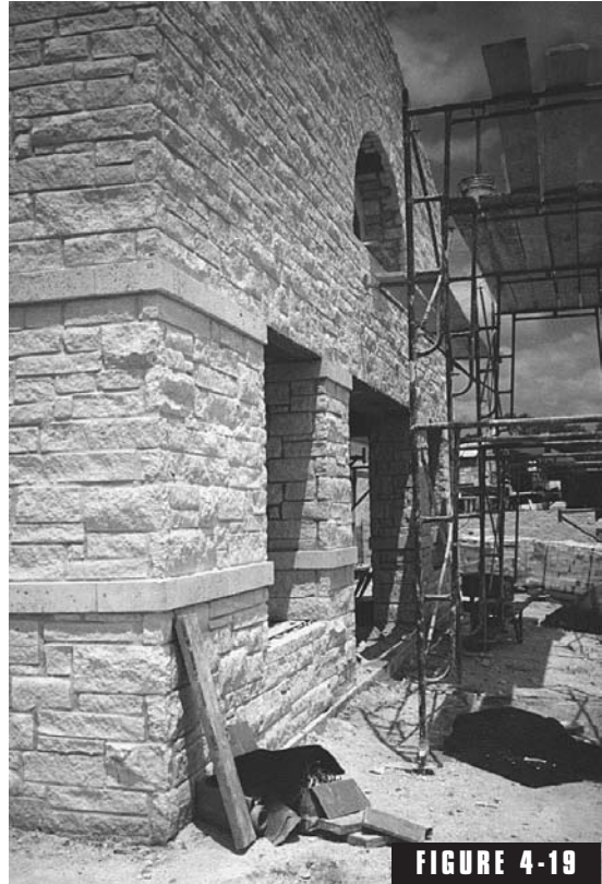
Rubble stone and ashlar used together.
