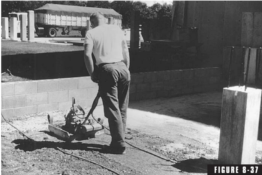
Vibrating plate compactor.
