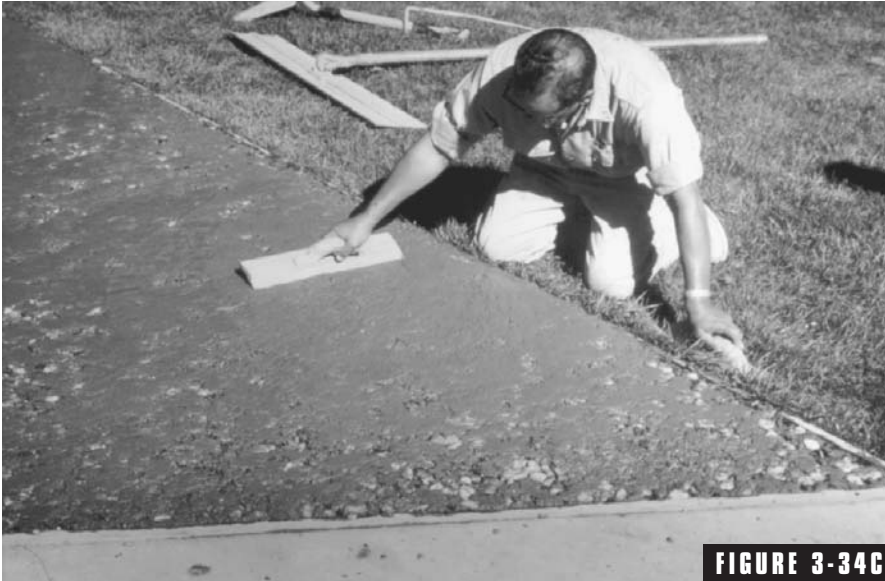
Embedding aggregate for exposed aggregate finish. (Photo courtesy PCA).
