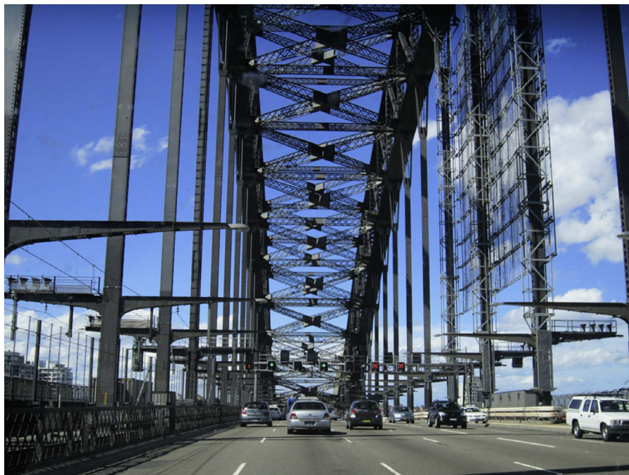
FIGURE 3.2 The deck hangers of the Sydney Harbour Bridge. Note the scaffolding on the right hand side, ready for carrying the fireworks for the world famous New Year's Eve firework display. -35\ 51\ 14.40\ S\ 151\ 12\ 51.66E
