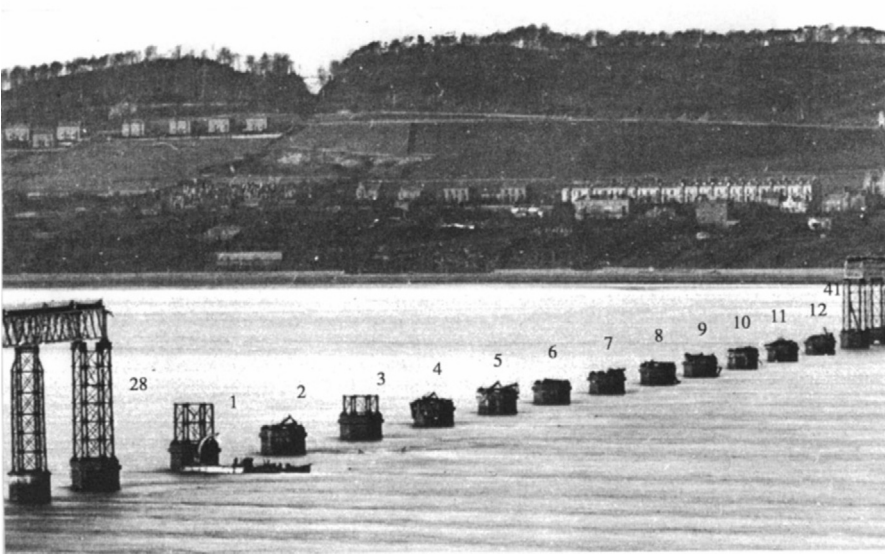
Fallen piers as seen from the south bank of the fiord. For the purposes of the investigation, the piers between 28 and 41 were renumbered 1 to 12. (Courtesy of University of St. Andrews.)
